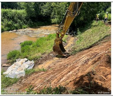
**Photo Description:** Topsoil was removed from the right bank and stockpiled.
