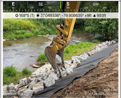
**Photo Description:** Class III rip rap was placed over geotextile fabric along the right bank.
