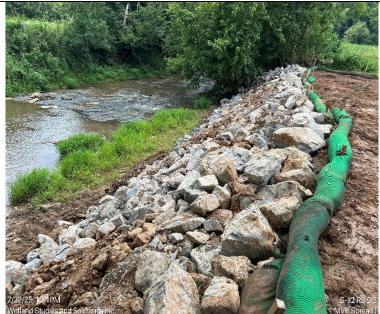
**Photo Description:** Overview of right bank after the repair.
