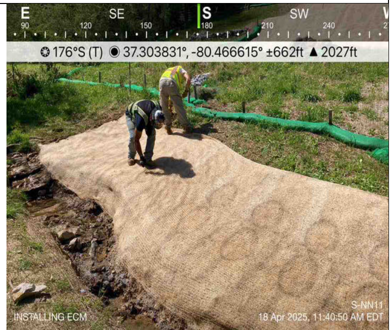
Photo Description: ECM was installed and properly keyed in.
