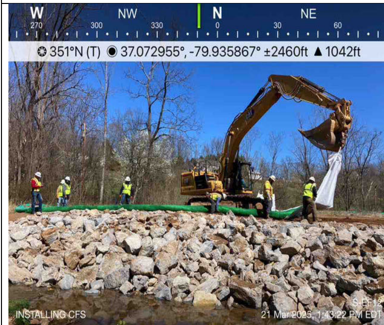
Photo Description: CFS installed around newly repaired stream bank.
