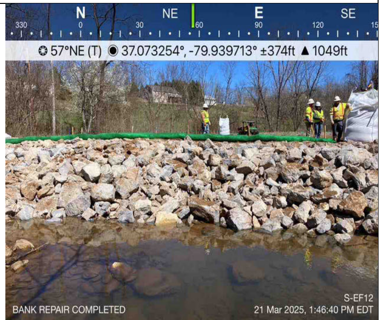
Photo Description: Stream bank repaired in full.
