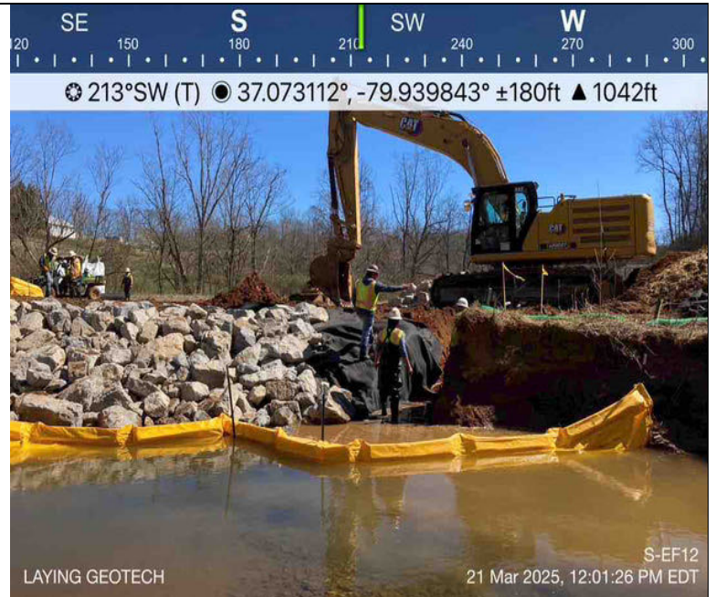
Photo Description: Geotech installed under class 3 riprap.
