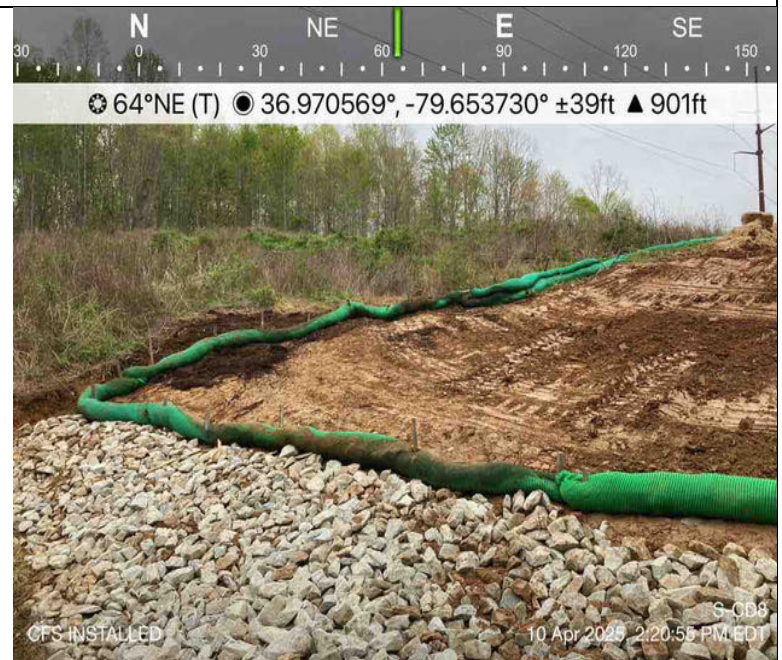
Photo Description: CFS installed along recently repaired banks.
