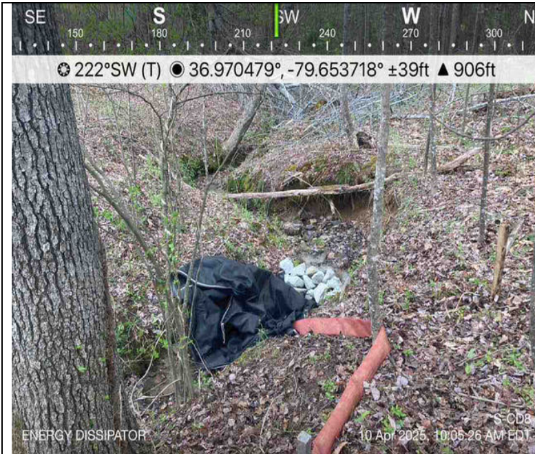
Photo Description: Energy dissipator installed downstream.
