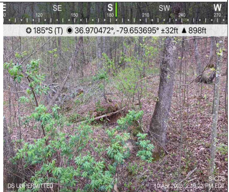
Photo Description: Conditions of the downstream area outside the ROW during post-construction assessment.
