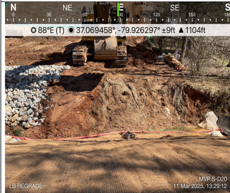
Photo Description: Regrading left bank where bridge was staged.
