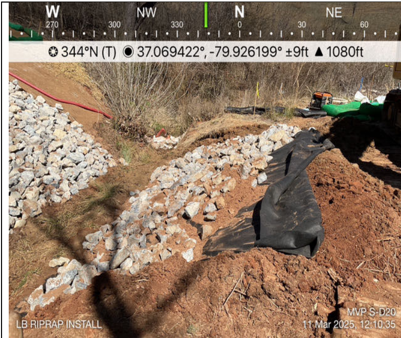
Photo Description: Riprap placement on left bank.
