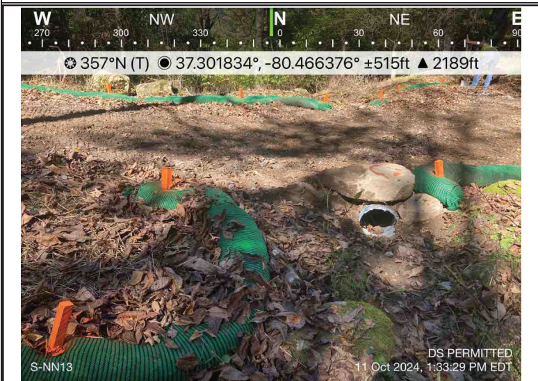
Photo Description: Downstream view of permitted impact area during post-construction assessment.
