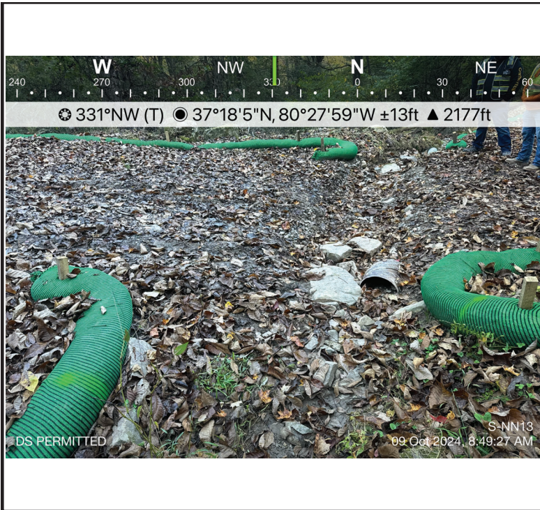
Photo Description: Downstream view of permitted impact area during pre-construction assessment.
