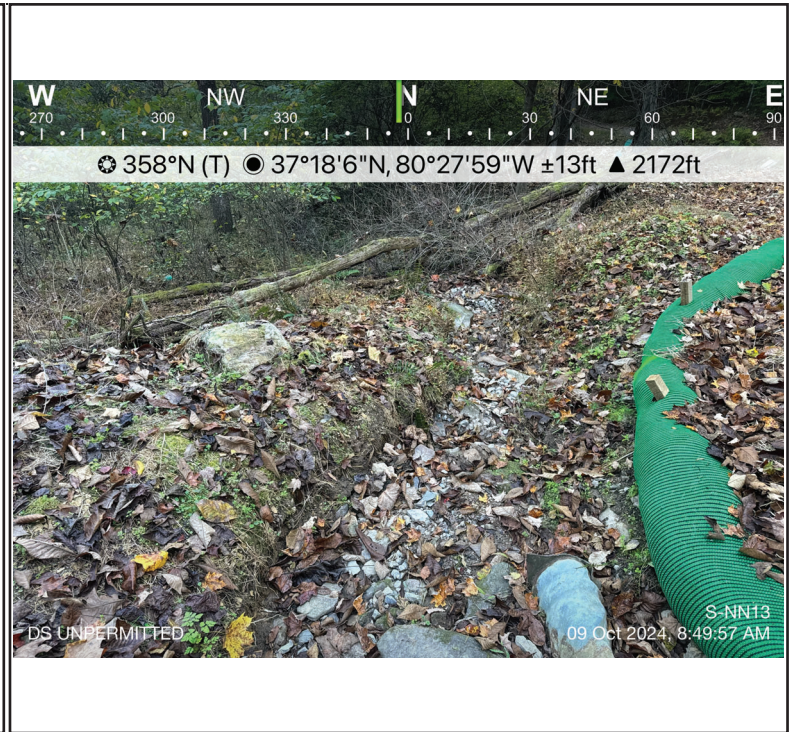
Photo Description: Downstream view of unpermitted area during pre-construction assessment.
