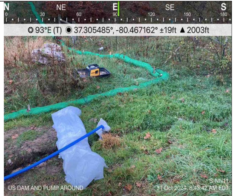
Photo Description: Dam and pump around installed.
