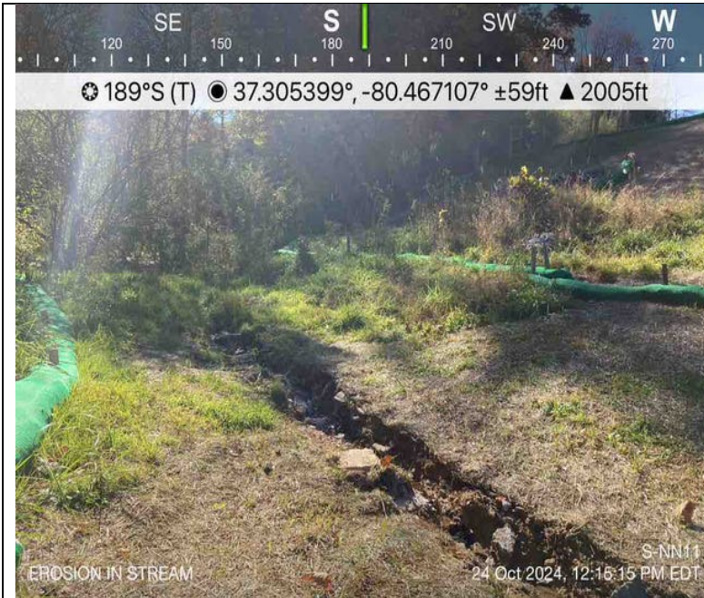
Photo Description: Erosion within the stream bed.
