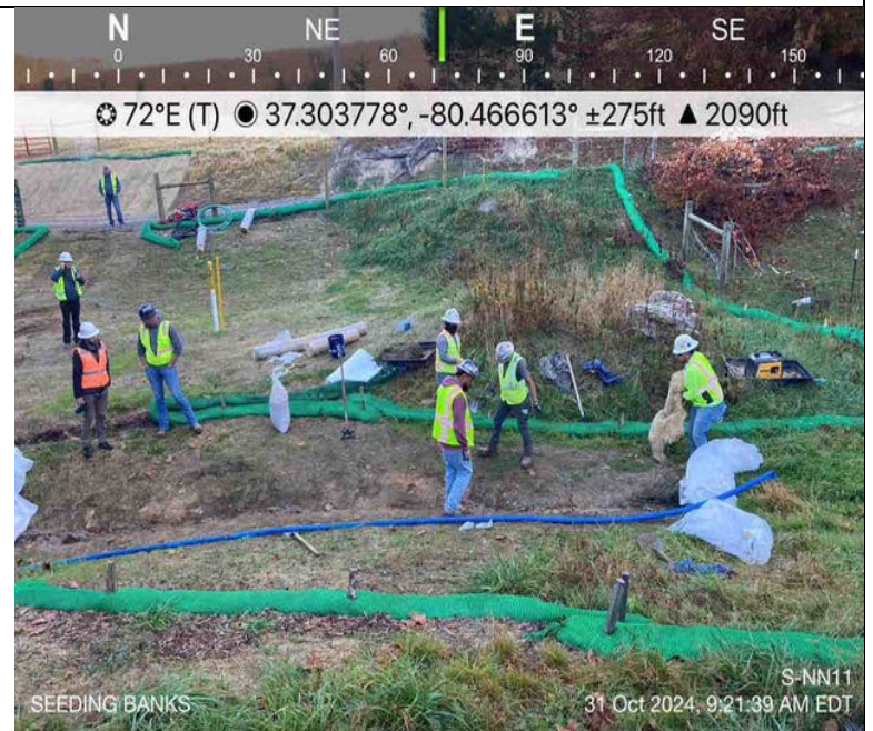
Photo Description: Applying seed to the banks before installing ECM.
