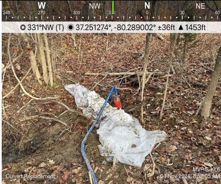
Photo Description: Dam and pump installation on upstream side of culvert.
