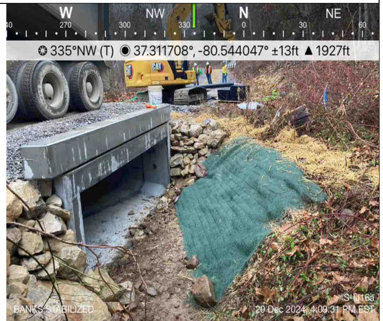
Photo Description: Banks were seeded and strayed and ECM installed.
