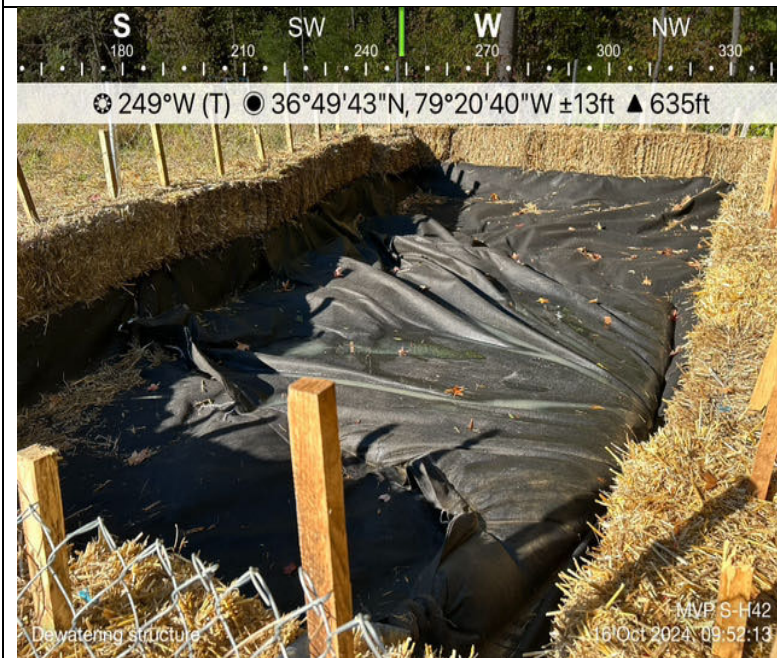
Photo Description: Dewatering structure onsite.
