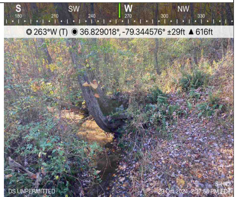
Photo Description: Conditions of the downstream area outside the ROW during post-construction assessment.
