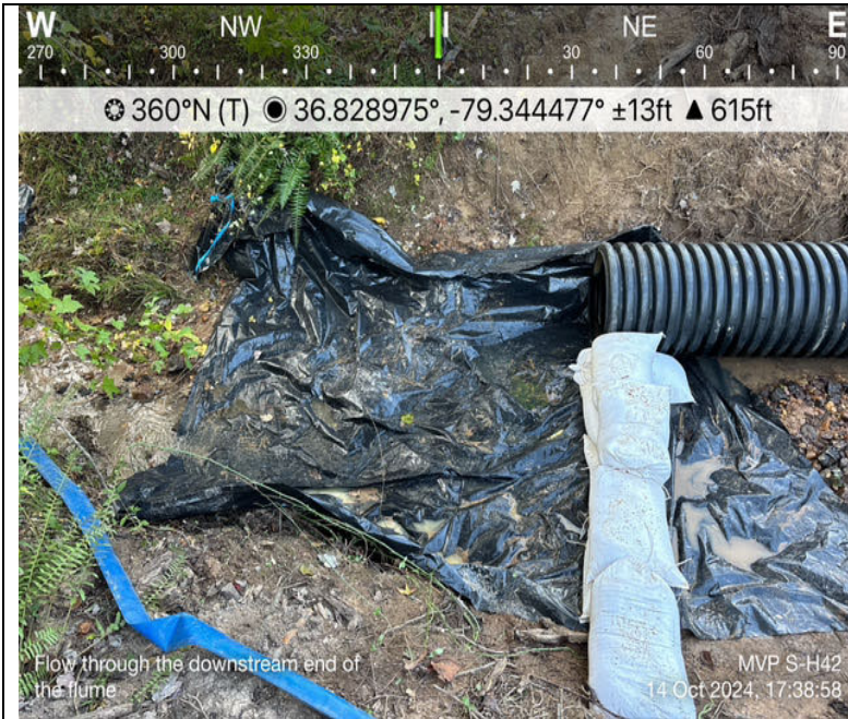
Photo Description: Flume installed to convey stream flow.
