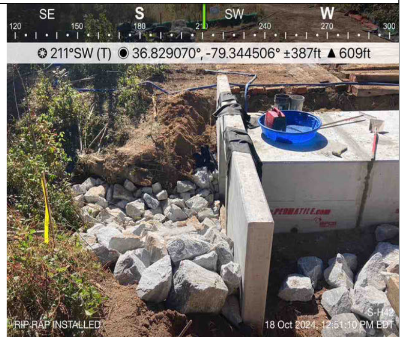
Photo Description: Riprap installed on inflow of culvert.
