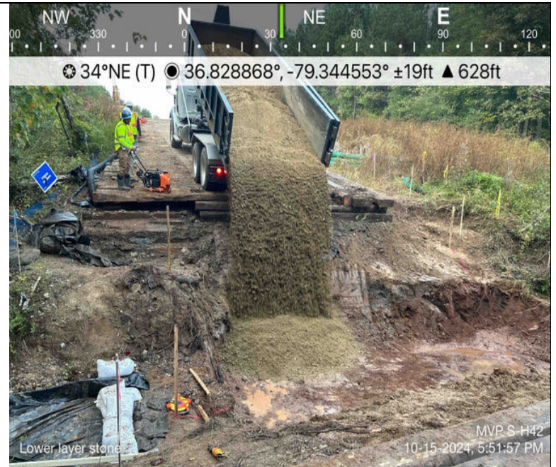
Photo Description: Bottom layer of stone installed.
