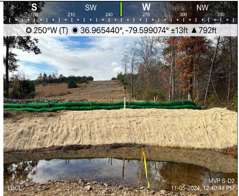
Photo Description: View of the regraded right bank from standing on the left bank.
