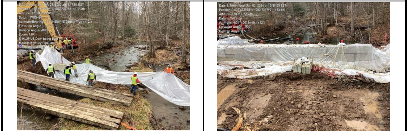
GPS Location See Photo GPS Location See Photo Description Photo 1: Constructing upstream dam. Description Photo 2: Top 12 inches of substrate removed from aquatic resource.
