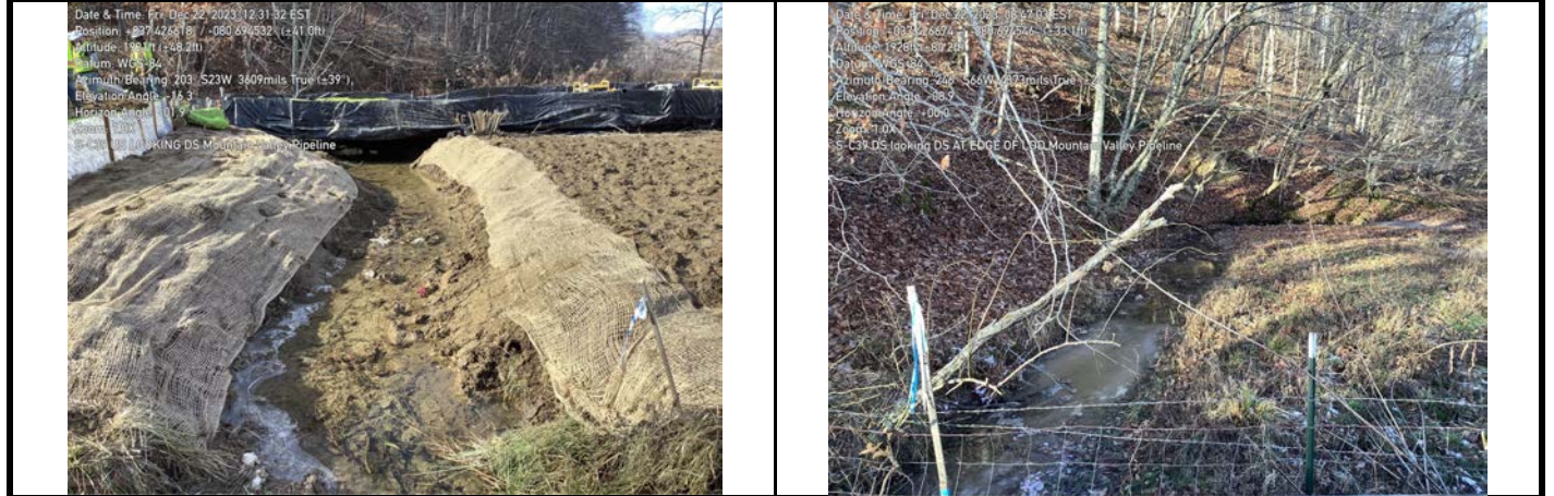
GPS Location See photo GPS Location See photo Description Downstream view of permitted impact area during post-construction assessment. Description Downstream view of unimpacted area during post-construction assessment.
