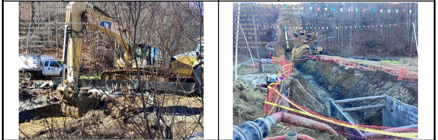
GPS Location See photo GPS Location See photo Description Photo 1: Excavating of first 12 inches of substrate. Description Photo 2: Excavated through aquatic resource.
