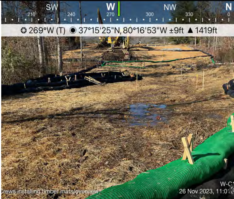
Photo Description: Crews laid timber mats to work in the wetland.
