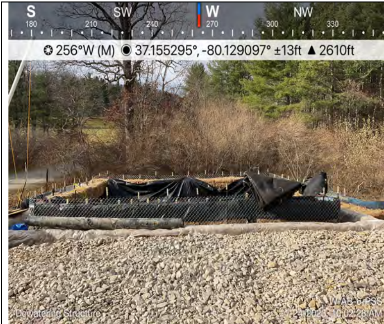
Photo Description: Second dewatering structure installed on site.
