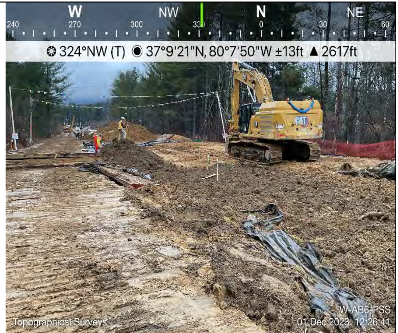
Photo Description: Survey team on-site providing pre-construction data for restoration.
