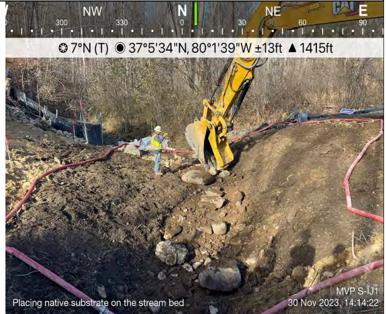
Photo Description: The crew replacing the native substrate into the stream bed.
