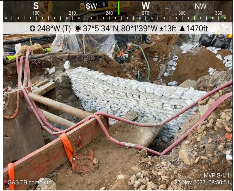
Photo Description: The trench breaker installed on the GAS.
