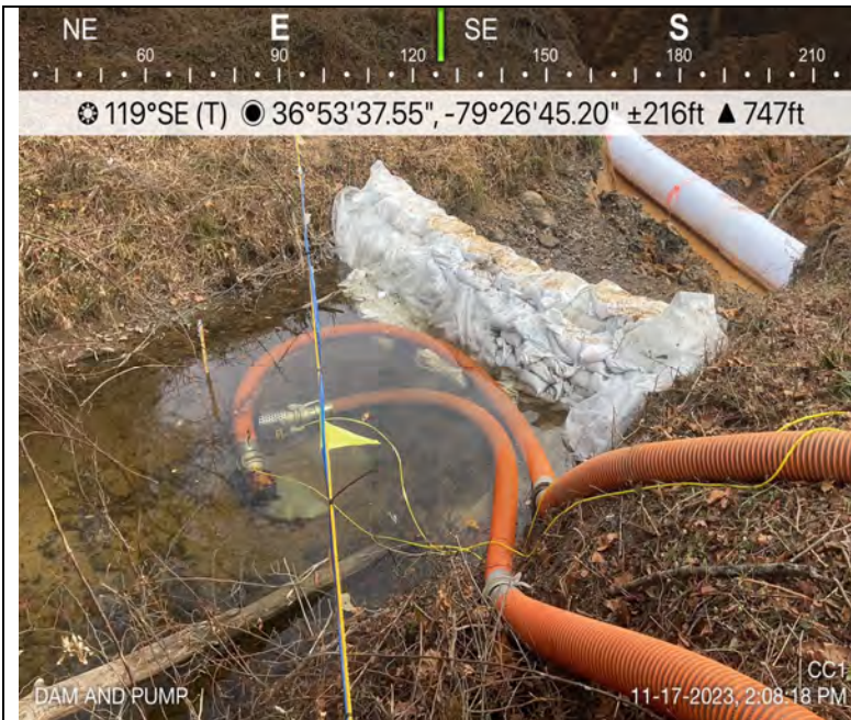
Photo Description: The dam and pump installed and functioning.
