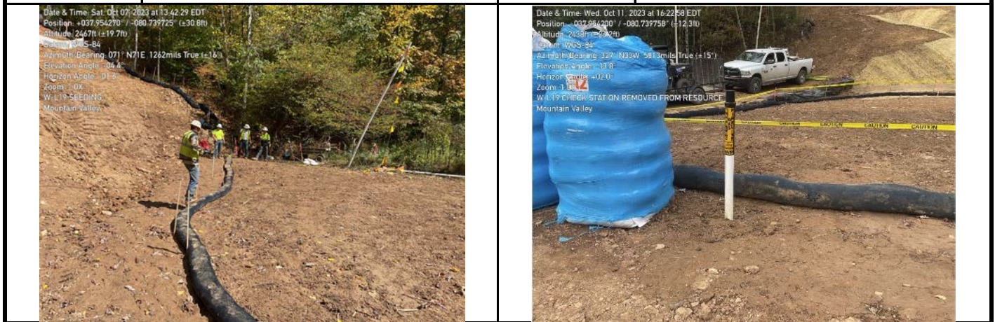
GPS Location See Photo GPS Location See Photo Description Photo 7: Seeding aquatic resources. Description Photo 8: Test station after removal from wetland (now outside of resource).
