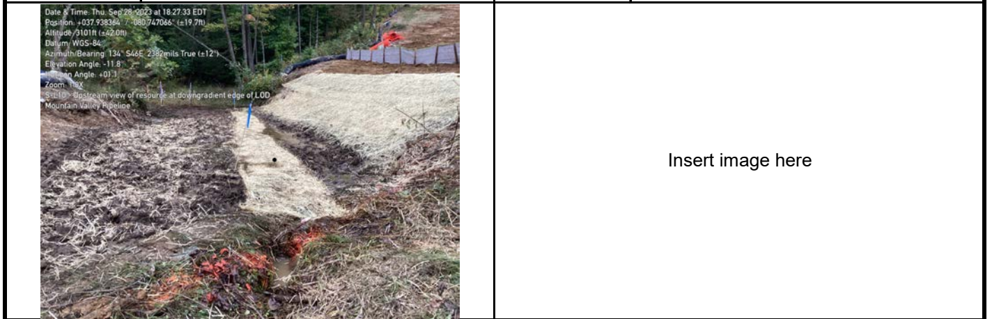
GPS Location See Photo GPS Location Description Photo 7: Curlex installed on bank. Description
