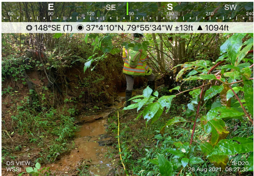
Downstream view within the ROW. Assessment is limited to areas within the temporary ROW.
