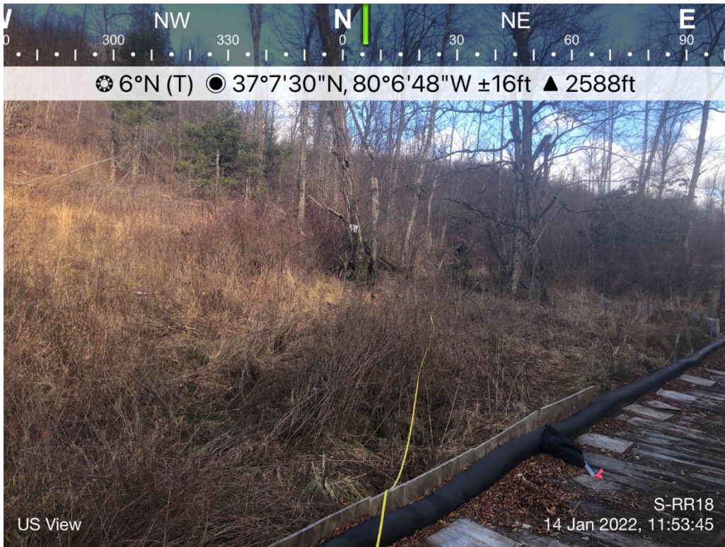
Photo Type: US VIEW Location, Orientation, Photographer Initials: Upstream view of LOC looking N, KB
