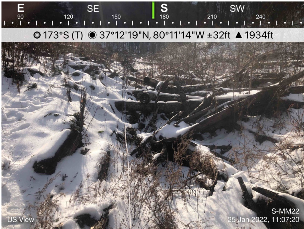
Photo Type: US VIEW Location, Orientation, Photographer Initials: Upstream view of LOC looking S, KB
