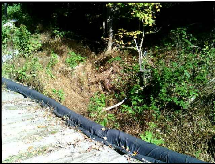
PHOTO TAKEN OCTOBER 15, 2021 LOOKING UPSTREAM FROM DOWNSTREAM IMPACT LIMITS
