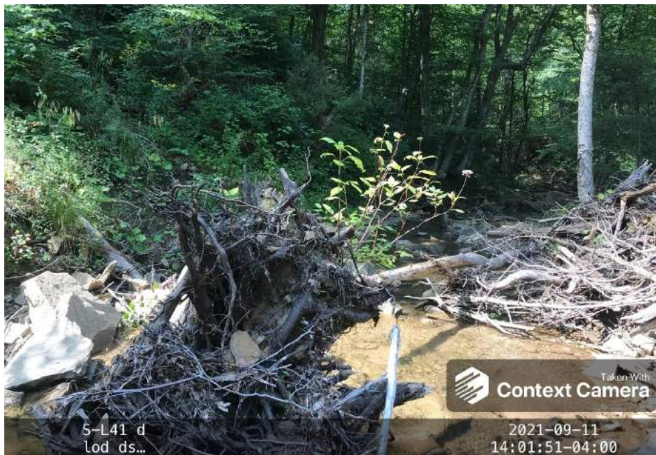
Photo Type: DS, DS View Location, Orientation, Photographer Initials: Downstream Edge of ROW, Downstream View, JD/AR Lat: 38.220793 Long: -80.7171
