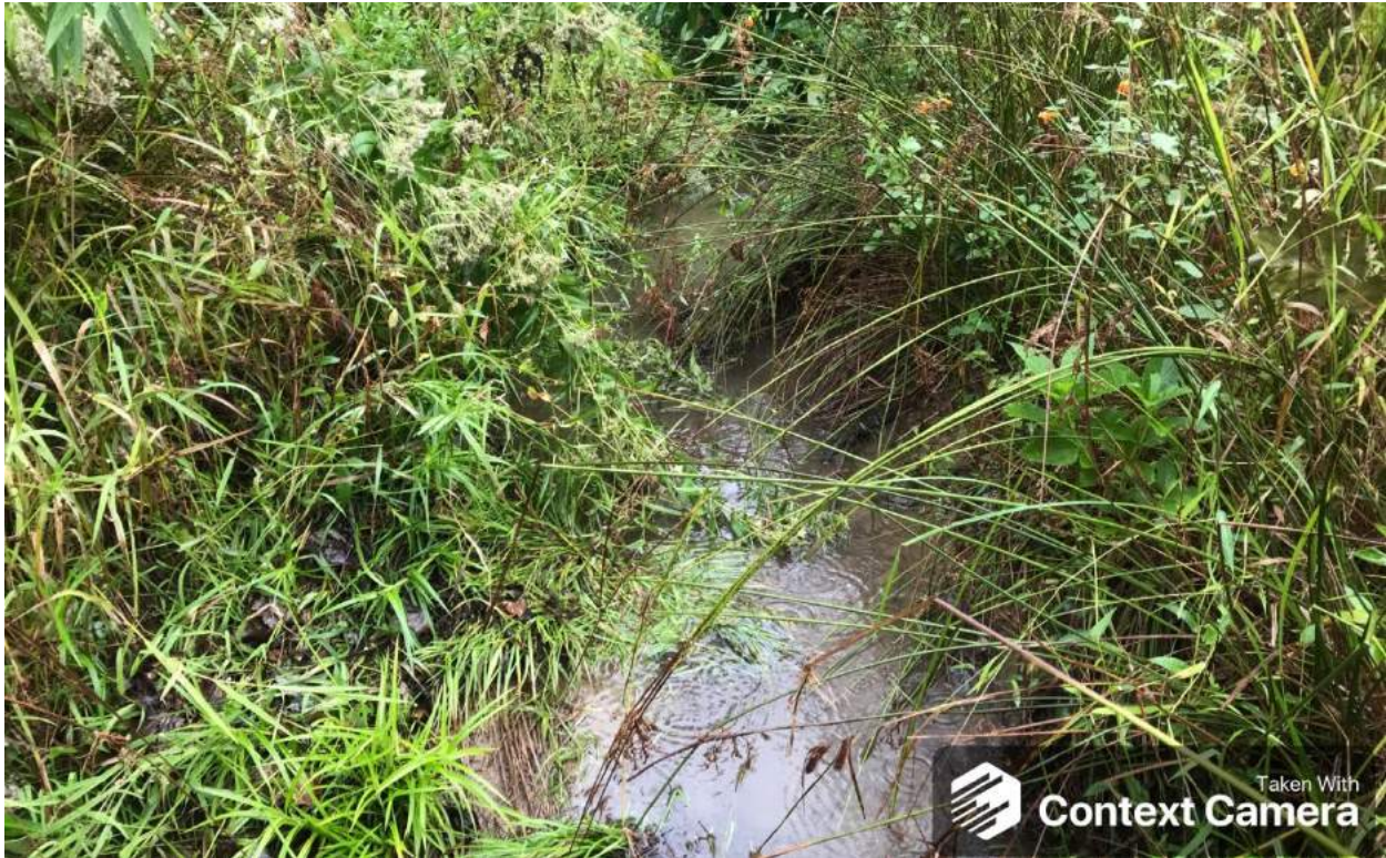
Photo Type: US View at Center Location, Orientation, Photographer Initials: Center ROW, Upstream View, AE PL Lat: 38.766123 Long: -80.520308
