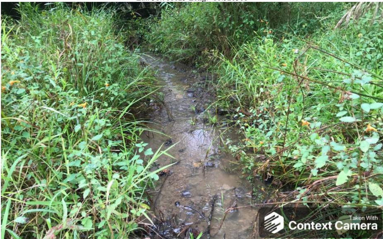
Photo Type: DS, DS View Location, Orientation, Photographer Initials: Downstream Edge of ROW, Downstream View, AE PL Lat: 38.766123 Long: -80.520308
