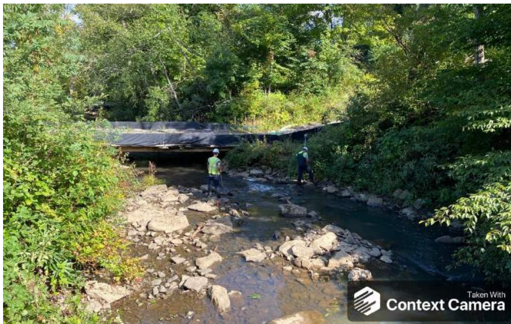
Photo Type: DS, DS View Location, Orientation, Photographer Initials: Downstream Edge of ROW, Downstream View, RC/CC Lat: 38.363374 Long: -80.617277
