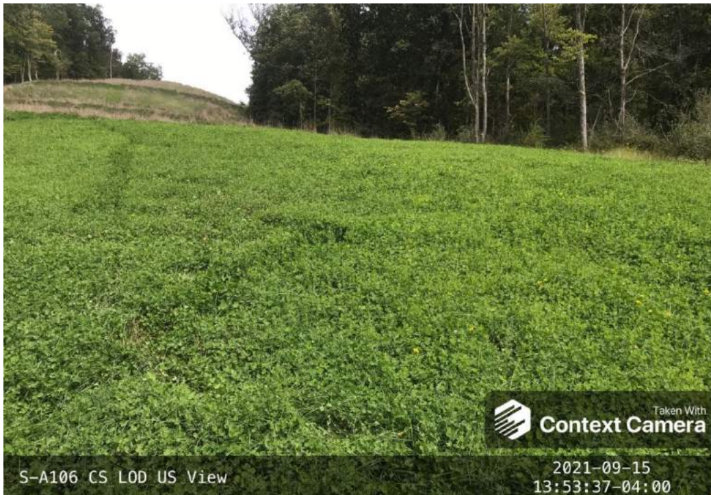
Photo Type: US View at Center Location, Orientation, Photographer Initials: Downstream Edge of ROW, Upstream View, Lat: 39.168435 Long: -80.577625
