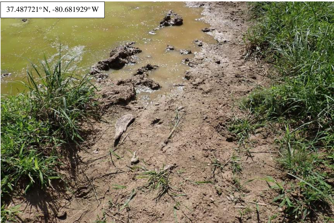
Photo Type: CP, DS View Location, Orientation, Photographer Initials: Center of Right of Way, Downstream View, AK/RA
