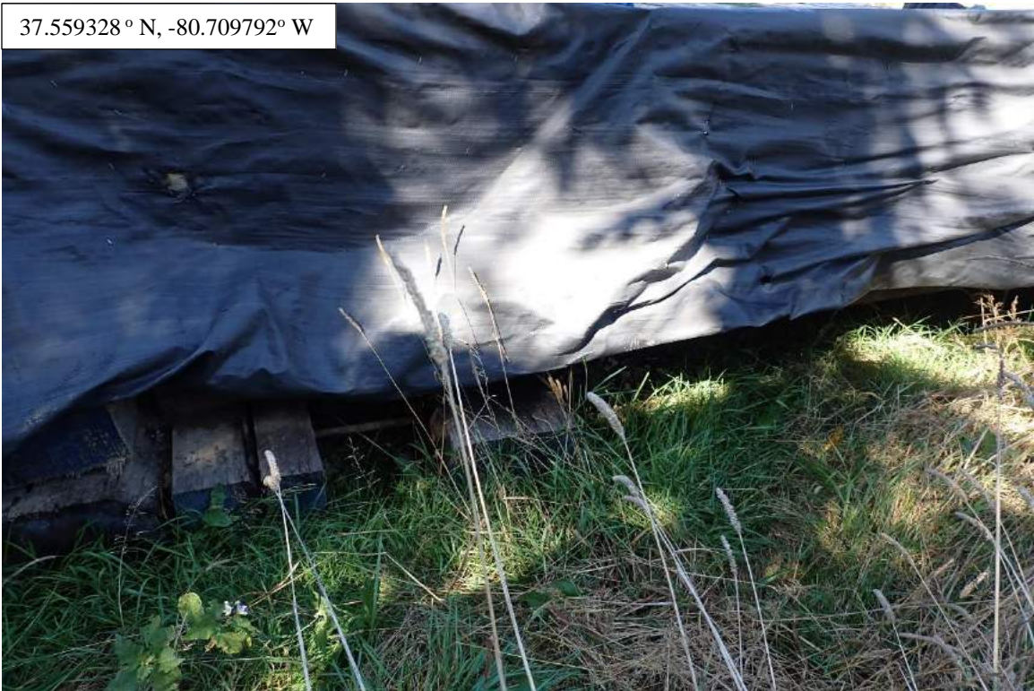
Photo Type: DS View Location, Orientation, Photographer Initials: Right of Way, Downstream View, AAK/SM/TA
