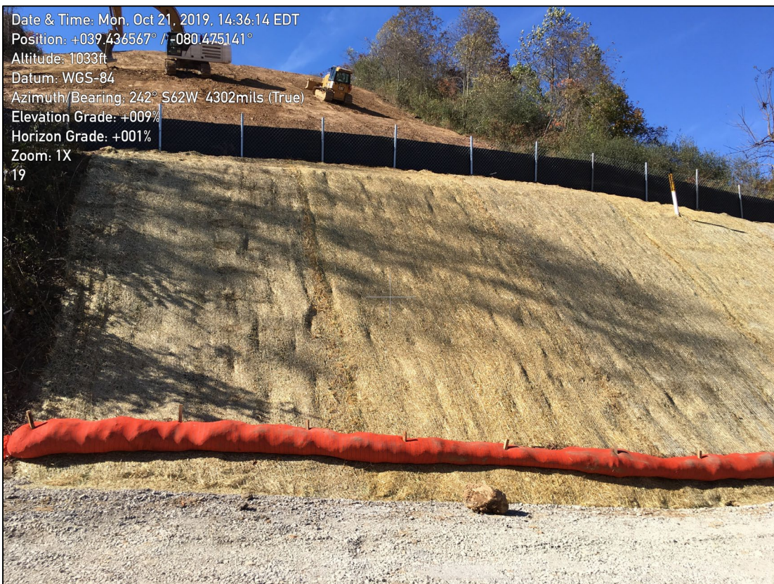
Photos 3 & 4: Photos illustrates the restoration near station 645+00. Erosion control blanketing and supersilt fence has been installed. The area upslope of the super silt fence is being prepared for restoration and stabilization.
