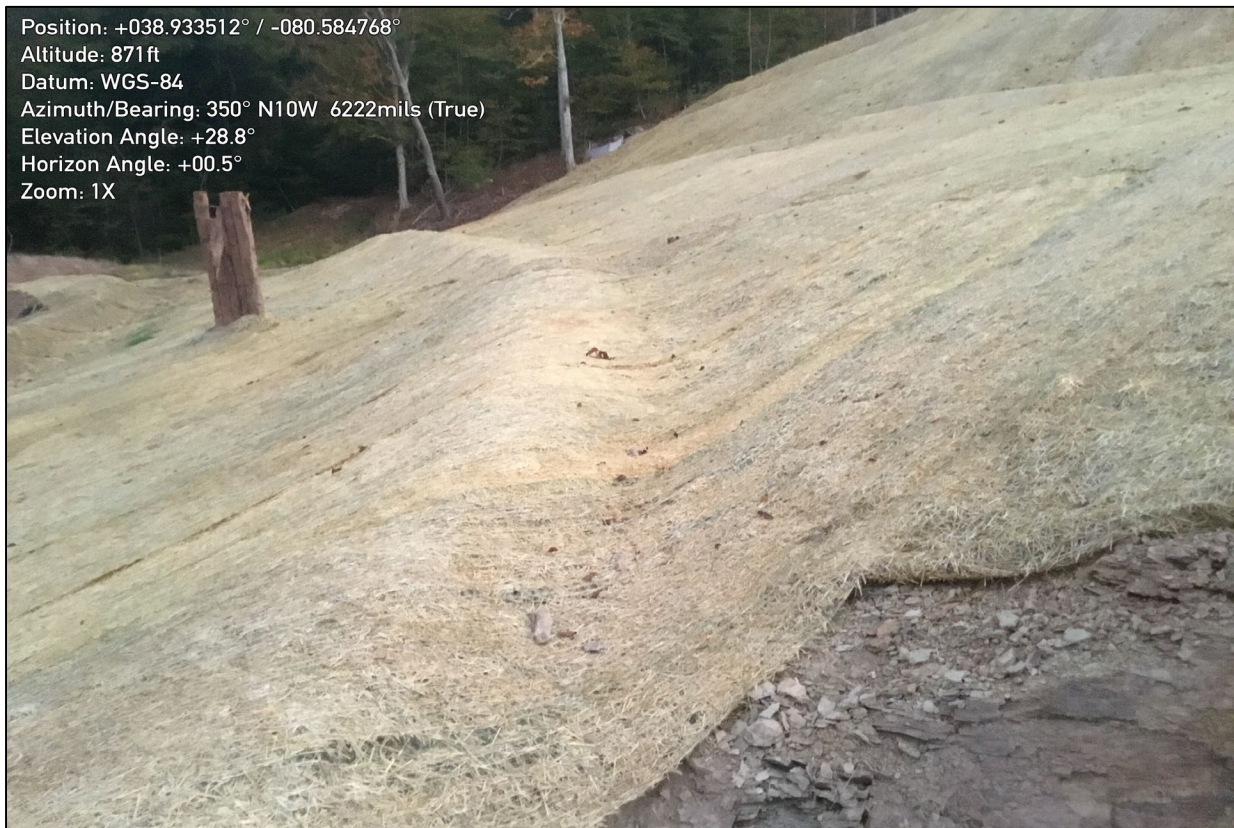
Photo 4: Photo illustrates the repaired waterbar and stabilized hillside, using ECB, located above CR 21.
