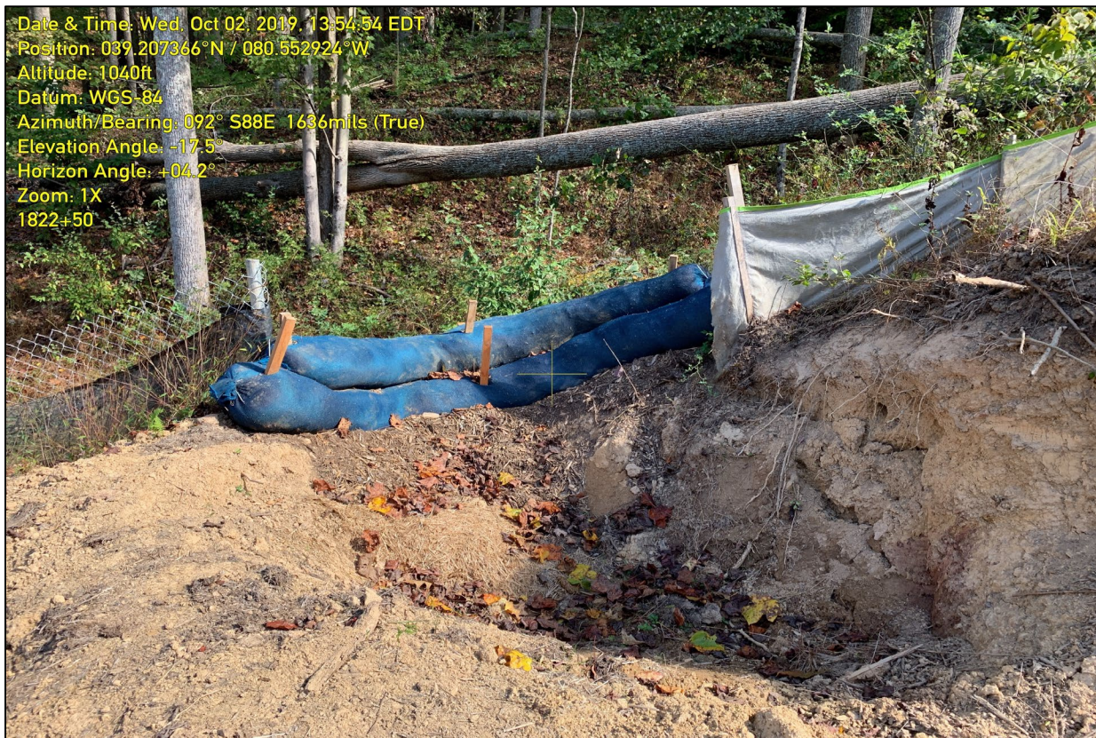
Photo 5: Photo illustrates repaired compost filter sock (CFS) that has been installed at the end of the waterbar in the inspection area.
