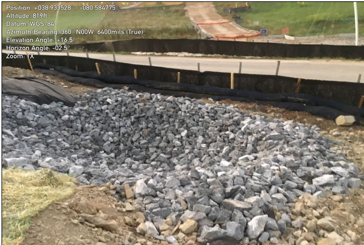
Photo 3: Photo illustrates the rock sump that has been installed near CR 21.
