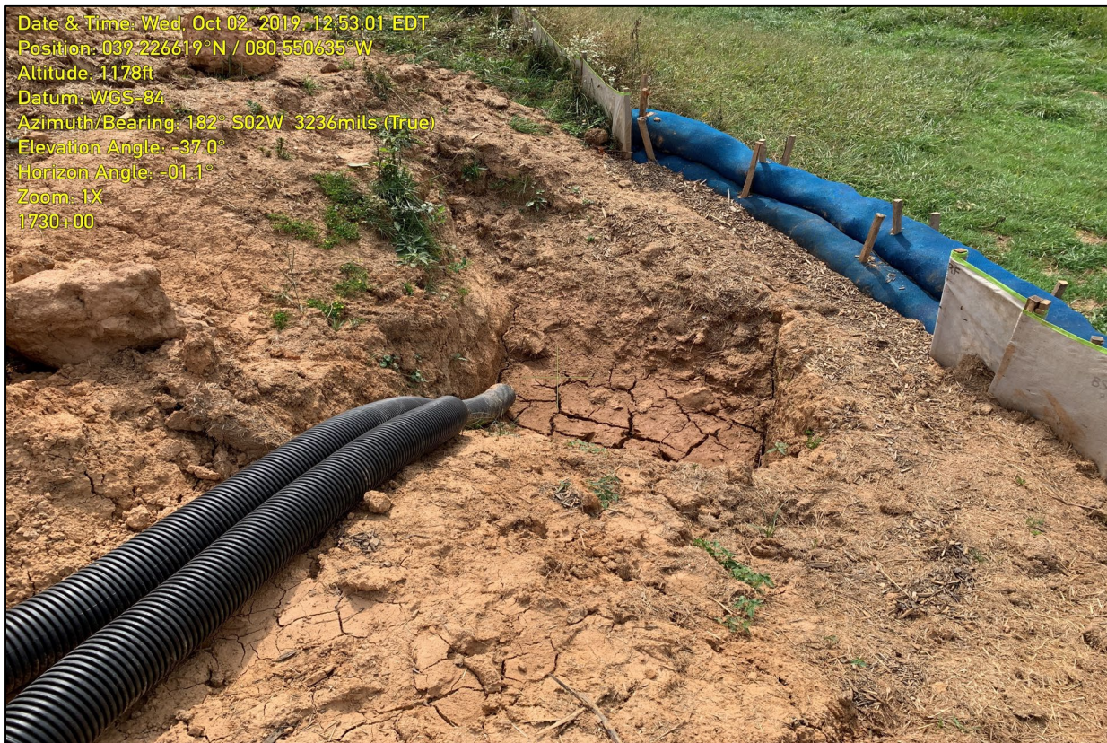
Photo 4: Photo illustrates the additional slope drain and triple stacked CFS that have been added near station 1730+00.
