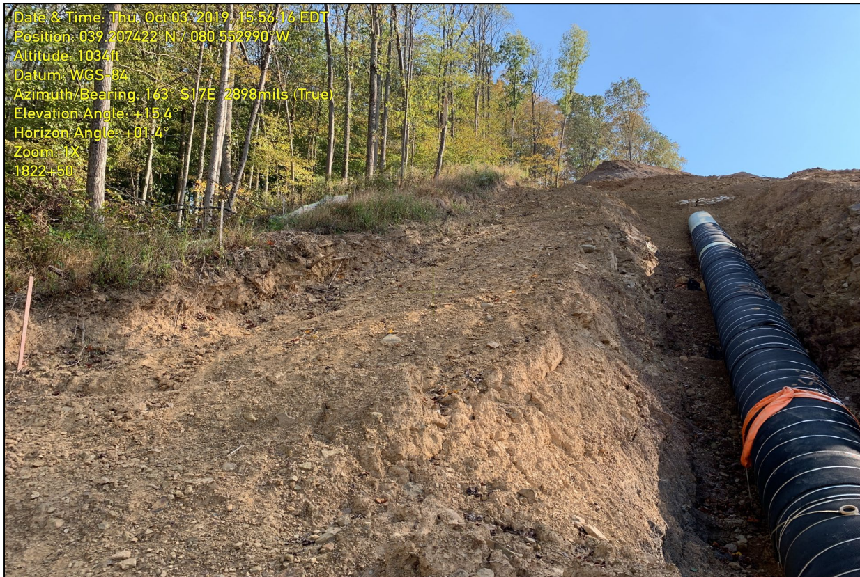
Photo 1: Photo illustrates the regraded slope near Station 1822+50. The area is still in active construction and will be stabilized once complete.
