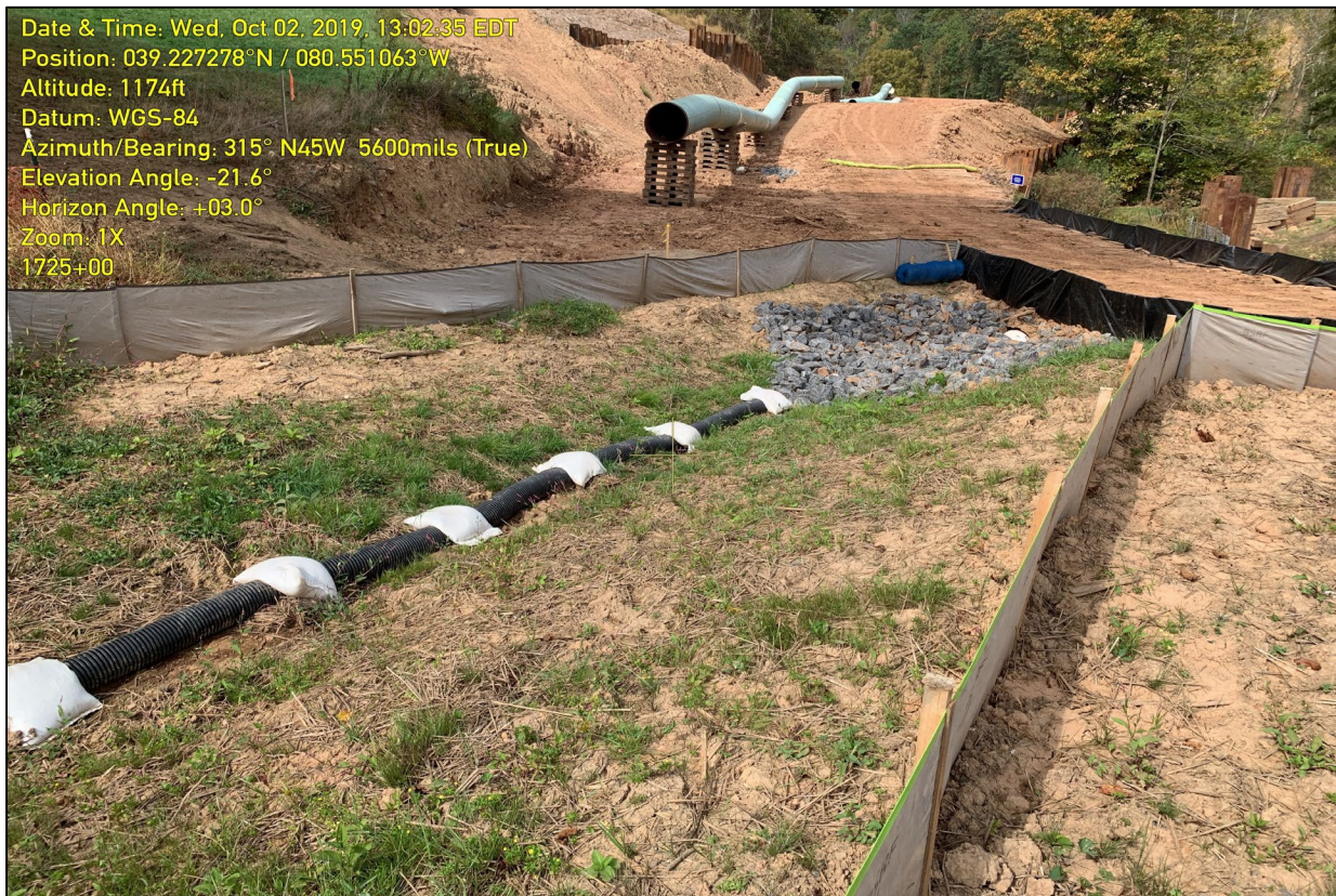
Photo 2: Photo illustrates the clean water diversion that was installed to contain the seep and prevent onsite saturation.
