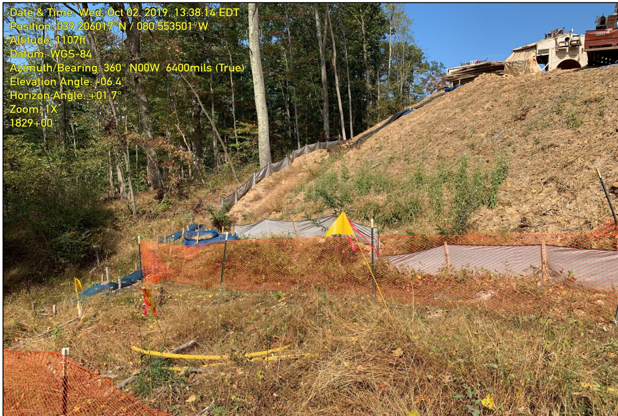
Photo 3: Photo illustrates additional ECDs that have been installed downslope of the inspection area.
