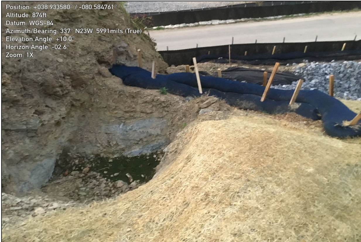
Photo 1: Photo illustrates the repaired and replaced controls upslope of CR 21. An additional row of compost filter sock (CFS), erosion control blanketing (ECB), and super silt fence (SSF) have been installed.
