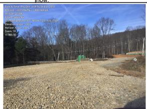
**GPS Location** 37.2060238276495, -80.3941326702235 See photo for GPS location and station number. RCE in place and will assist in Description prevention of track out.
