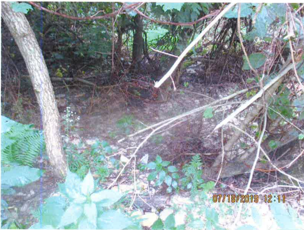
Section of MVP-WB-119 with no perimeter controls installed. Significant Sediment deposits were observed past the LOD throughout the vegetated area downslope of the road.
