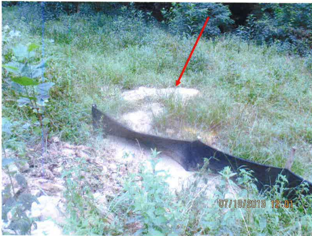
Downslope of Waterbar outlet terminating on slope. Controls overwhelmed with sediment and deposits were present past the LOD and Controls. Arrow depicts sediment deposits.
