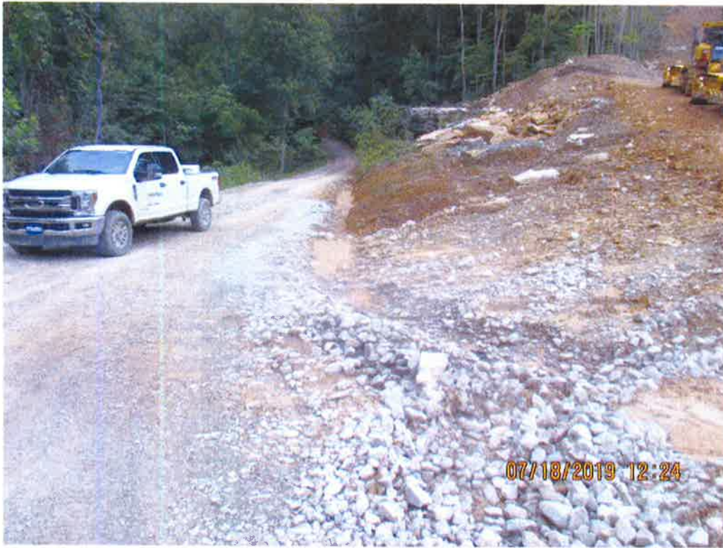
Standing at station No. 4559+96 facing Access Road MVP-WB-119. Sediment deposits present in roadside ditch.
