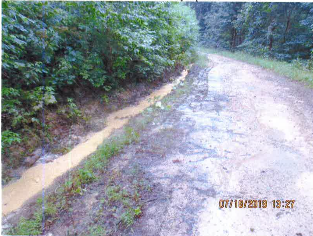
Approximately 200 feet downslope of ROW crossing with MVP-WB-119. SLW being conveyed to culvert.
