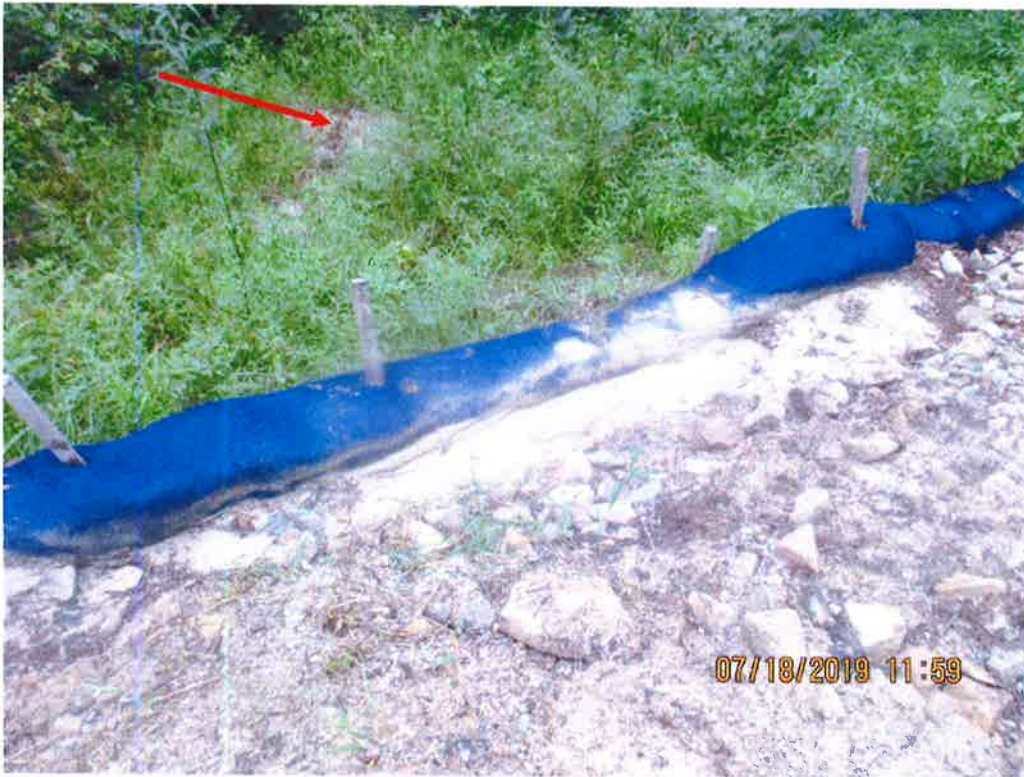
Perimeter controls overwhelmed with sediment with sediment deposits past the LOD. Arrow depicts sediment deposits.
