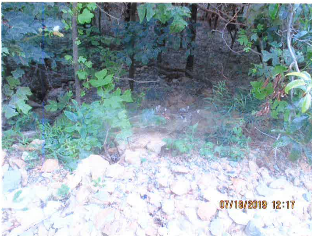
Section along Access road MVP-WB-119 where rock washed out past LOD. No controls present on downslope edge of road. Sediment deposits observed past LOD.
