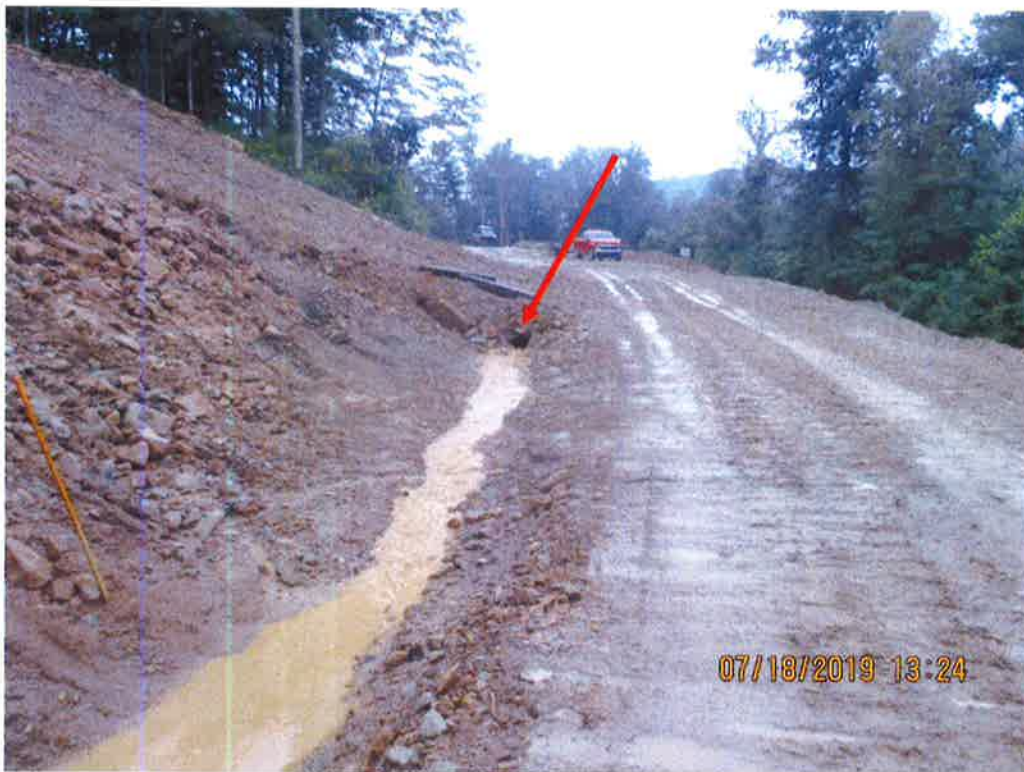
Downslope from where SLW was entering ditch. Arrow depicts culvert that conveys under ROW crossing. No controls present upslope of ditch below station No. 4539+00.
