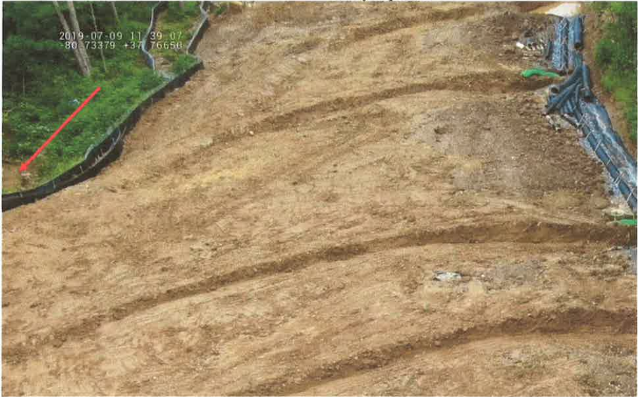
Close up view of additional waterbars added to re-direct run-off to East side of LOD. Arrow depicts deposits of sediment in stream S-T35A.
