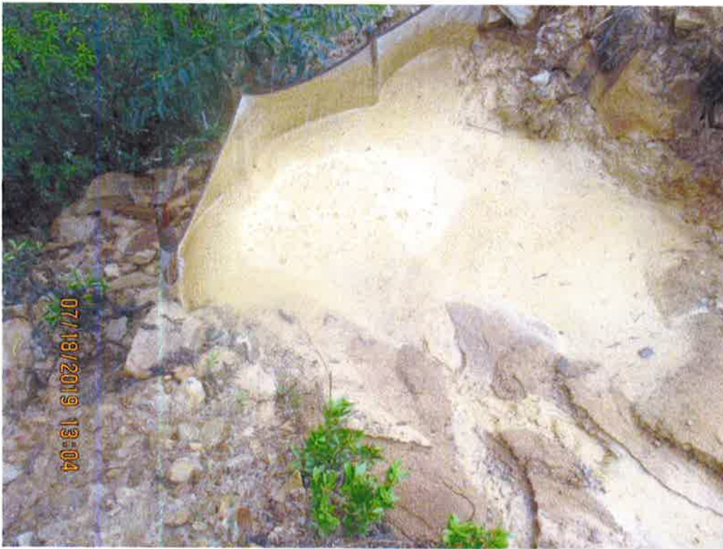
Above station No. 4539+00 during rain event. Sump full of sediment and in need of maintenance. Sediment laden water undercutting silt fence and flowing past LOD.
