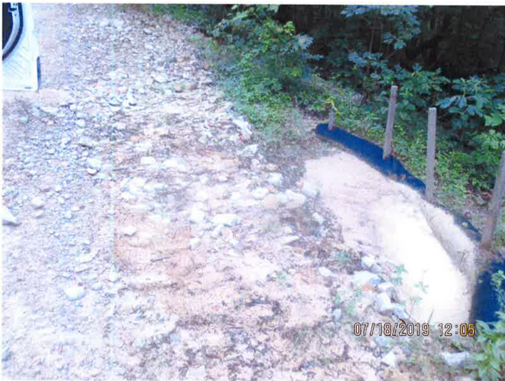
Perimeter controls overwhelmed with sediment along access road MVP-WB-119
