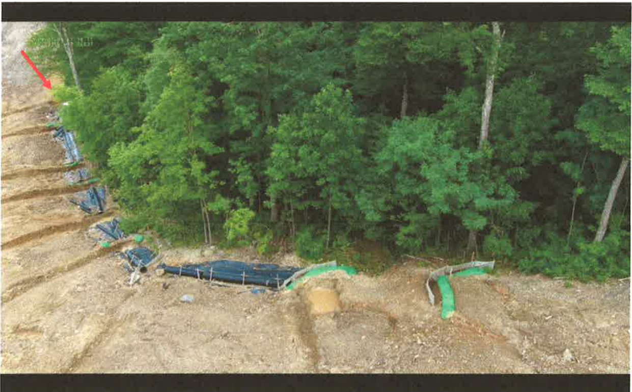
Lower Portion of Slope with flume pipe system. Arrow depicts where single outlet received concentrated flow from Run off and impacts occurred to East side of LOD.
