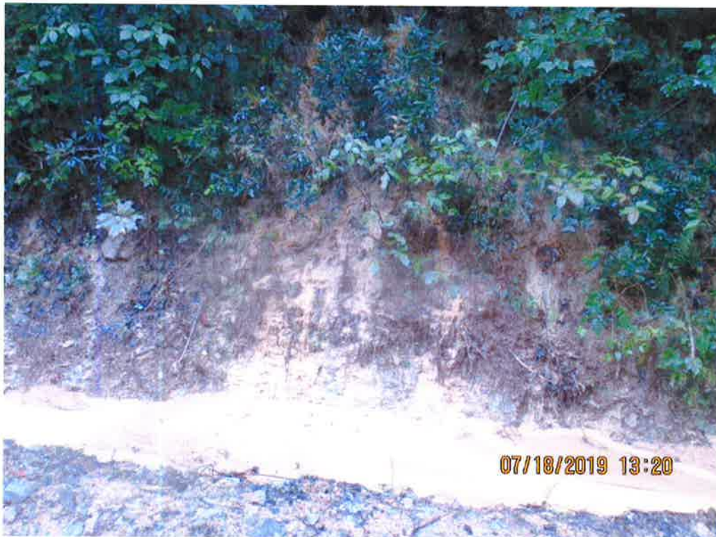
Downslope of failed controls post rain event along Access Road MVP-WB-119. SLW was entering/cascading into the ditch that conveys back downslope towards ROW crossing with access road.
