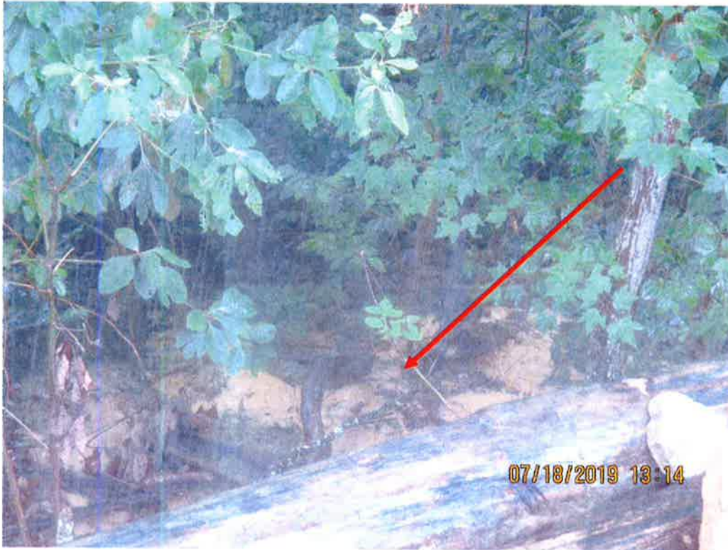
Downslope from Waterbar terminating onto fill slope at station No. 4539+00. SLW observed past controls and LOD conveying downslope.
