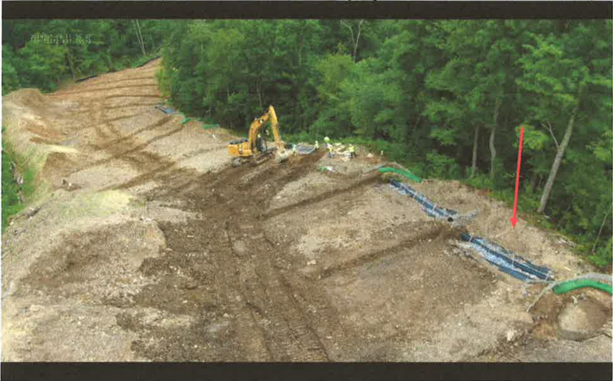
Overview of upper portion of slope near station No. 8634+00. Flume pipe system actively being maintained and enhanced during inspection. Arrow depicts cut original cut that created a “wall” effect not allowing for proper Waterbar outlets to be installed per SWPPP.
