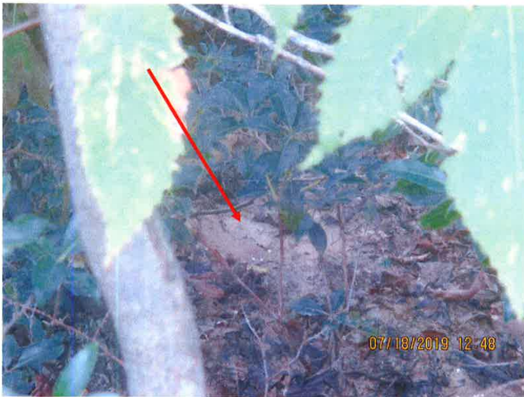
Waterbar outlet on opposite side of ROW at station no. 4559+96. Controls undercut and sediment deposits observed past controls and LOD.
