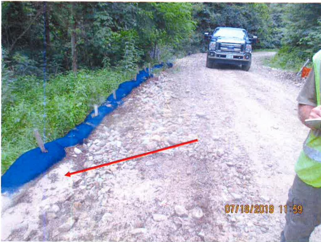
Facing perimeter controls along access road MVP-WB-119. Controls were overwhelmed with sediment.
