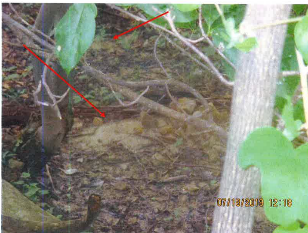
Section along Access road MVP-WB-119 where rock washed out past LOD. No controls present on downslope edge of road. Sediment deposits observed past LOD. Arrow depicts deposits.
