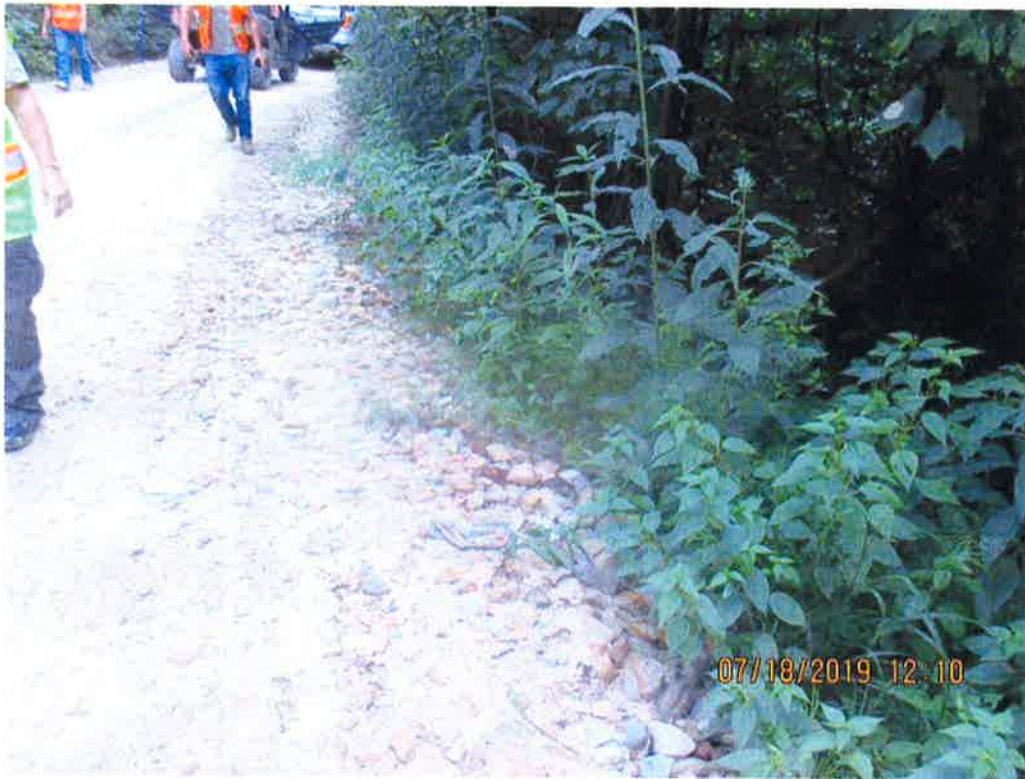
Section of MVP-WB-119 with no perimeter controls installed. Sediment deposits were observed past the LOD.
