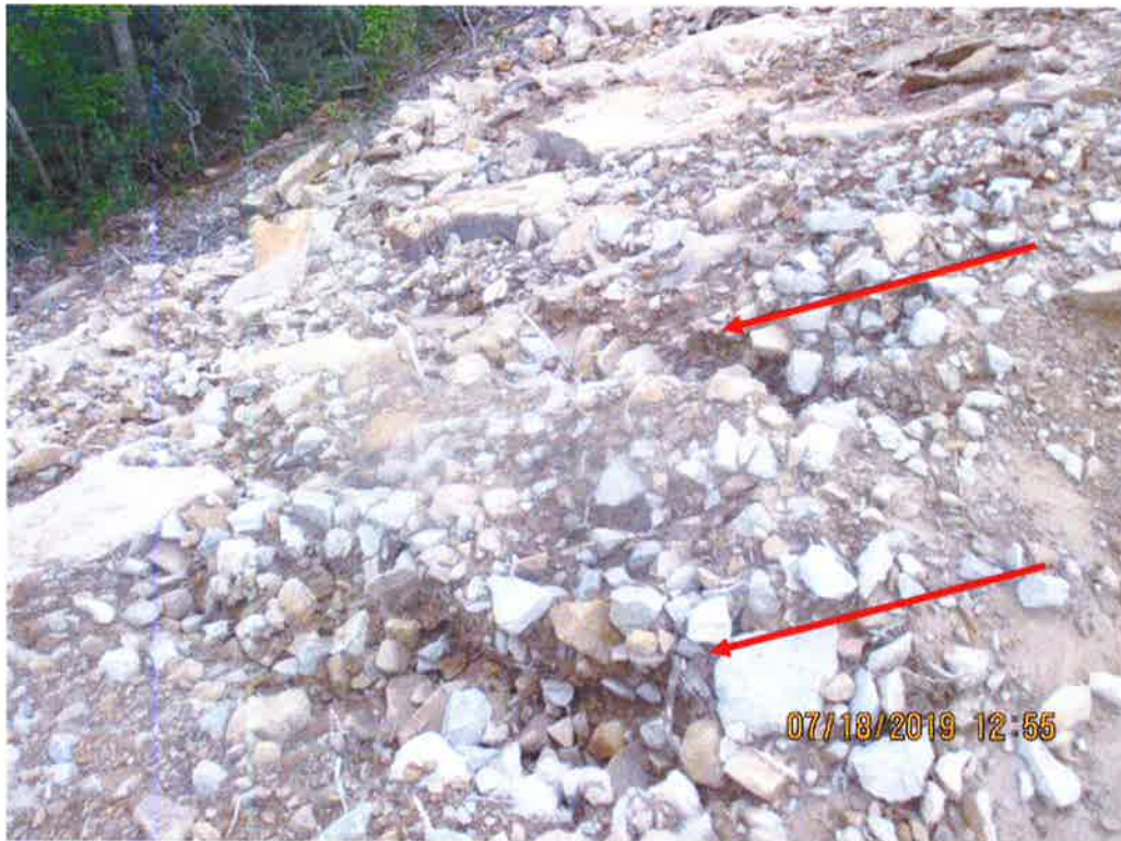
Near station No. 4559+96 erosion present on fill slope. Arrows depict erosion that was observed.
