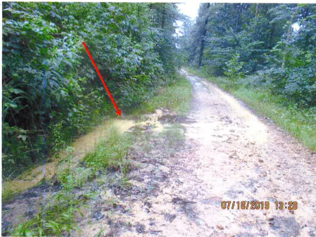
Culvert inlet that conveys under unapproved access road.
