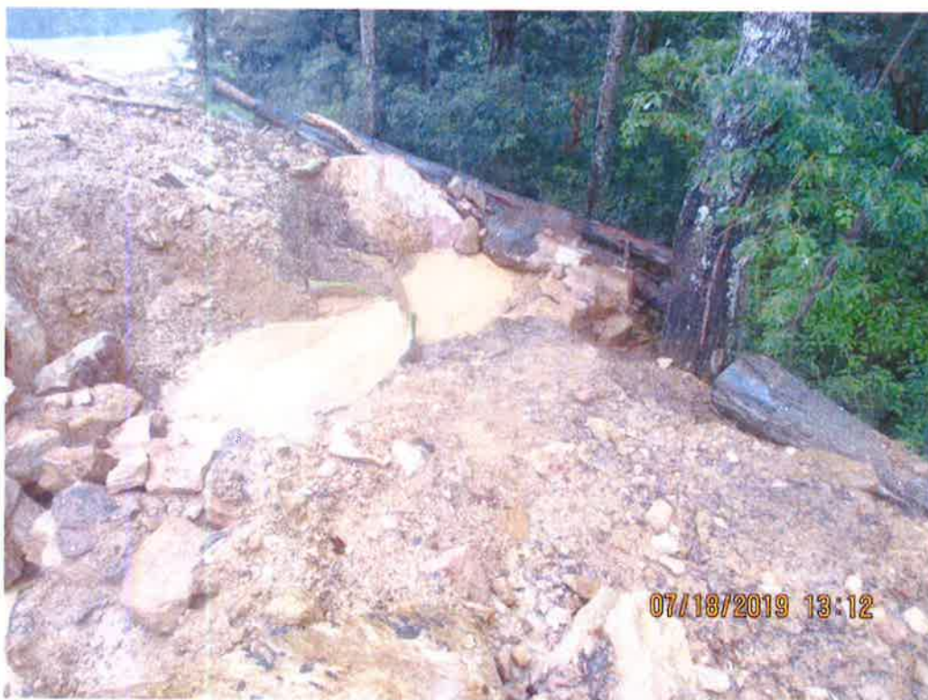
Waterbar terminating onto fill slope at station No. 4539+00. Large rocks installed as checks in eroded channel. SLW was flowing under and through these checks overwhelming controls.
