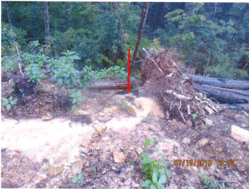
Sediment laden water flowing off ROW and through log pile during rain event. No perimeter controls were present at the base of the slope. Arrow depicts where SLW was flowing through log pile.
