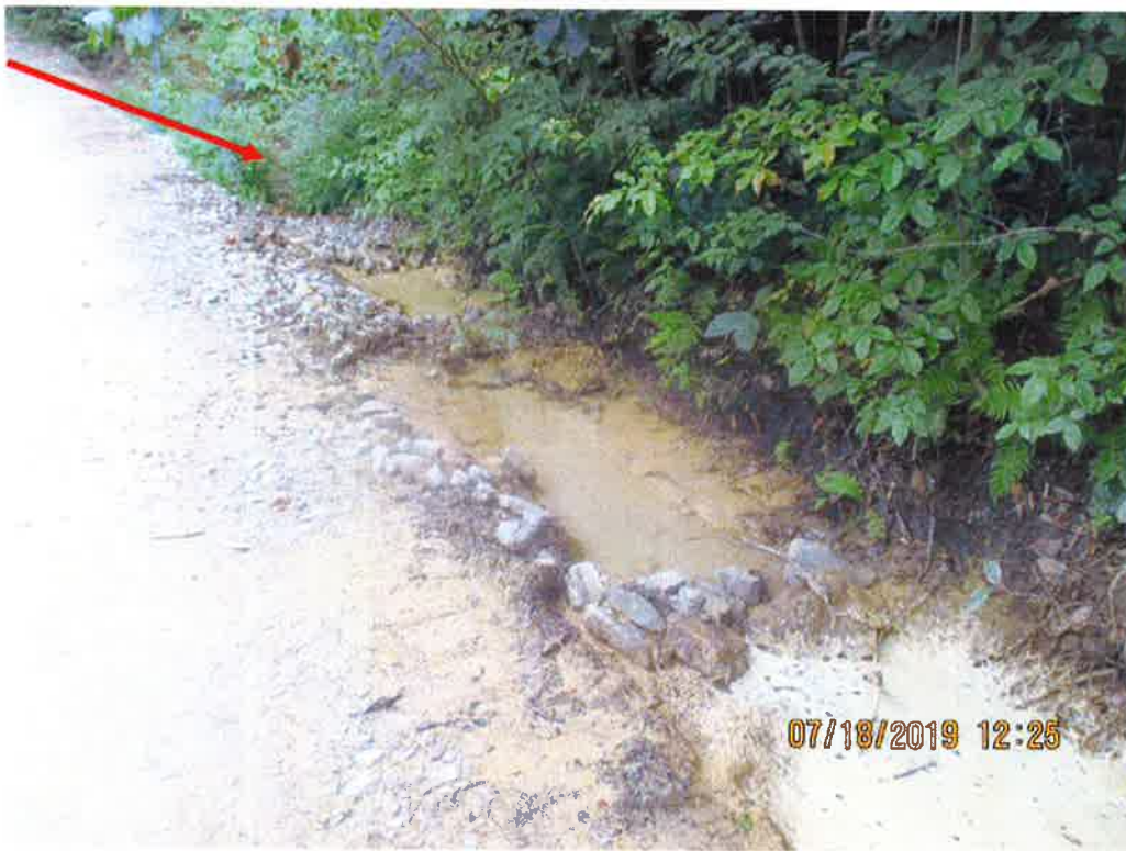
Standing downslope from station No. 4559+96 from Access Road MVP-WB-119 facing towards MVP ROW. Sediment deposits present in roadside ditch.
