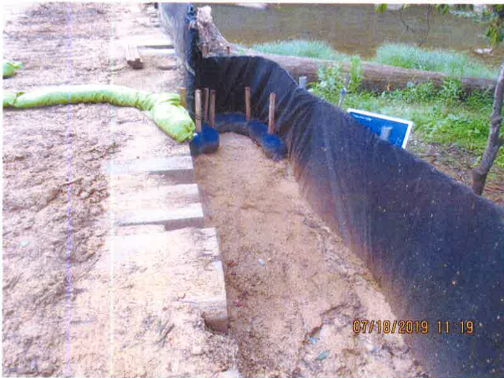
Sediment deposited behind controls on NW side of Bridge.
