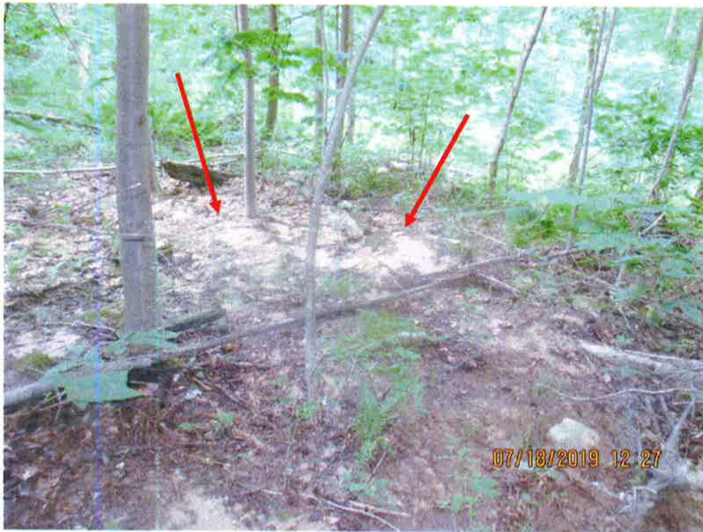
Downslope of culvert outlet. Significant sediment deposits present past controls and LOD. Arrow depicts examples of deposits observed.
