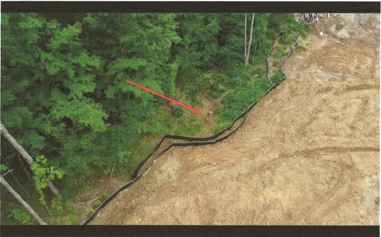
View of Stream S-T35A at station No. 8634+00 at the West side of the LOD. Arrow depicts additional super silt fence installed post impacts. Sediment deposits observed in Stream at time of inspection.
