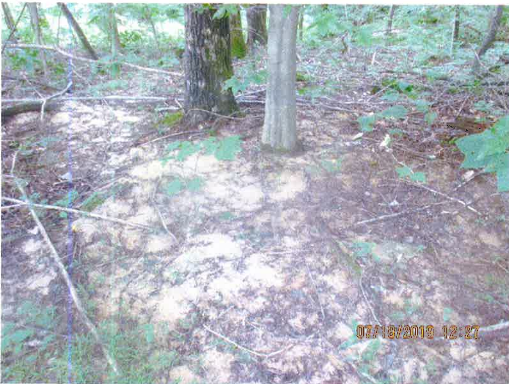
Downslope of culvert outlet. Significant sediment deposits present past controls and LOD.
