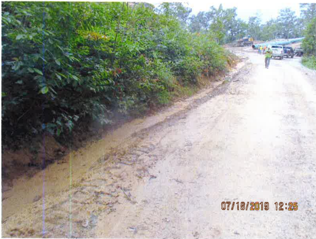
Standing downslope from station No. 4559+96 from Access Road MVP-WB-119 facing towards MVP ROW. Sediment deposits present in roadside ditch.
