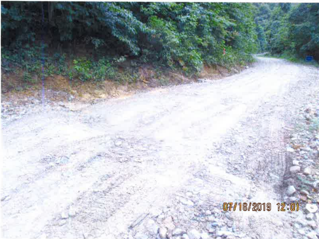
Waterbar installed on Access Road MVP-WB-119. Ditch line had rock checks present. Sediment deposits overwhelmed perimeter controls downslope of Waterbar.
