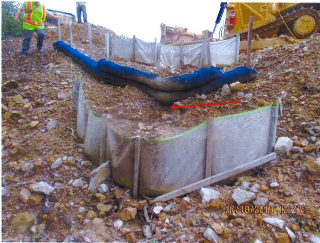
Waterbar outlet on opposite side of ROW at station no. 4559+96. Controls undercut and sediment deposits observed past controls and LOD. Arrow depicts undercut controls.
