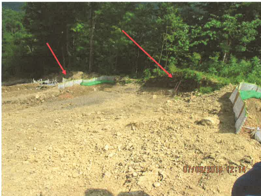
Standing above Stream S-T35A near station No. 8634+00 facing towards the East side of LOD. Arrows depict how the original cut to grade ROW created a wall preventing proper Waterbar outlet installation.
