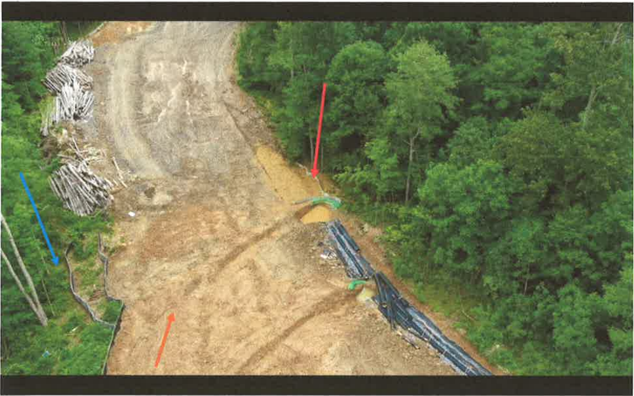
View of East and west side of MVP ROW and LOD. Red arrow depicts where last Waterbar at base of slope was overwhelmed and impacts occurred. Blue arrow depicts stream S-T35A. Orange arrow depicts where additional waterbars were installed to redirect run-off towards East side of LOD.
