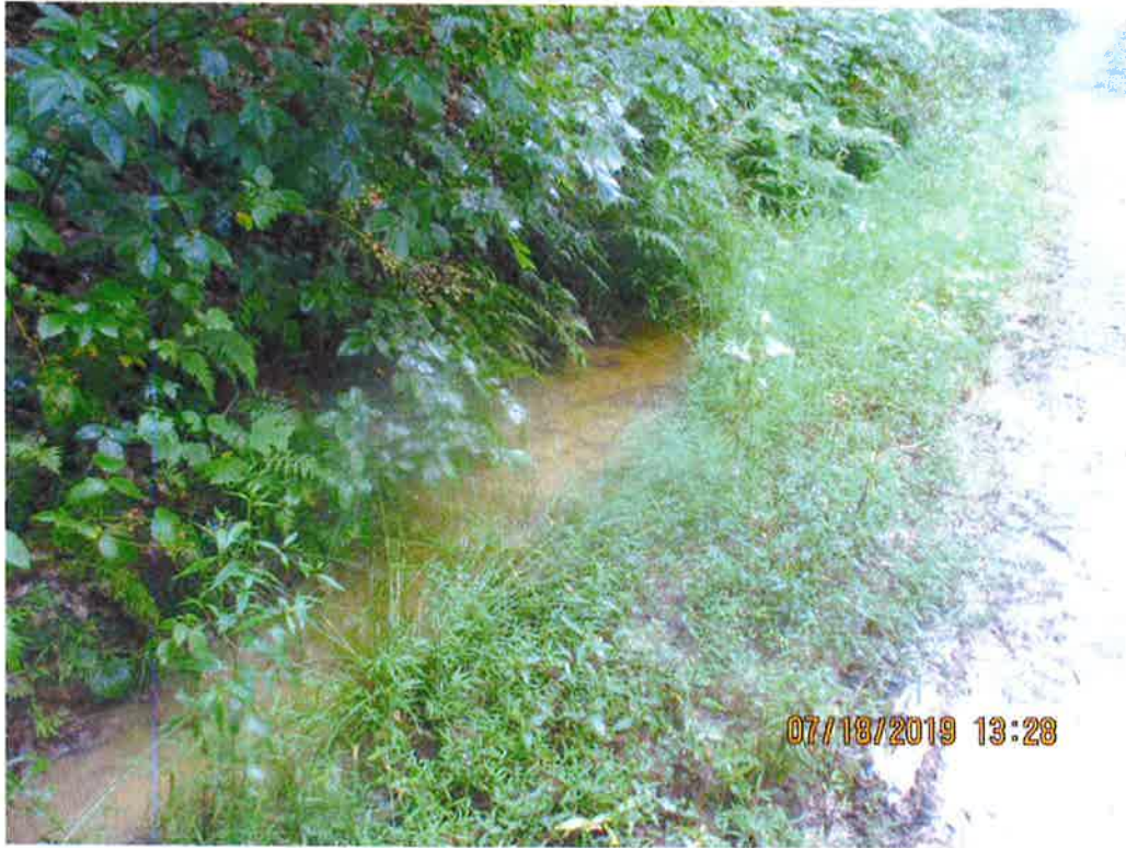
Upslope of culvert inlet receiving sediment laden water. Run-off present in ditch line distinguishably different than what was originating from upslope and entering culvert.
