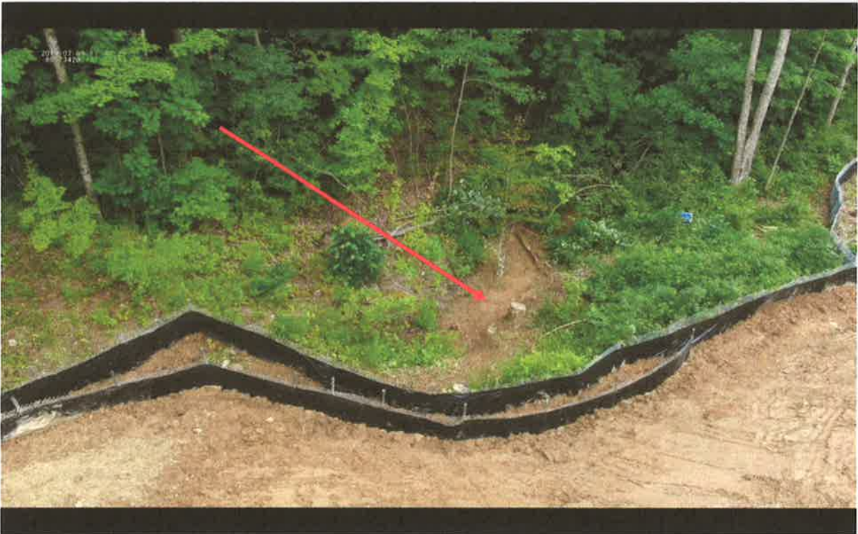
Close up view of additional waterbars added to re-direct run-off to East side of LOD. Arrow depicts photo of sediment deposits in stream S-T35A.
