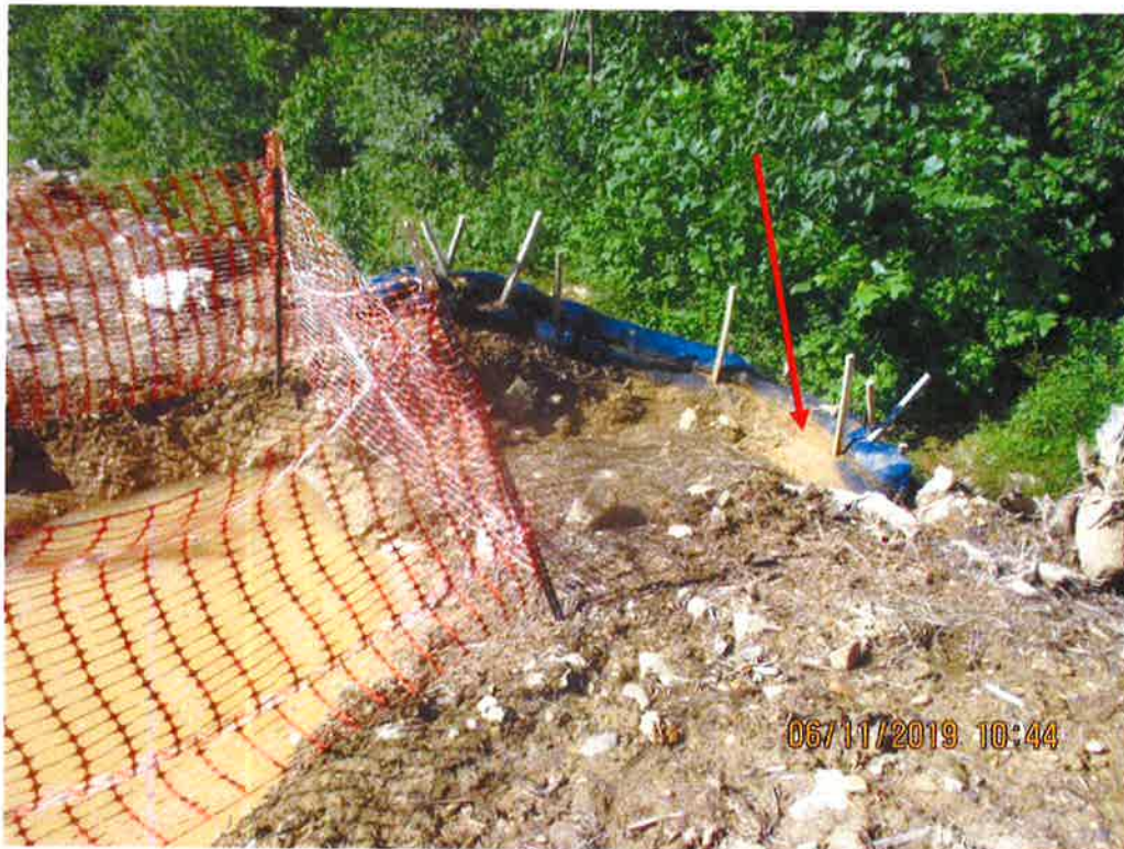
Standing above Station No. 7604+41. Controls below Waterbar and sump that had sediment present due to erosion. Perimeter controls being overwhelmed with sediment.
