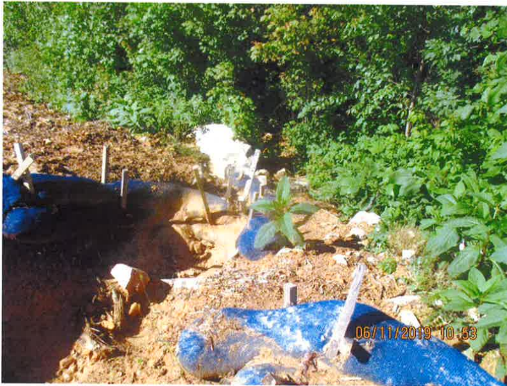
Standing above Station No. 7604+41. Perimeter controls overwhelmed with sediment.
