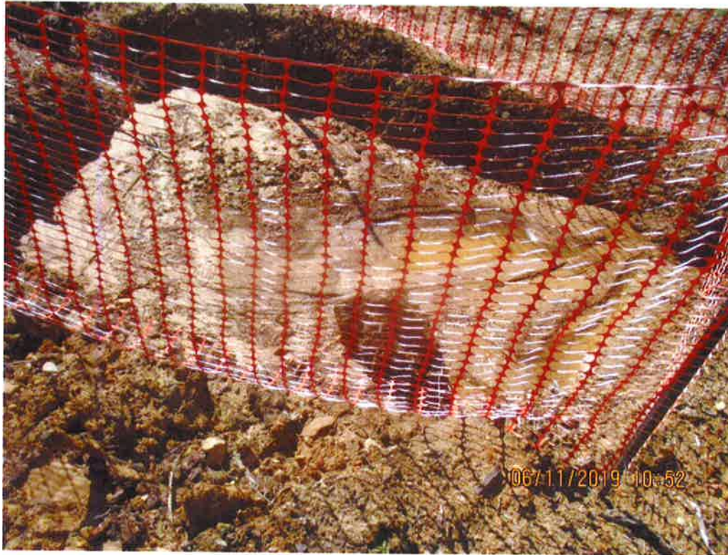
Standing above Station No. 7604+41. Waterbar had sediment being deposited in it from erosion causing sump to be full of sediment.
