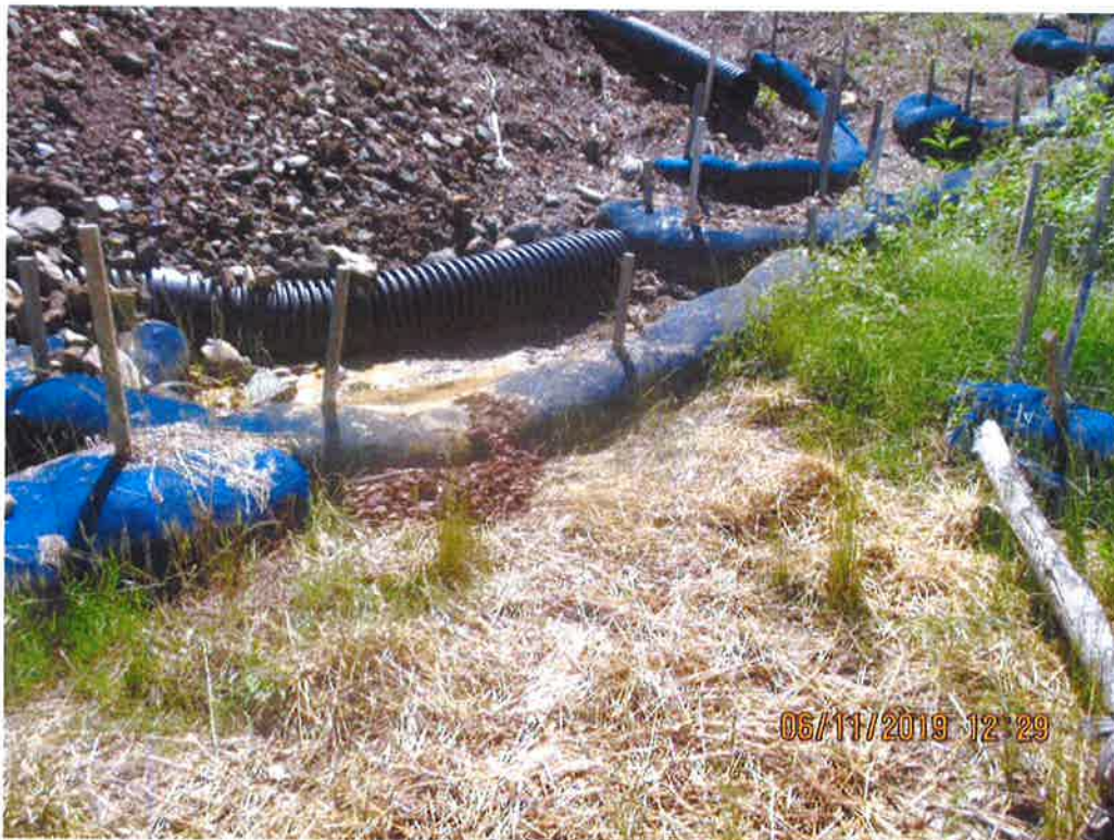
Standing at station No. 7636+00 at Waterbar outlet and slope drain. Slope drain was being undercut. Sediment was overwhelming perimeter control. Control in need of maintenance.
