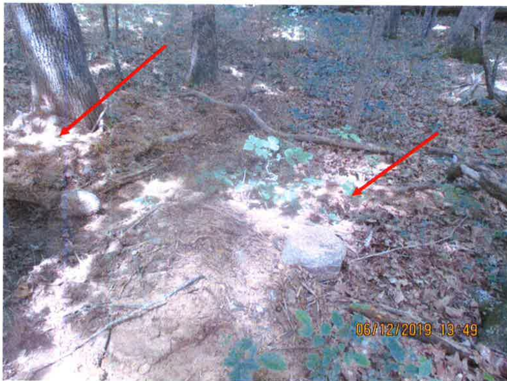
Sediment Deposits below and past controls/LOD at station No. 9780+00. Arrow depicts deposits.
