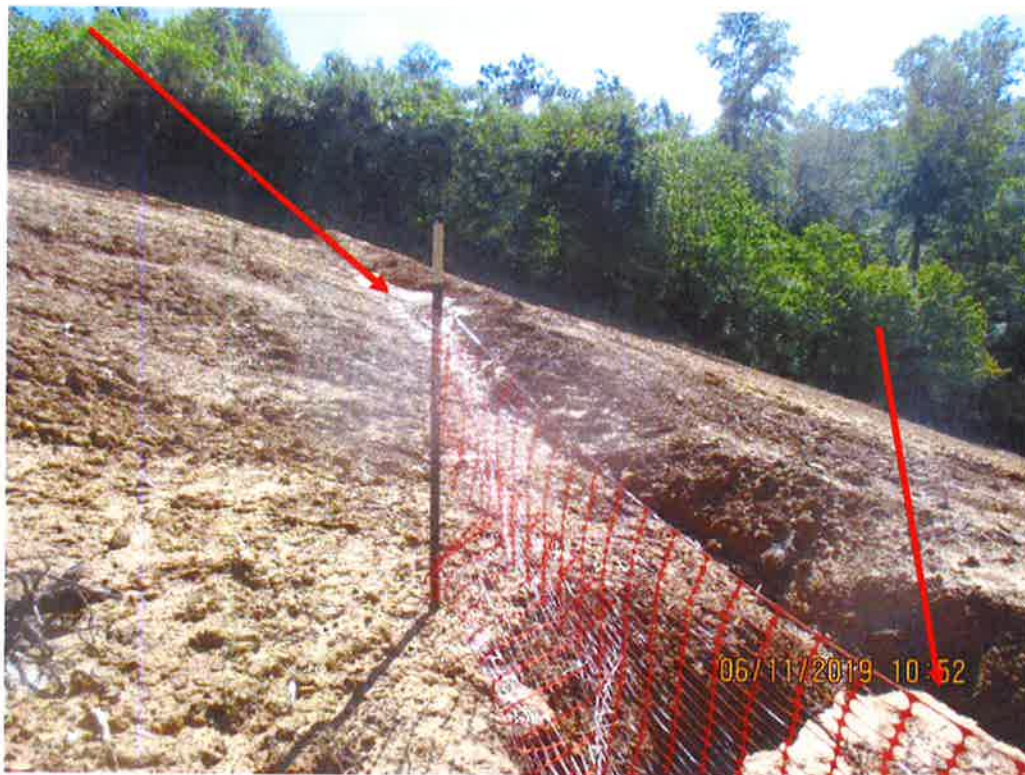
Standing above Station No. 7604+41. Waterbar had sediment being deposited in it from erosion upslope. Sump was full of sediment and needed maintained. Arrow depicts sediment in Waterbar and sump.
