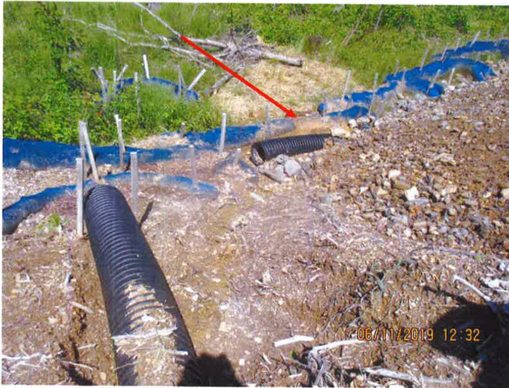
Standing at station No. 7636+00 at Waterbar outlet and slope drain. Slope drain was being undercut. Sediment was overwhelming perimeter control. Sediment deposits observed past controls and LOD.
