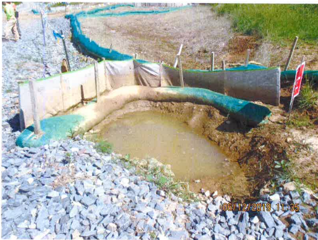
Controls added on edge of LOD to control run-on from adjacent property disturbance.
