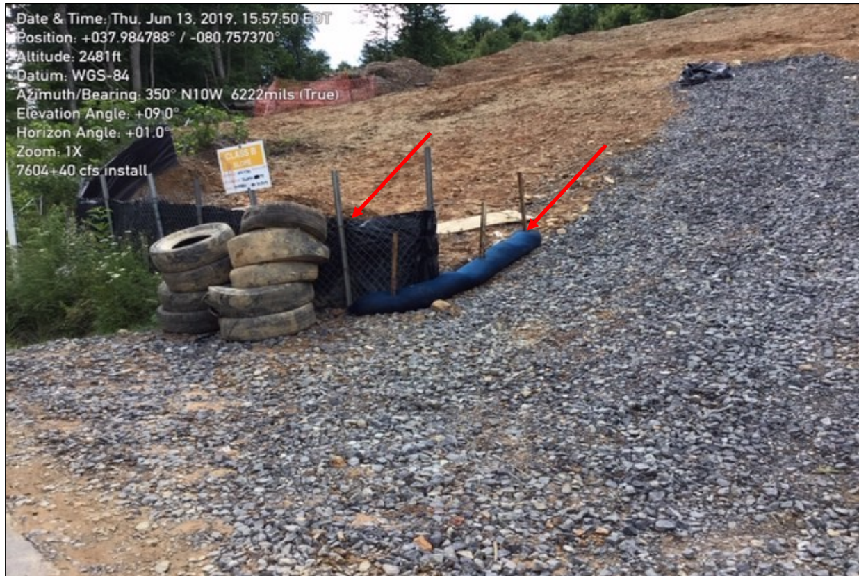
Photo 5: Photo illustrates the additional ECDs, including CFS and supersilt fence (SSF) that have been installed along Crosier Road.
