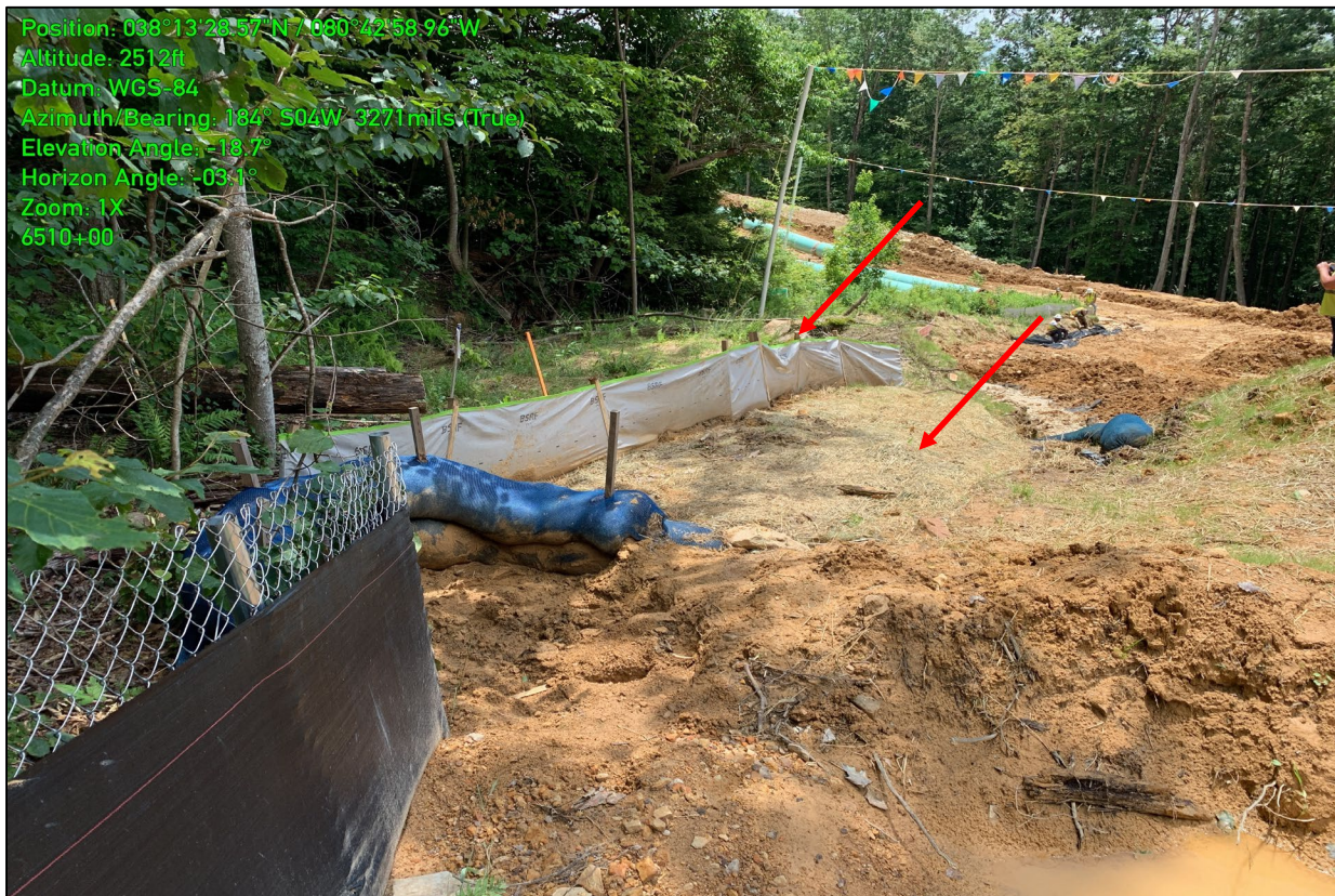
Photo 10: Photo shows the additional P1 silt fence and temporary stabilization that has been installed near Station 6510+40.
