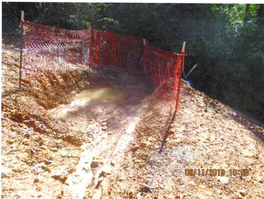
Above Lower Krosier Road crossing. Erosion present on ROW above Waterbar. Sediment being deposited in Waterbar and sump, overwhelming sump and perimeter controls near station no. 7604+41.
