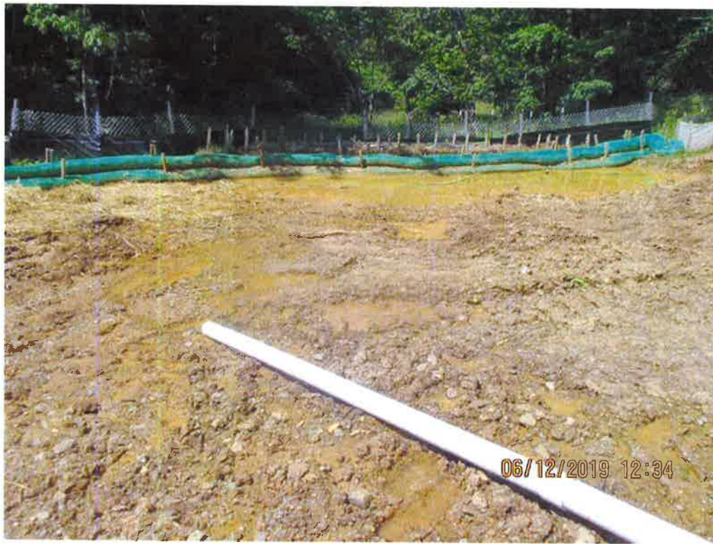
Pipe slope drain terminating onto ROW above controls (Dargo silt fence).
