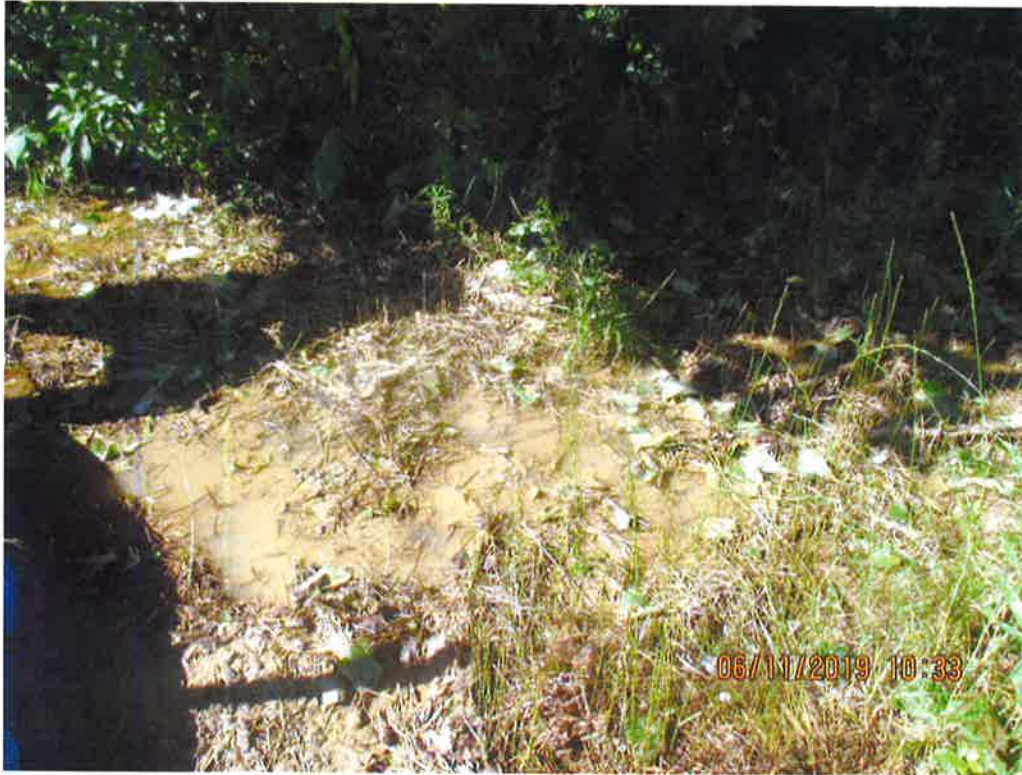
Downslope of Krosier Road Crossing near station No. 7576+01. Sediment laden water (SLW) and deposits were present past controls and LOD.
