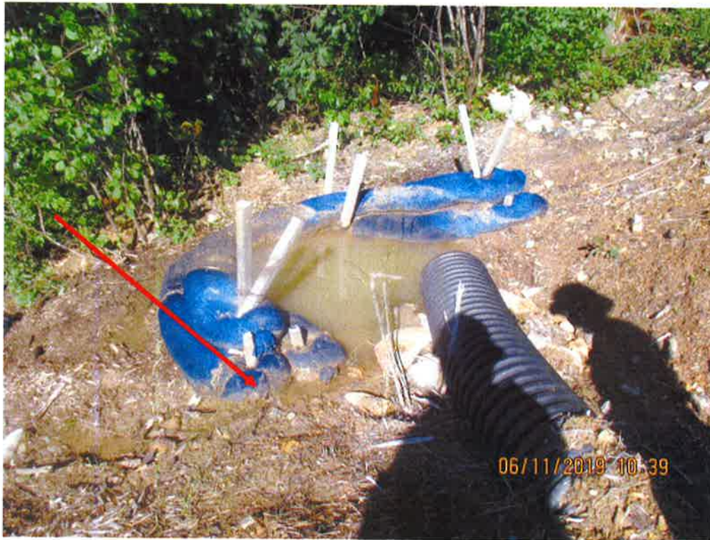
Below upper Krosier Road crossing near station no. 7576+01 facing downslope below Waterbar outlet. Arrow depicts evidence of Run-off flowing around controls and causing erosion downslope of controls was observed.
