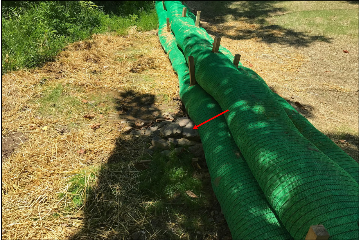
Photo 3: The rock energy dissipater shown in the photo is the outlet of the subterranean drains near the Dargo pond.
