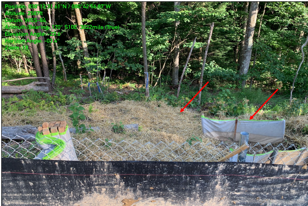
Photo 6: Photo illustrates the temporary stabilization and additional ECDs that have been installed near Station 6508+30
