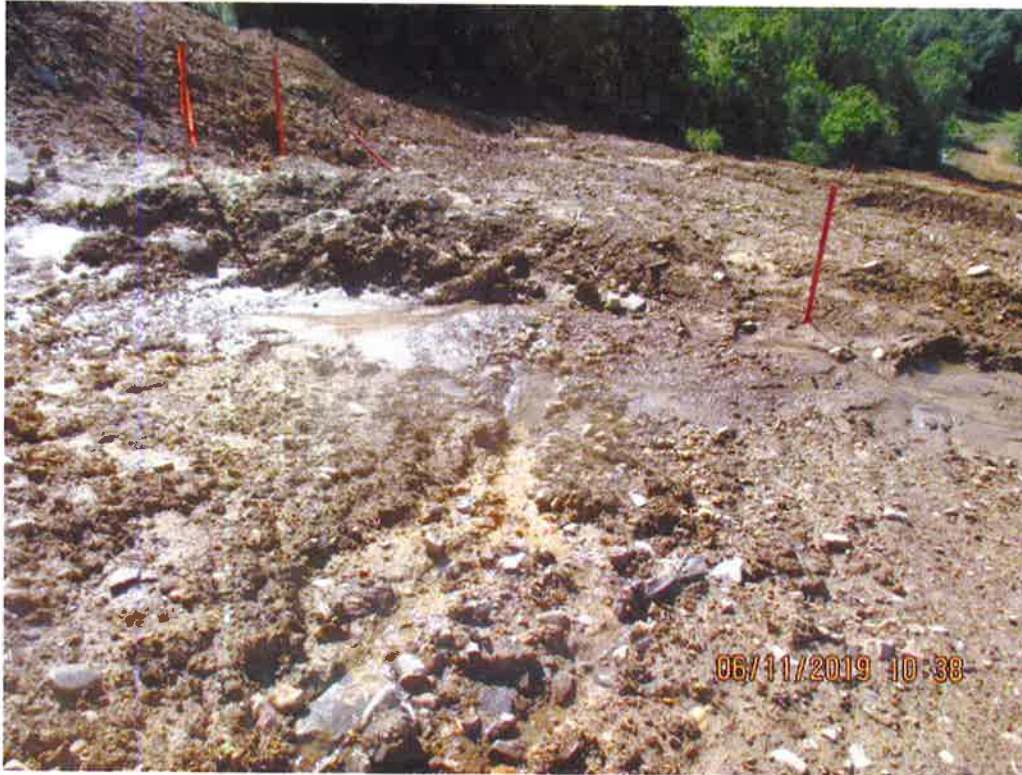
Below upper Krosier Road crossing near station no. 7576+01 facing South at Waterbar. Erosion present on slope due to seep running onto ROW. Sediment deposited in Waterbar.
