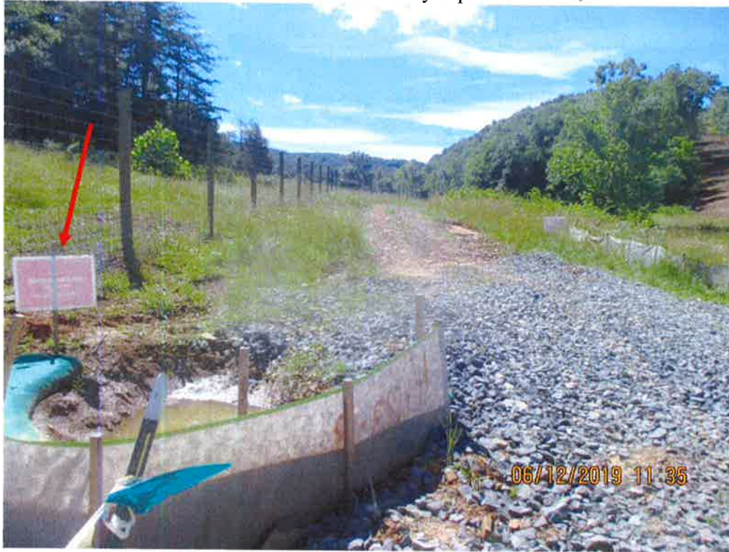
Above Anne's Branch crossing near station 9744+00. Facing upslope of MVP ROW. Erosion ongoing on road as well as slope above road. Arrow depicts LOD.
