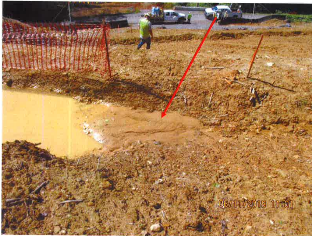
Above Lower Krosier Road crossing. Erosion present in Waterbar causing Sediment to be deposited in sump. Sump needed maintained.
