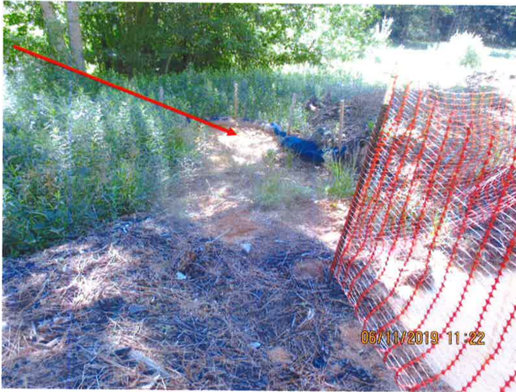
Facing South (Downslope) at station No. 7609+50. Waterbar outlet controls overwhelmed with SLW and deposits.
