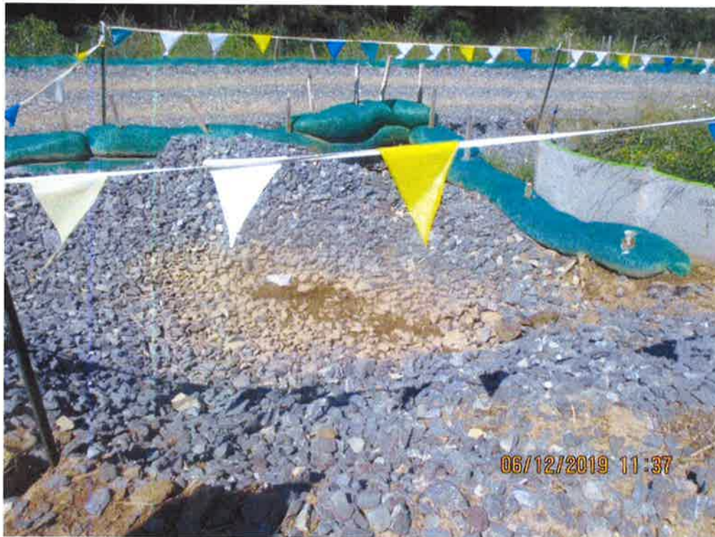
Culvert outlet terminating in sump along AR 227.
