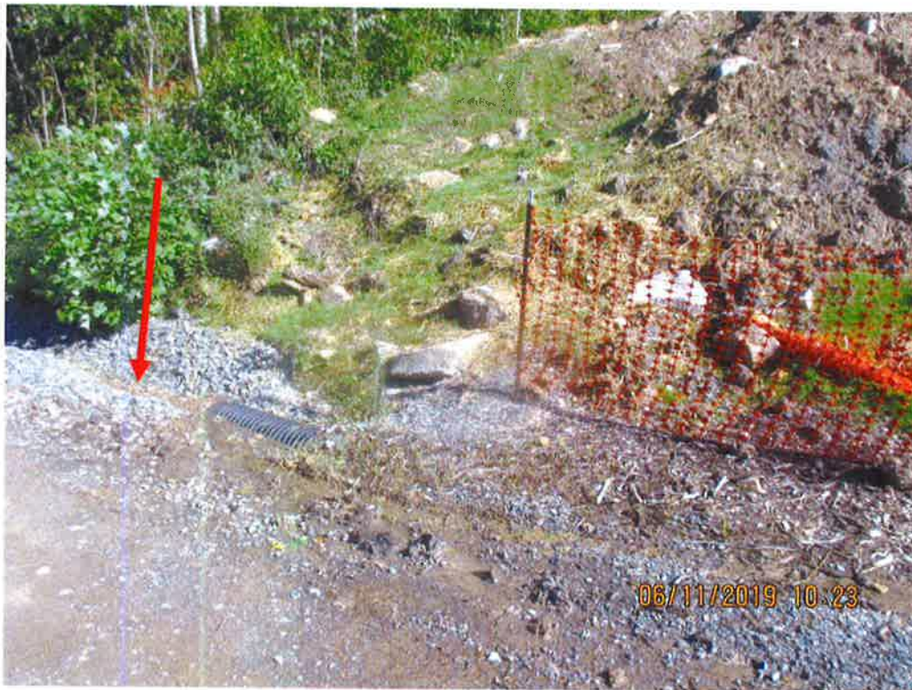
Culvert outlet with sediment deposits in ditch line. Erosion present on slope above outlet. Arrow depicts deposits present in ditch.
