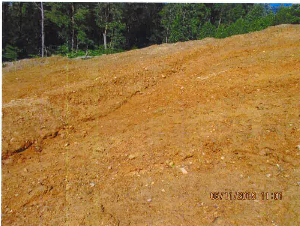
Above Lower Krosier Road crossing. Erosion present in Waterbar near station no. 7604+41.
