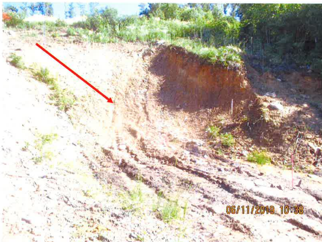
Below upper Krosier Road crossing near station no. 7576+01 facing North. Erosion present on slope due to seep running onto ROW.
