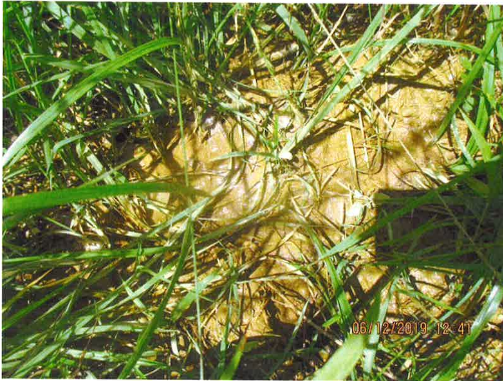
Below Dargo silt fence. Sediment deposits observed past LOD and low-lying area not delineated as a wetland.
