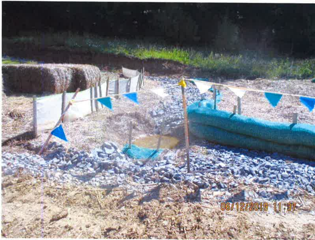
French drain installed at base of cut slope. Drain terminated into sump with controls and conveys under ROW to outlet that has sump present with controls.
