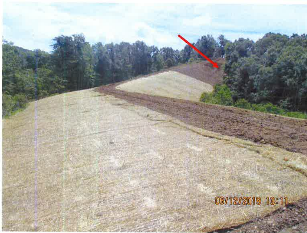
Upslope of Dargo silt fence. Facing South towards AR-221. Arrow depicts where dozer work was ongoing during inspection and controls needed maintenance.
