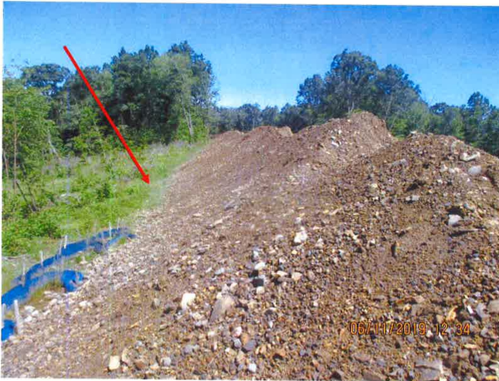
Spoil pile near station No. 7636+00. No perimeter controls at the base of pile. This is an area of concern due to the potential for sediment to be deposited past the LOD.
