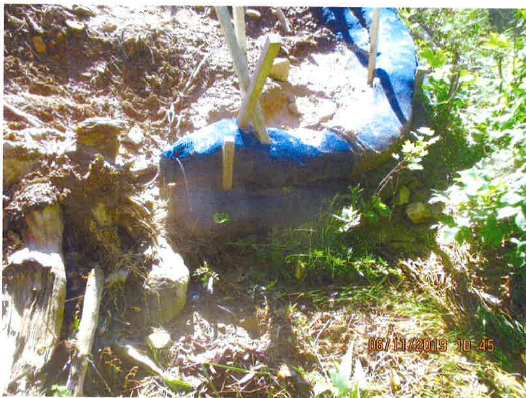
Downslope of Waterbar outlet near No. 7604+41. Perimeter controls in need of maintenance. Sediment deposited behind perimeter controls. Sediment deposits observed past controls and LOD.
