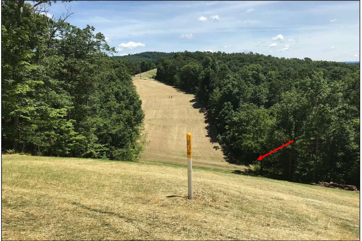
Photo 1: Photo illustrates the stabilized slope near the Dargo Pond. The pipe has been installed in this area. The red arrow is the drainage swale in the valley, leading to the Dargo Pond.
