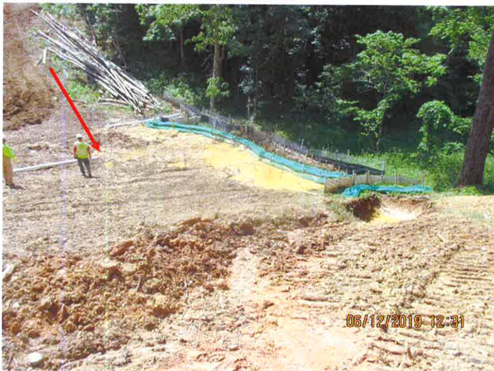
Dargo silt fence. Pipe slope drain terminating on ROW and not extended to edge of LOD. Arrow depicts slope drain outlet.
