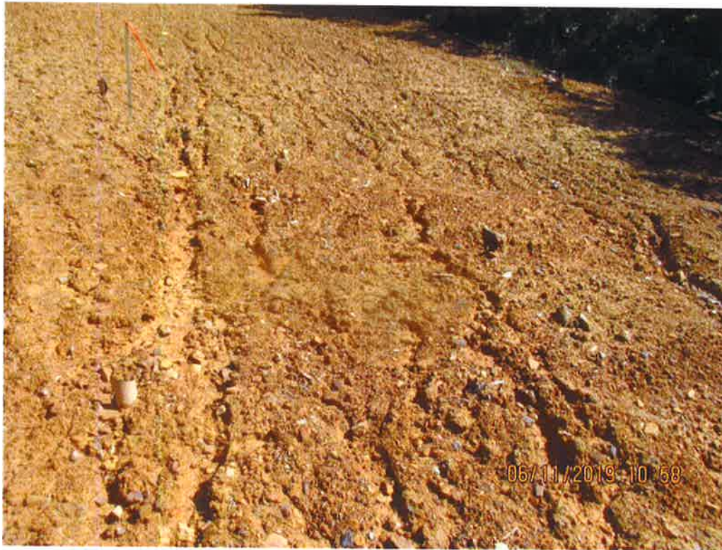
Above Lower Krosier Road crossing. Erosion present on ROW above Waterbar. Facing upslope near station no. 7604+41.
