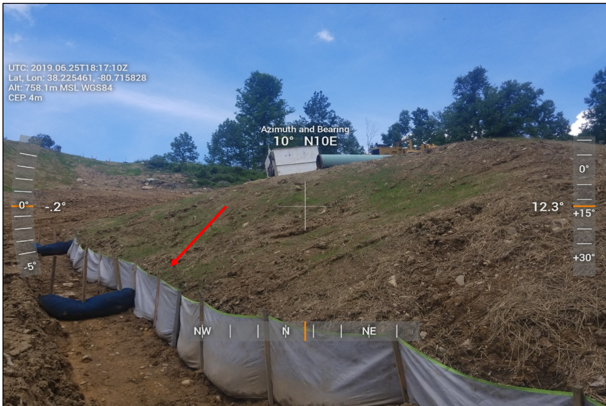
Photo 8: Photo shows the row of P1 fencing that has been installed to separate the stockpile from the waterbar near Station 6508.
