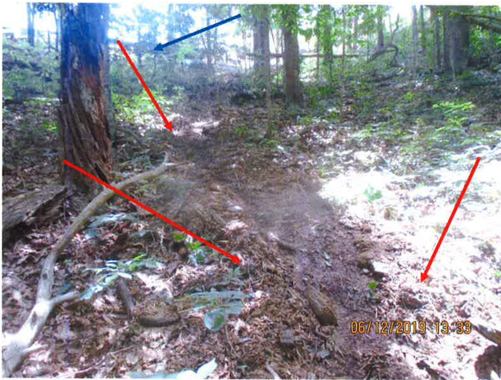
Scoring and sediment deposits below controls at station No. 9780+00. Red Arrow depicts deposits. Blue arrow depicts controls at edge of LOD.
