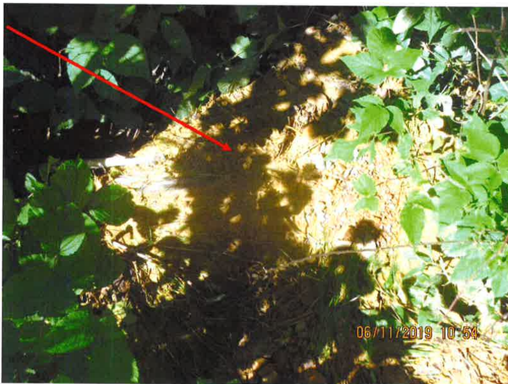
Standing above Station No. 7604+41. Perimeter controls overwhelmed with sediment. Sediment deposits observed past controls and LOD.
