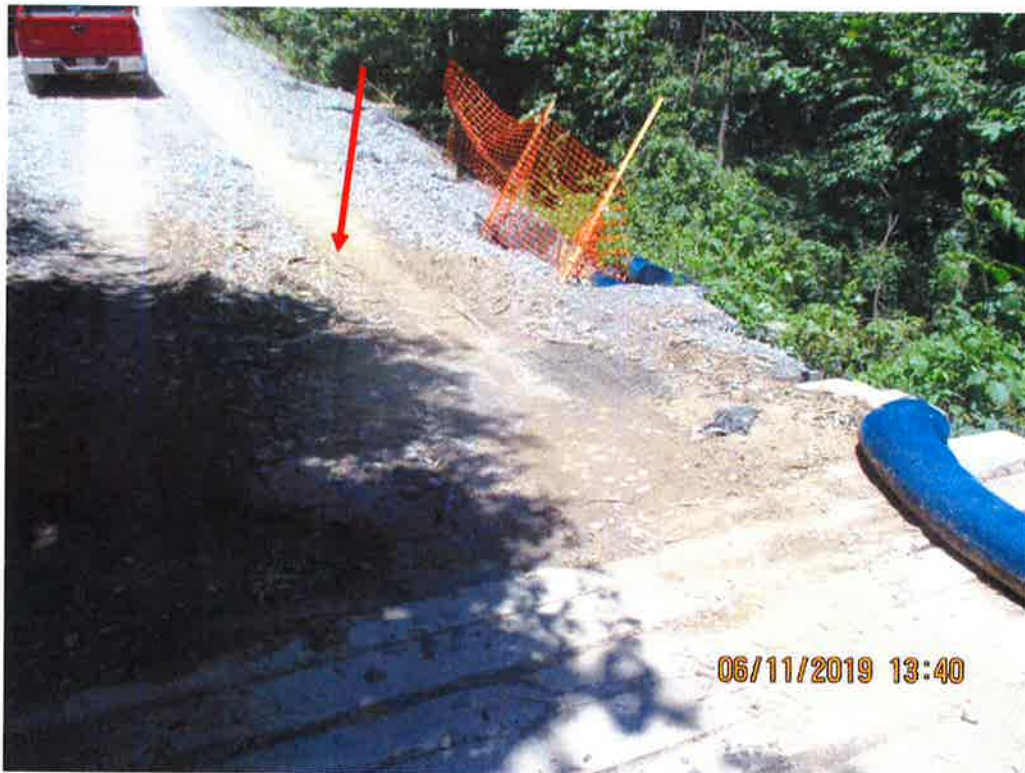
Facing up grade on Access Road 192.5 at wetland crossing W-V6. SWPPP detailed Waterbar above this crossing. Waterbar had been eroded and was barely distinguishable. Arrow depicts where Waterbar was installed and terminating on road bank (slope).
