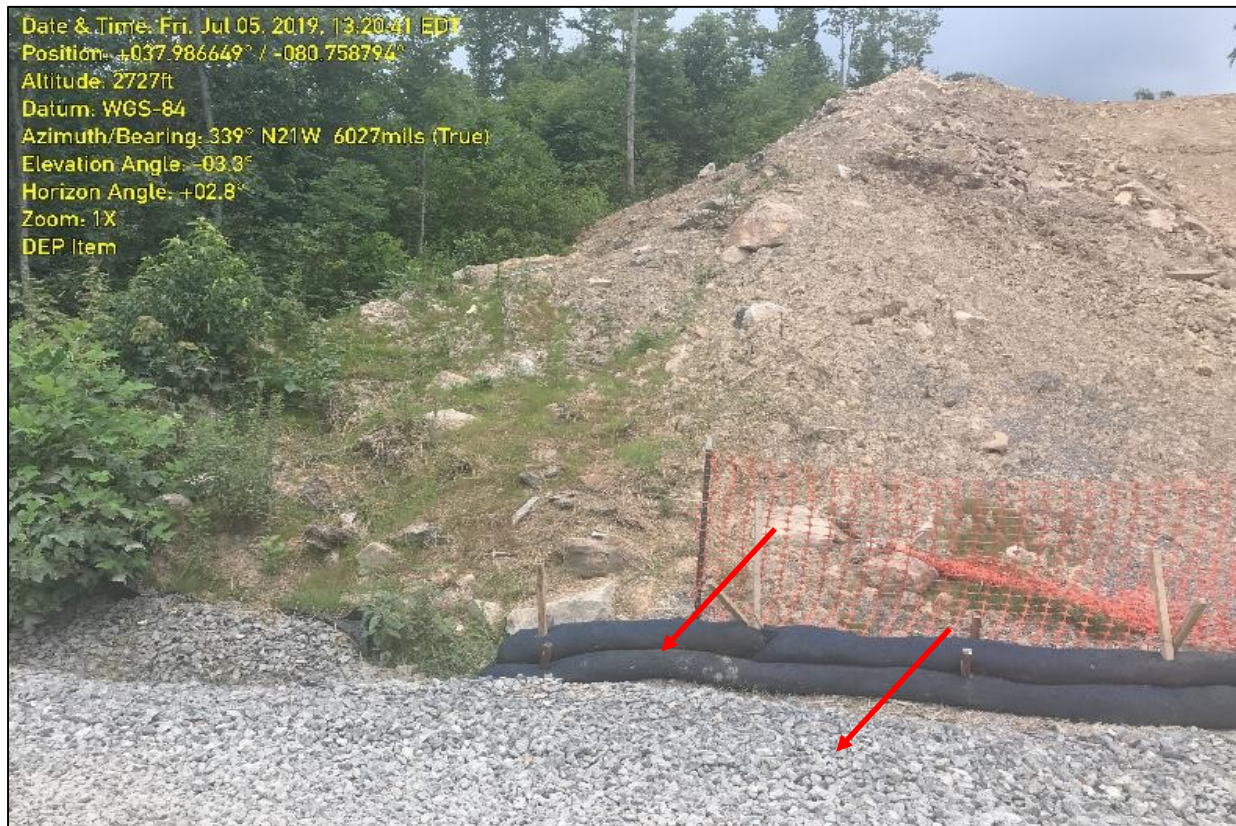
Photo 6: Photo illustrates the additional ECDs – CFS and additional gravel – that have been installed near the Crosier Road Culvert.
