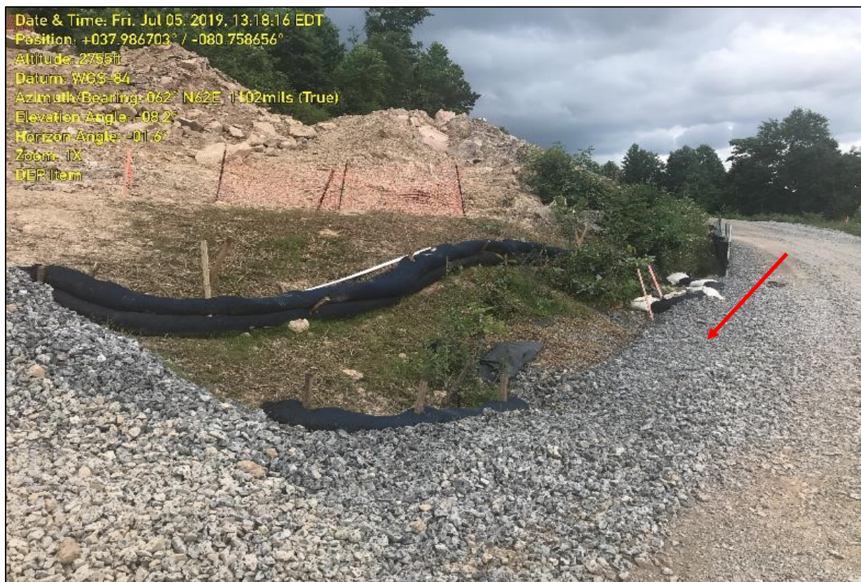
Photo 4: Photo illustrates the additional gravel that has been installed along Crosier Road.
