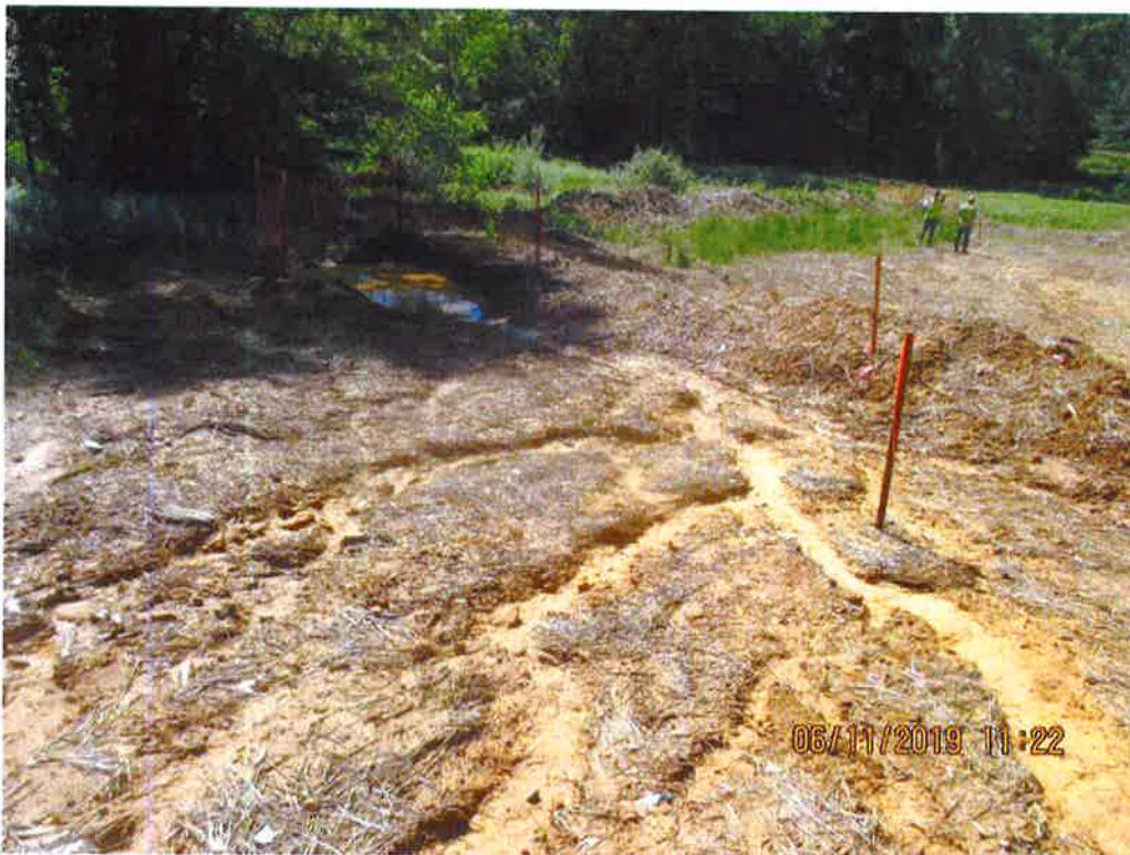
Facing South (Downslope) at station No. 7609+50. Waterbar receiving sediment due to erosion on slope. Controls overwhelmed with SLW and sediment.
