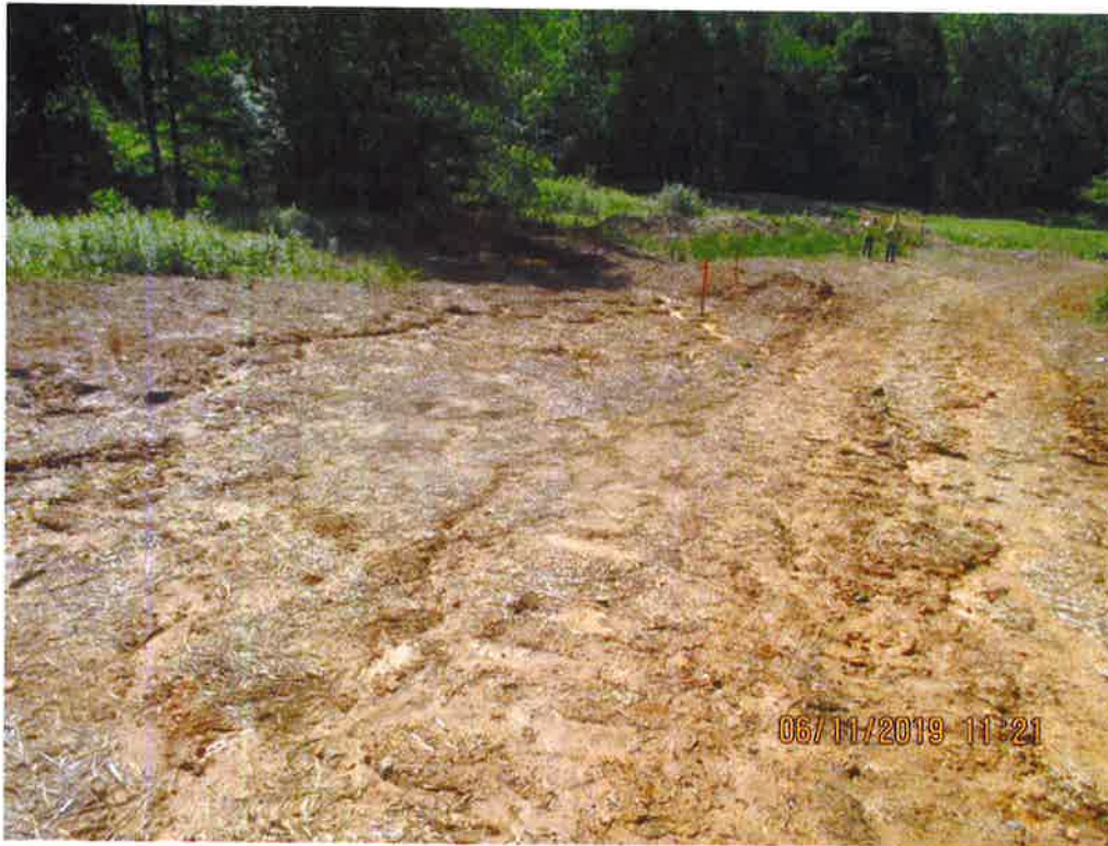
Facing South (Downslope) at station No. 7609+50. Waterbar receiving sediment due to erosion on slope.
