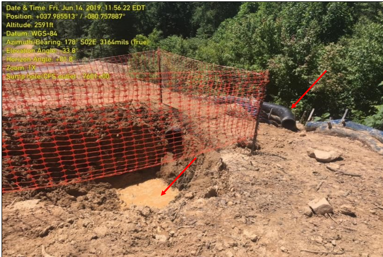
Photo 7: Photo illustrates the cleaned sump and additional CFS that has been installed near Station 7601+00.
