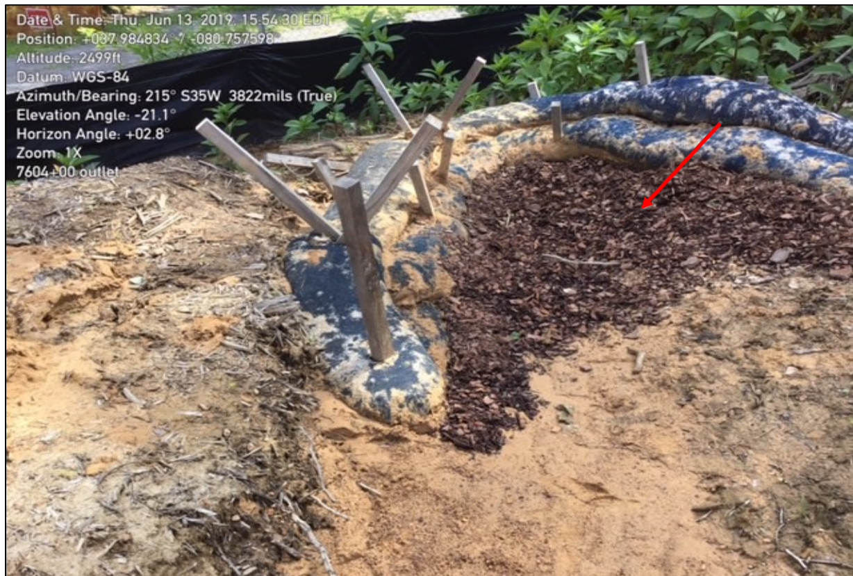
Photo 3: Photo illustrates additional filtration media that has been installed in front of existing CFS. This is upslope of Crosier Road.
