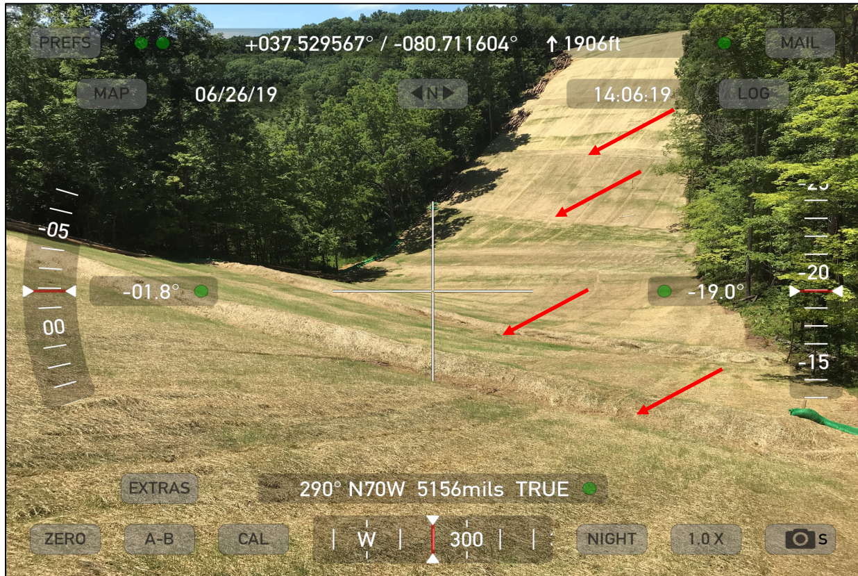
Photo 5: Photo illustrates the stabilization and permanent water bars that have been installed near Dargo Pond.
