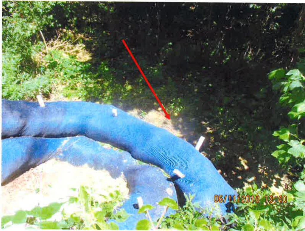
Controls below culvert outlet and bridge crossing with AR-182.5. Sediment deposits and SLW observed past these controls and LOD. Arrow depicts deposits.
