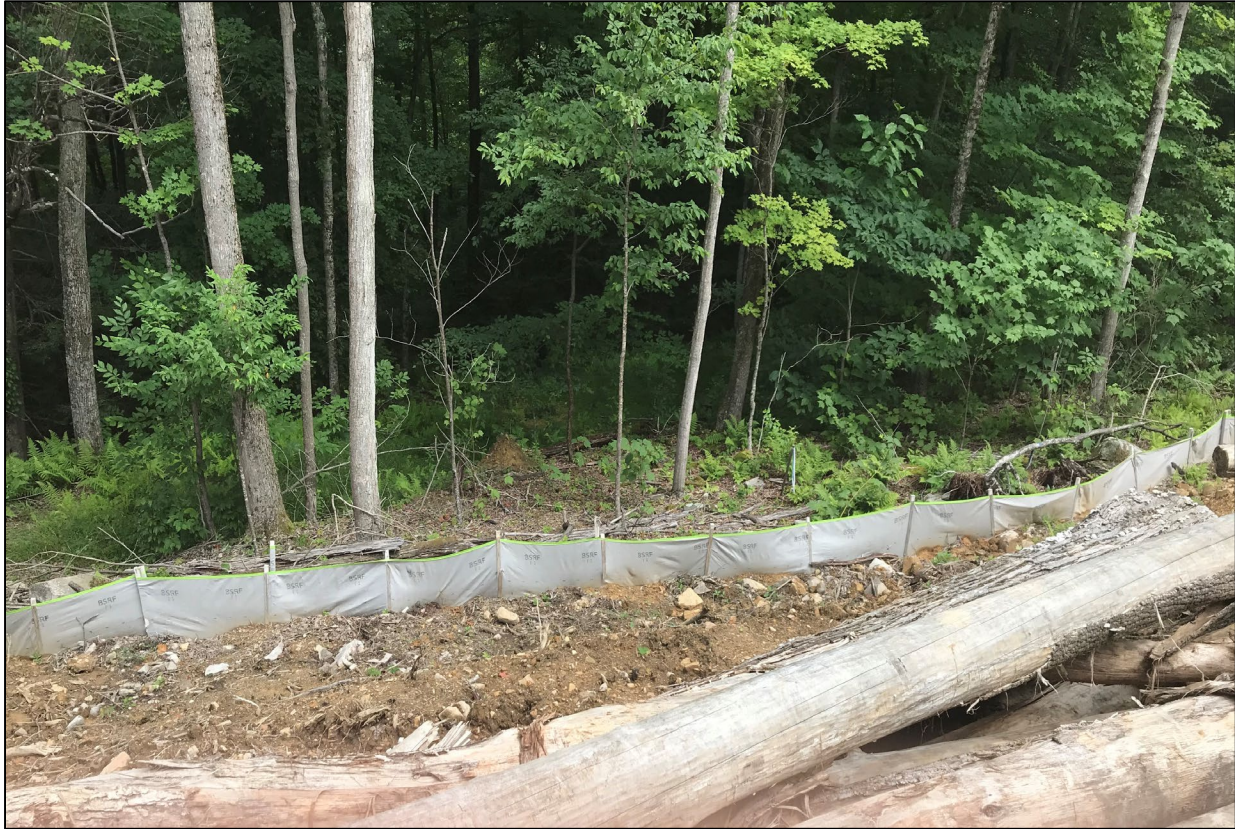
Photo 5: Photo illustrates the additional row of P1 silt fence that has been installed near Station 6497+50.
