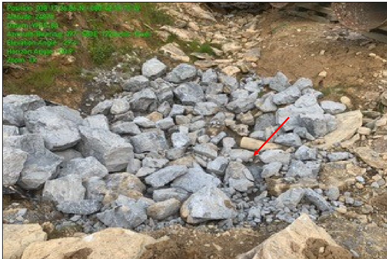
Photo 12: Photo shows the additional rock that has been added for stabilization near Station 6510+40.
