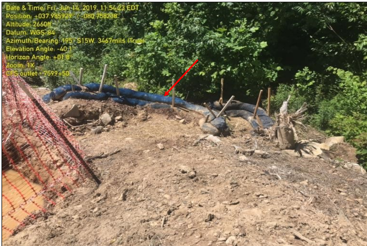
Photo 8: Photo illustrates the additional rows of ECDs that have been installed near Station 7599+50.
