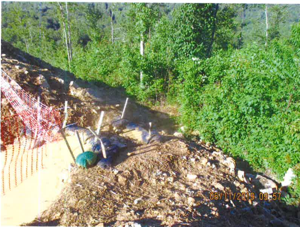
Station No. 7590. Waterbar outlet was overwhelmed with sediment and deposits were present past the LOD.
