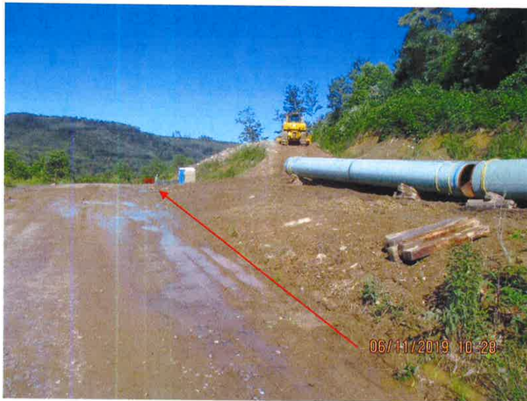
Standing on Krosier road facing east at additional workspace and ROW crossing. Mud and sediment present on road. Run-off flowing towards culvert inlet along Krosier road. Arrow depicts culvert inlet location.
