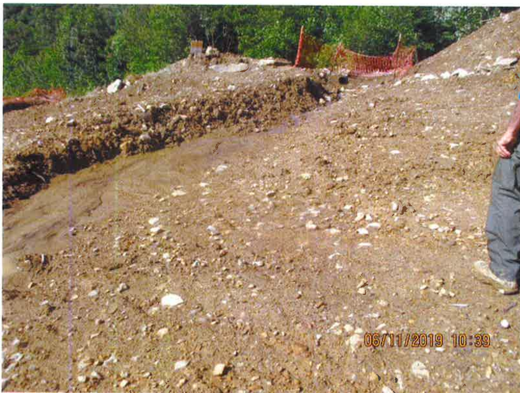
Below upper Krosier Road crossing near station no. 7576+01 facing towards Waterbar outlet. Erosion present on slope due to seep running onto ROW causing sediment to be deposited in Waterbar.
