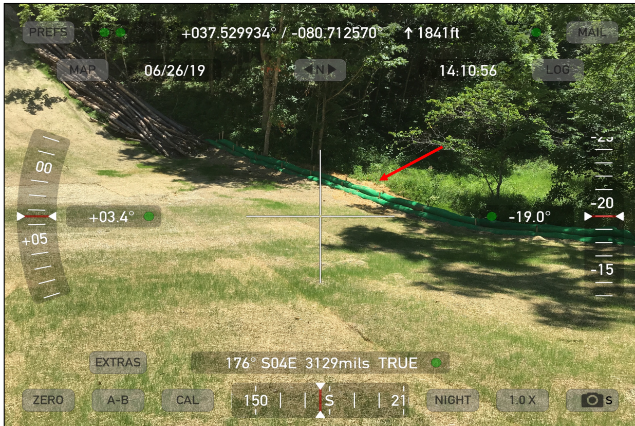
Photo 6: Photo illustrates the CFS and temporary stabilization that have been installed in the area upslope of Dargo Pond.
