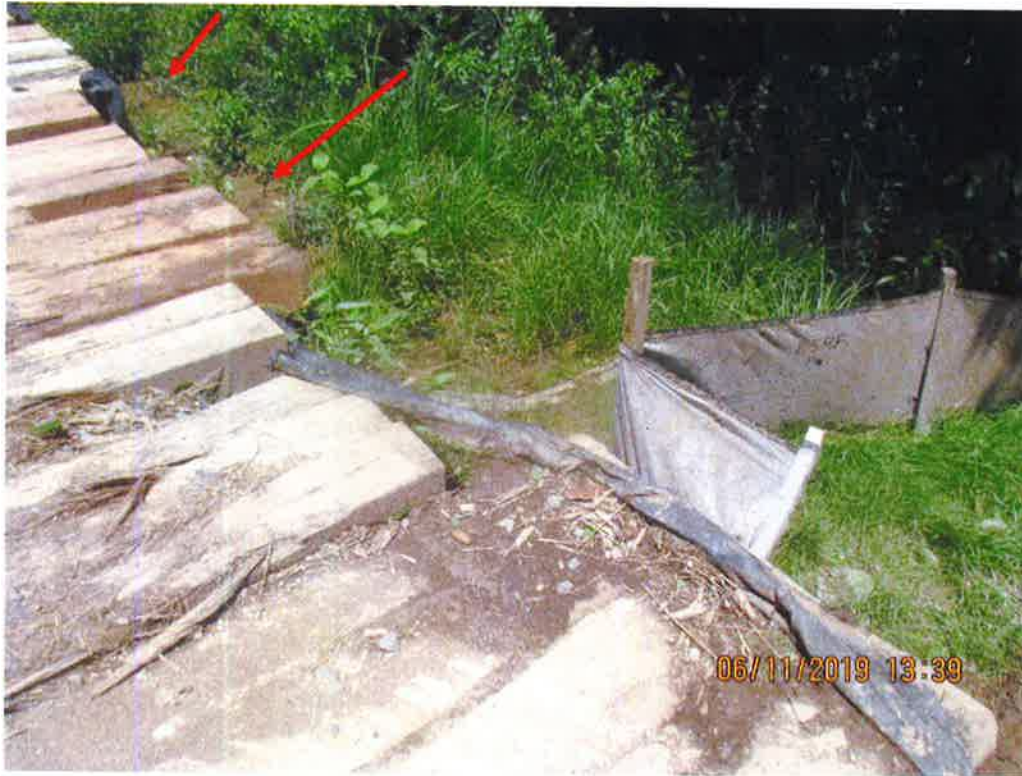
Wetland W-V2 crossing with AR-182.5. Sediment tracked onto bridge and has migrated past controls and into wetland. Arrow depicts deposits.
