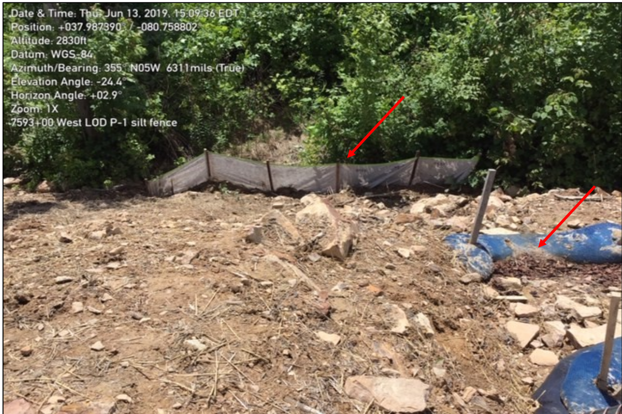
Photo 1: Photo illustrates the additional Priority 1 (P1) silt fence that have been installed and the filtration media has also been installed in front of existing compost filter sock (CFS).
