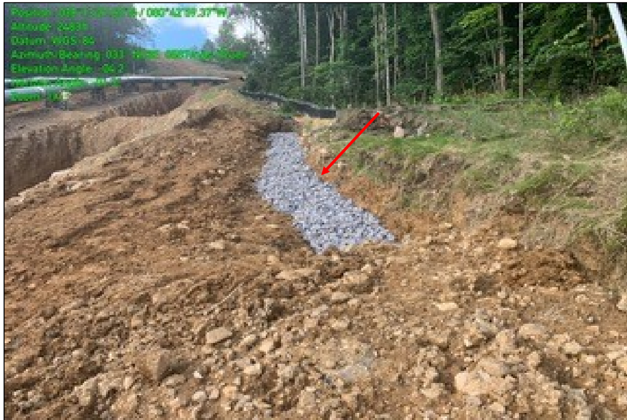
Photo 11: Photo illustrates the drainage channel installed near Station 6510+40.
