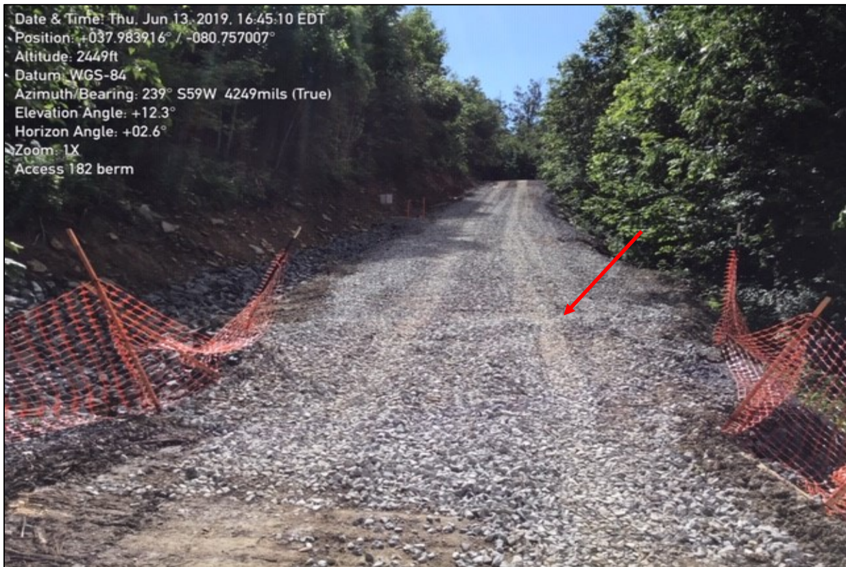
Photo 12: Photo illustrates the regraded broad-based dip in Access Road 192.
