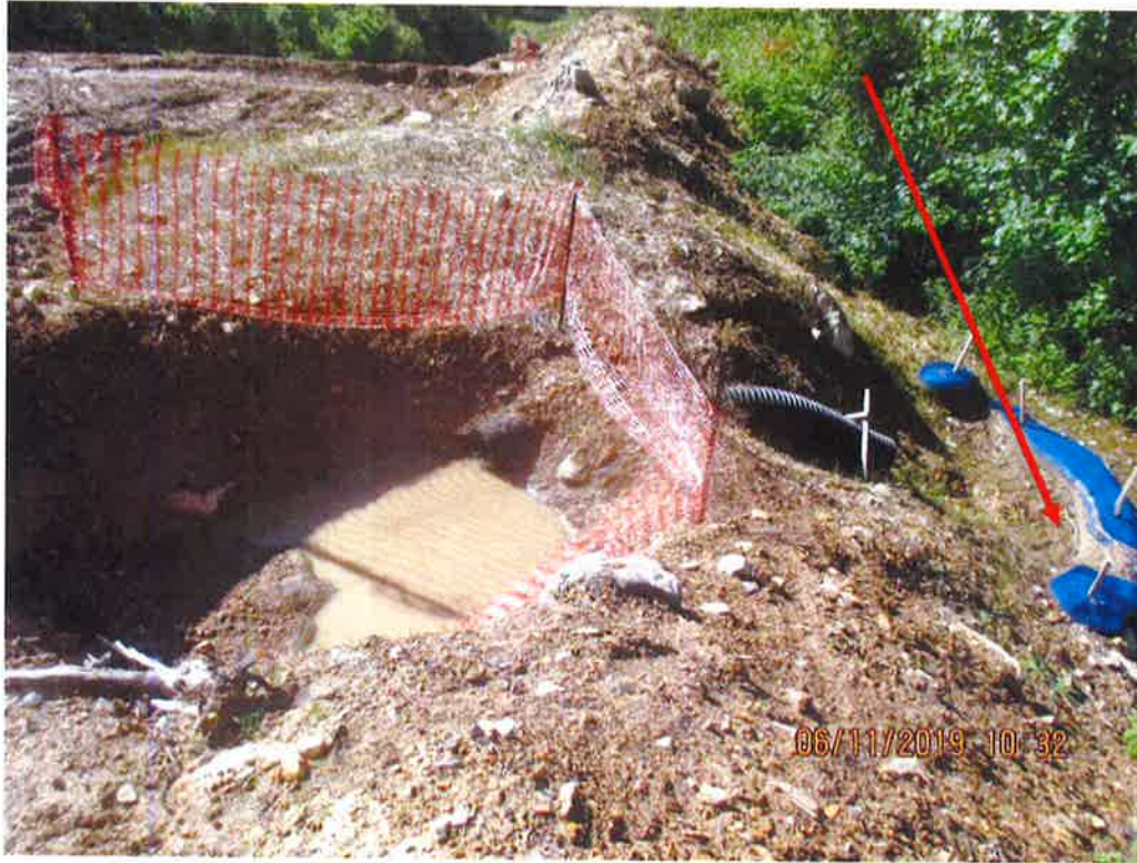
Downslope of Krosier Road Crossing near station No. 7576+01. Waterbar outlet perimeter controls in need of maintenance. Sediment laden water (SLW) and deposits were present past controls and LOD. Arrow depicts sediment backed up behind controls causing SLW to overtop the control.
