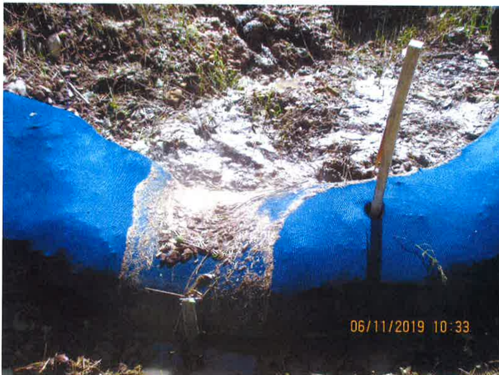
Perimeter control being overtopped with SLW and sediment backed up behind control.
