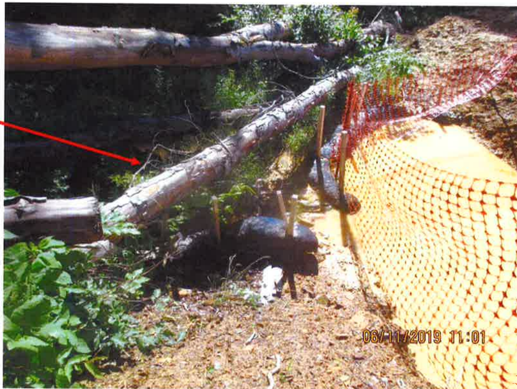
Above Lower Krosier Road crossing. Sediment and SLW overwhelming sump and perimeter controls near station no. 7604+41. Sediment deposits and SLW past controls and LOD.
