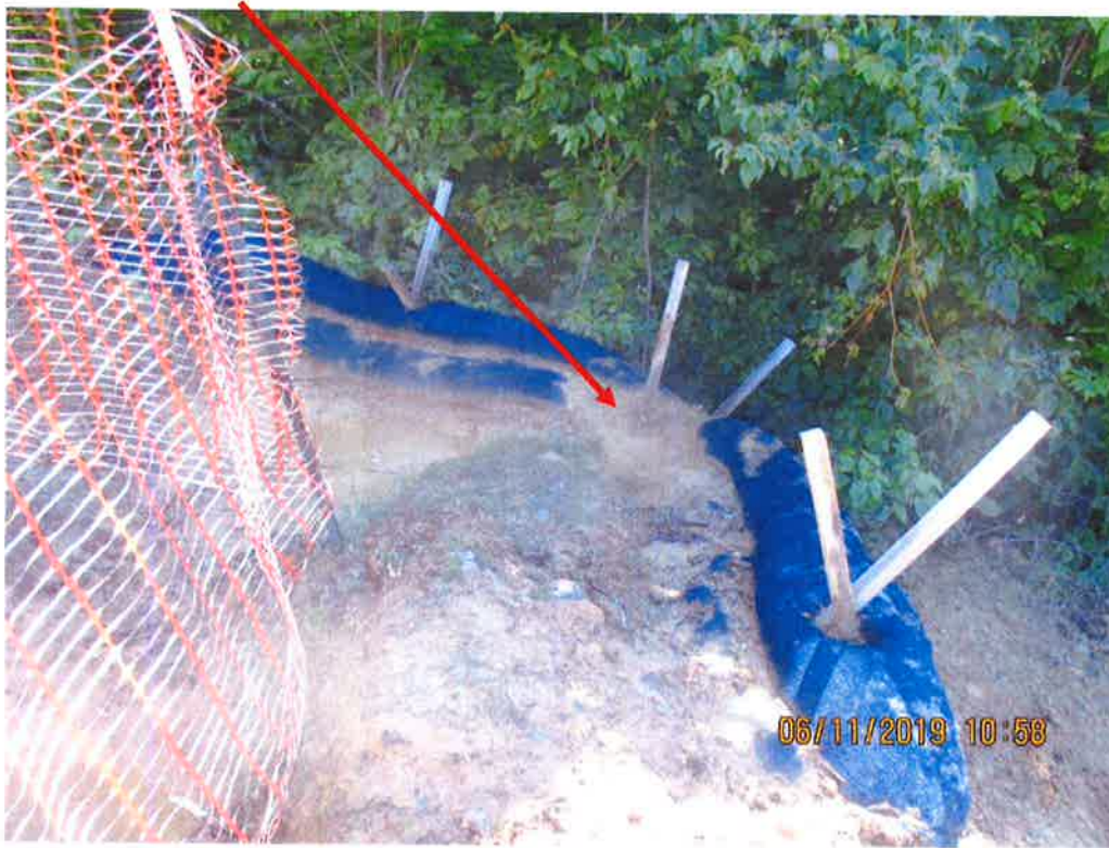
Above Lower Krosier Road crossing. Erosion present on ROW above Waterbar. Sediment being deposited in Waterbar and sump, overwhelming sump and perimeter controls near station no. 7604+41.
