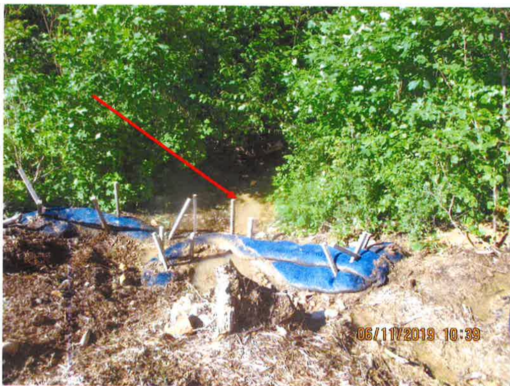
Standing at station No. 7576+01 downslope of Waterbar that had sediment being deposited in it due to run on from seep. Controls overwhelmed with sediment. Erosion on slope, SLW and deposits observed past LOD and controls.
