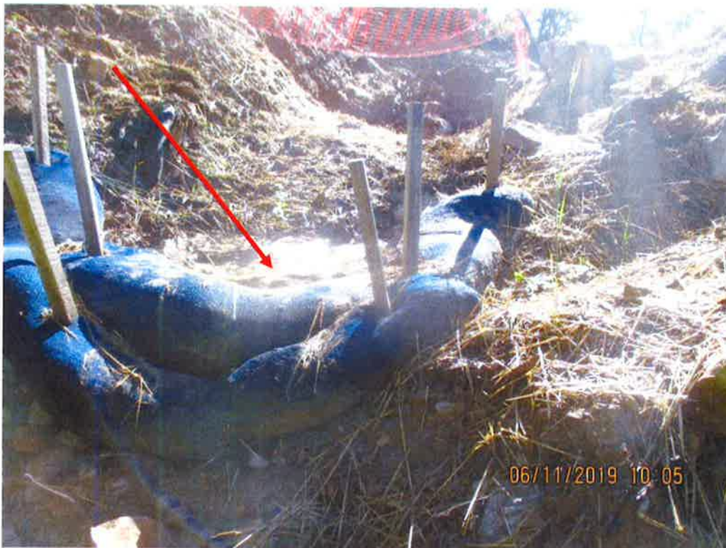
200-foot upslope of Krosier road crossing Waterbar outlet in need of maintenance. Controls overwhelmed with sediment. Deposits present past LOD.
