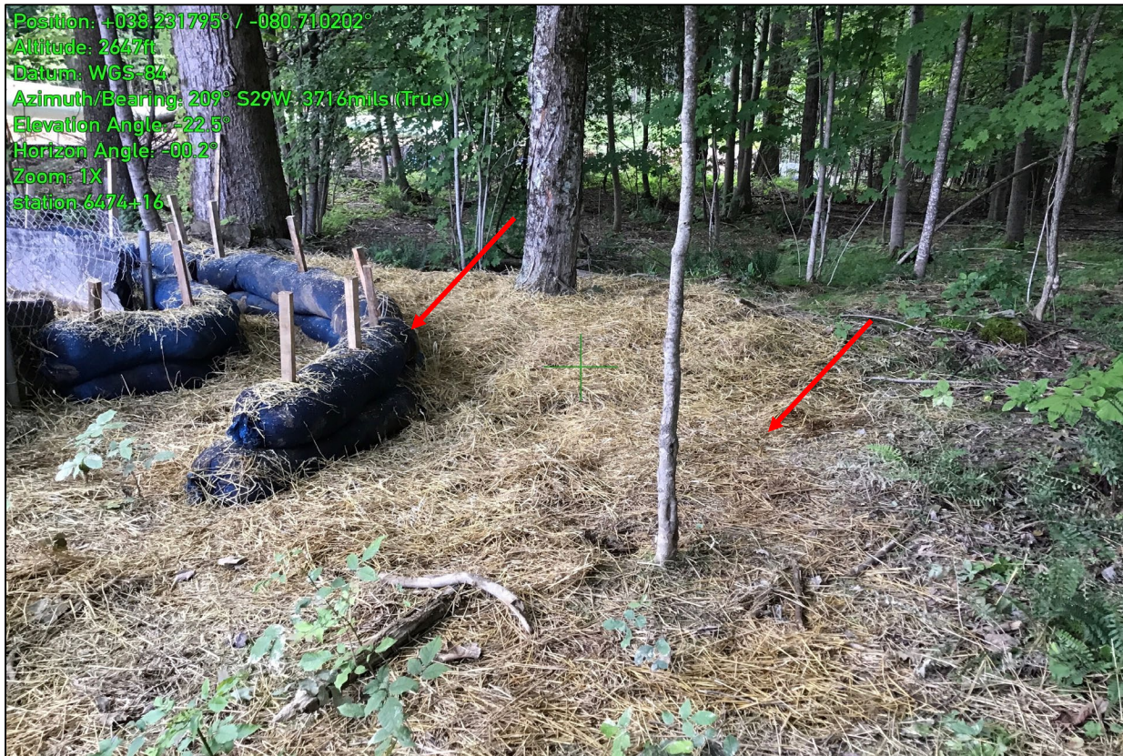
Photo 1: Photo illustrates the temporary stabilization and CFS that has been installed near Station 6474+16.
