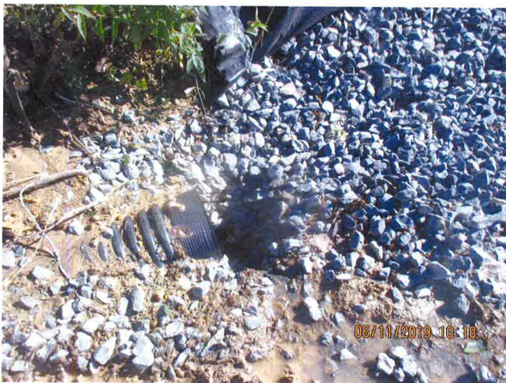
Culvert inlet with sediment present around the inlet at Krosier road ROW crossing. Downslope of Additional workspace and upslope of construction entrance and crossing.
