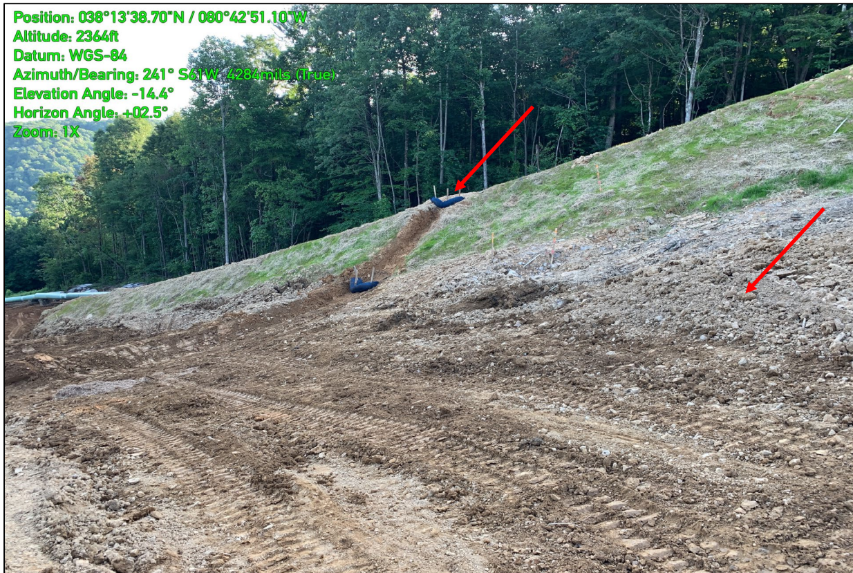
Photo 7: Photo illustrates the additional water bar that was installed near Station 6504+20 and the regraded LOD.
