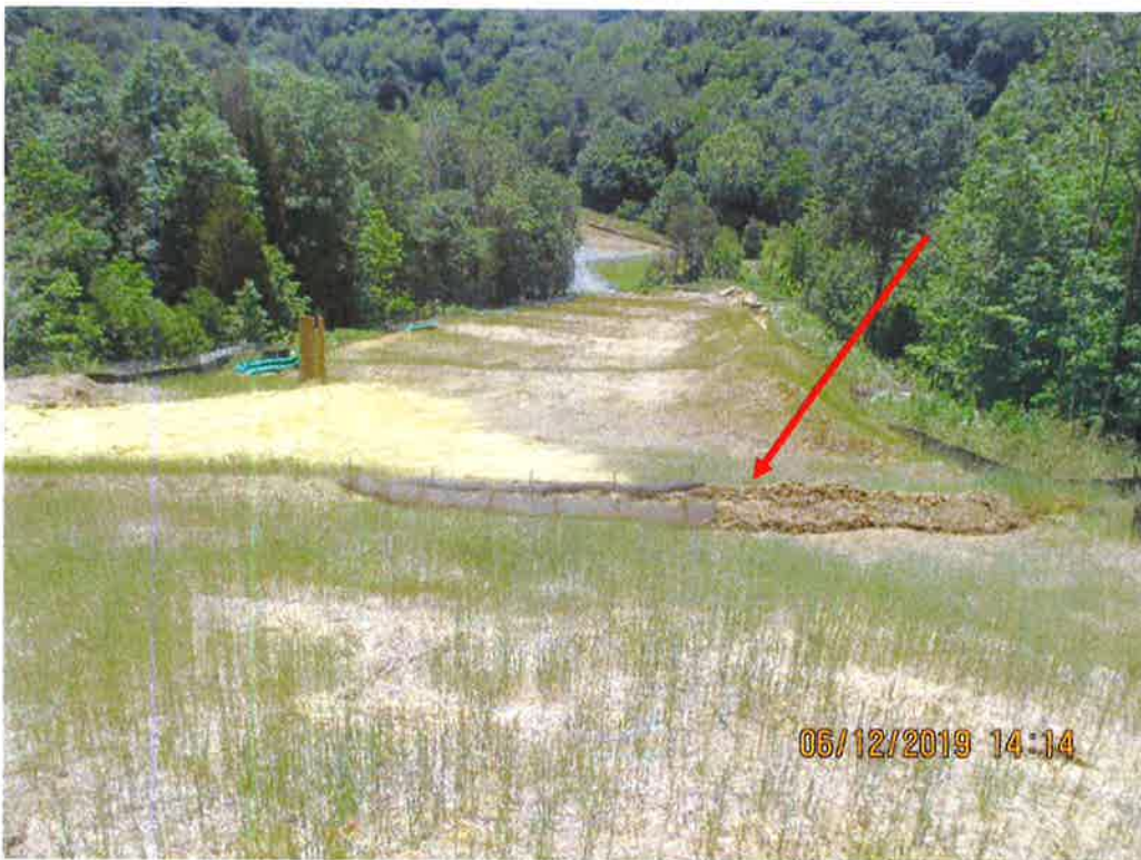
Facing South towards Ellison Ridge Road. Waterbar blow out and repair observed where AR-221 comes onto ROW.
