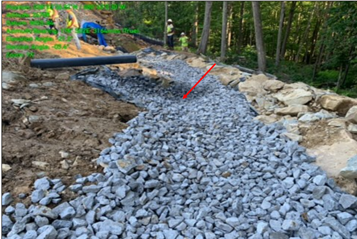
Photo 13: Photo illustrates the drainage channel installed near Station 6510+40.
