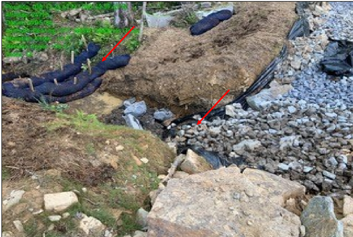
Photo 14: Photo shows the additional rock and CFS that have been installed near Station 6510+40.
