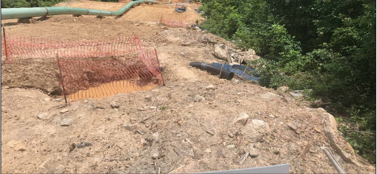
Photo 9: Photo illustrates the cleaned sump and regraded slope near Station 7576+01.
