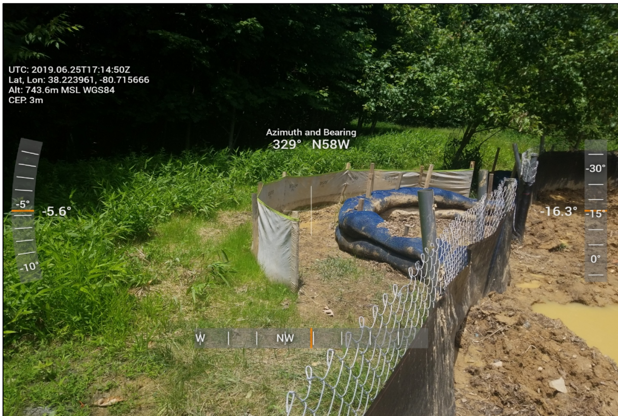
Photo 15: Photo illustrates the additional ECDs that have been installed along ATWS-22-7A., near Station 6514+60.
