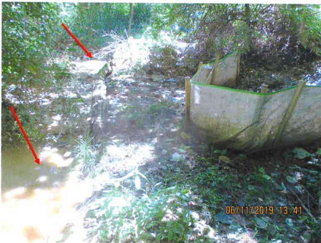
Further downslope of culvert outlet and standing below another culvert outlet where P1 silt fence was installed. Sediment deposits and SLW present. Arrows depict outlet controls and where SLW and deposits were observed.
