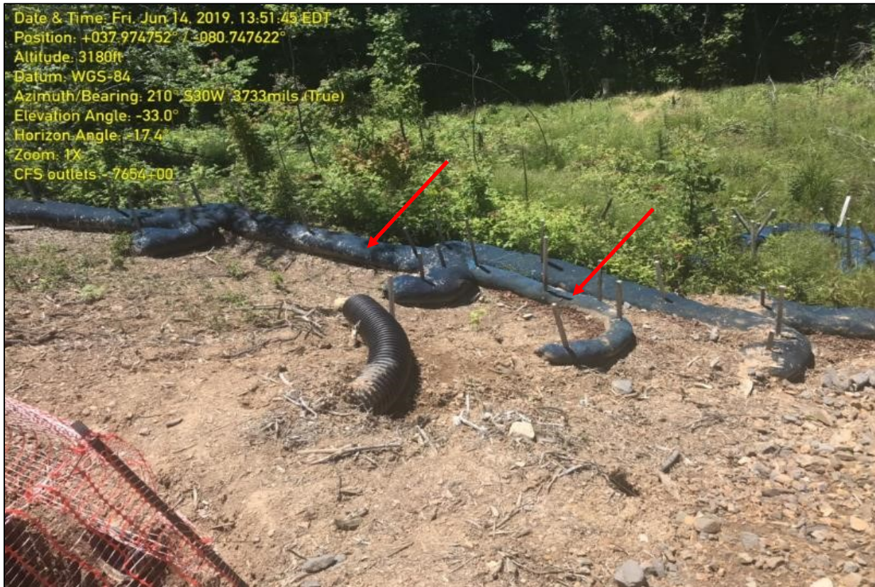
Photo 11: Photo illustrates the cleaned out area near Station 7656+00. The CFS has been replaced and the sediment has been pulled back onto the LOD. This area was identified as Station 7636+00 in the DEP report.
