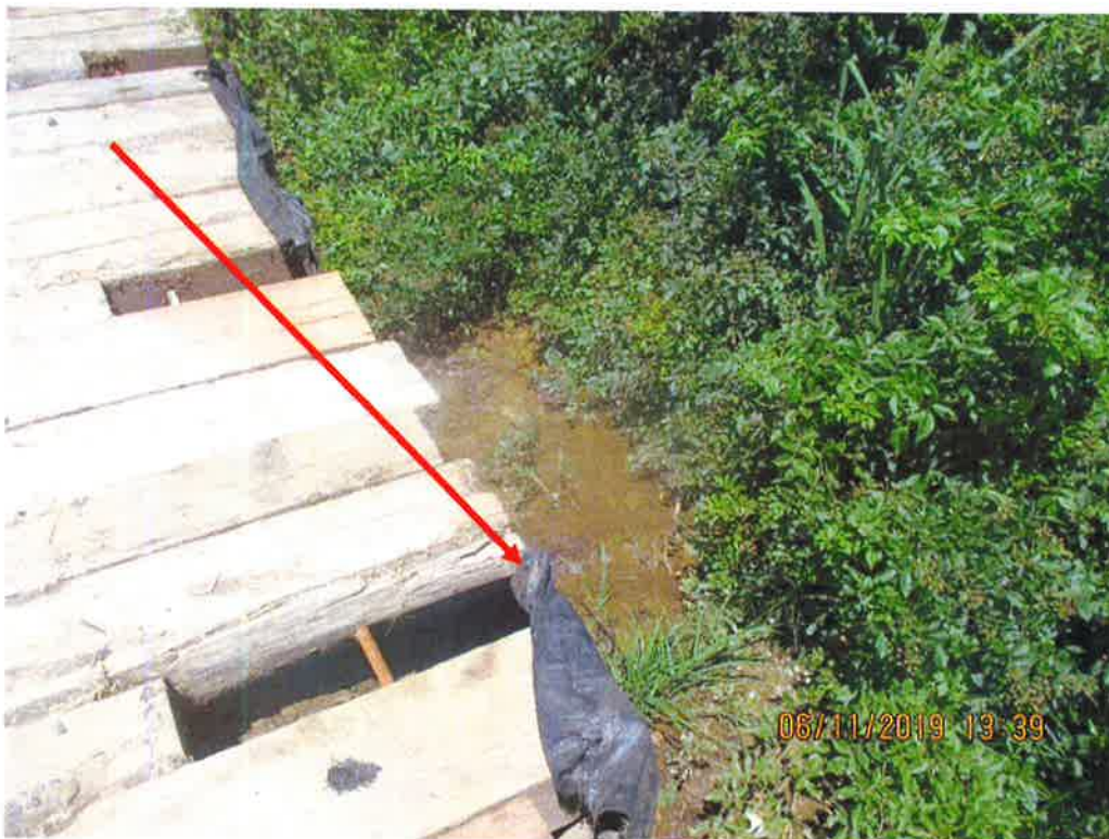
Wetland Crossing W-V6. Controls on bridge in need of maintenance. Impacts due to sediment migrating off bridge is an area of concern.
