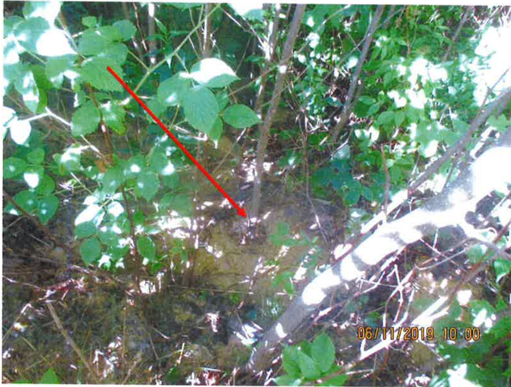
At station No. 7590 downslope of Waterbar outlet sediment deposits were present past the LOD.
