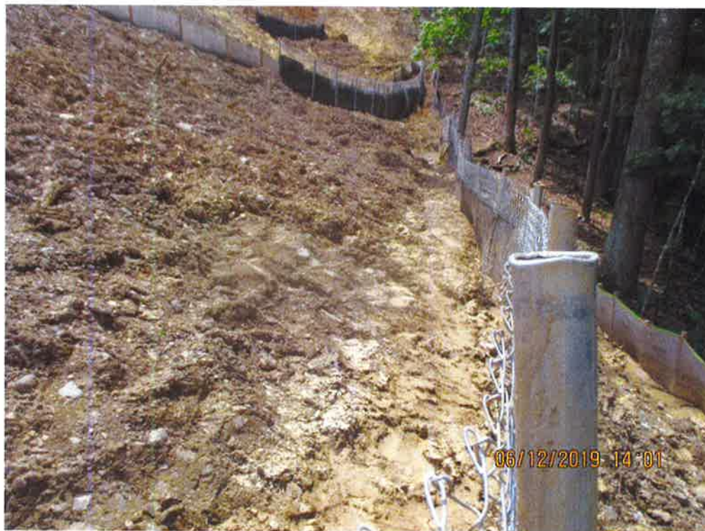
Controls below where dozer work was taking place. Sediment deposits observed below these controls at station No. 9780+00.
