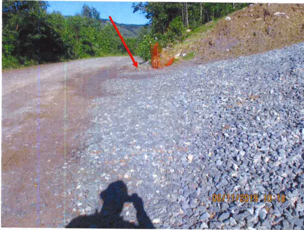
Upper Krosier Road Crossing facing West. Arrow depicts culvert outlets that flows downslope.
