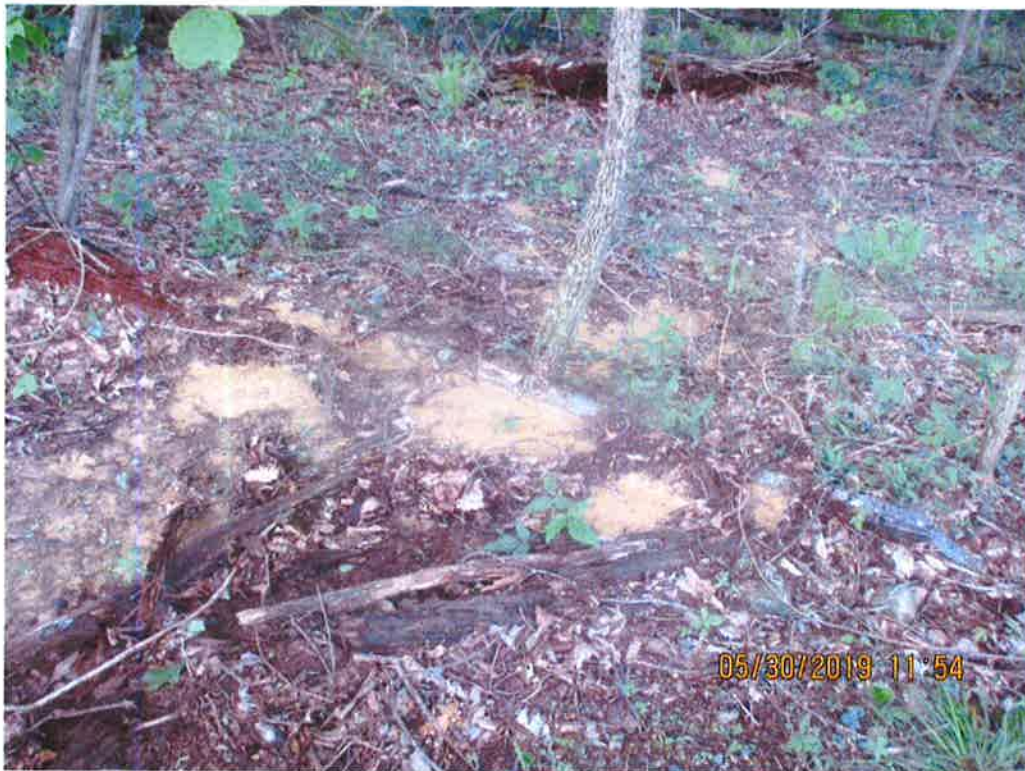
Sediment deposits observed past LOD and Controls below Waterbar and topsoil pile at station No. 6508+30.
