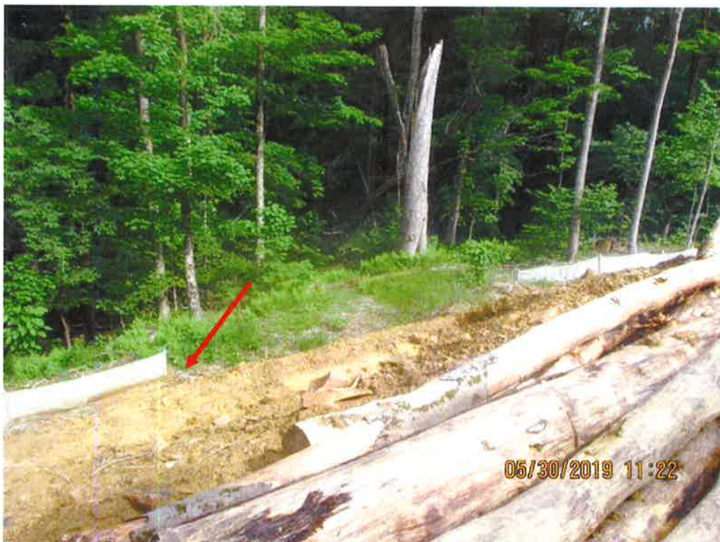
Station No. 6497+50. Perimeter controls not installed per SWPPP. Diversion berm installed however, arrow depicts section where sediment was being deposited against controls and not tied into berm.
