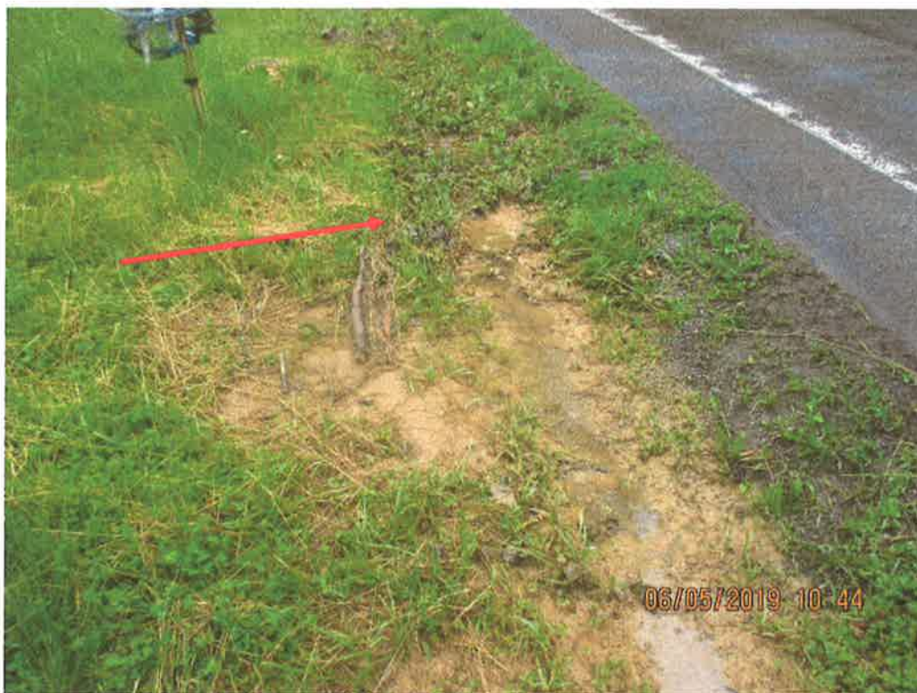
Sediment deposits in roadside ditch that parallels route 82. Arrow depicts culvert intake that conveys under route 82.
