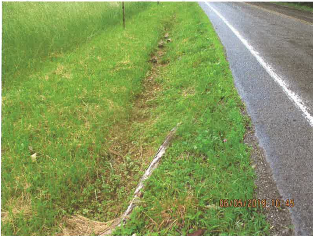
Upslope of culvert intake that conveys under route 82. No sediment deposits present at time of inspection.
