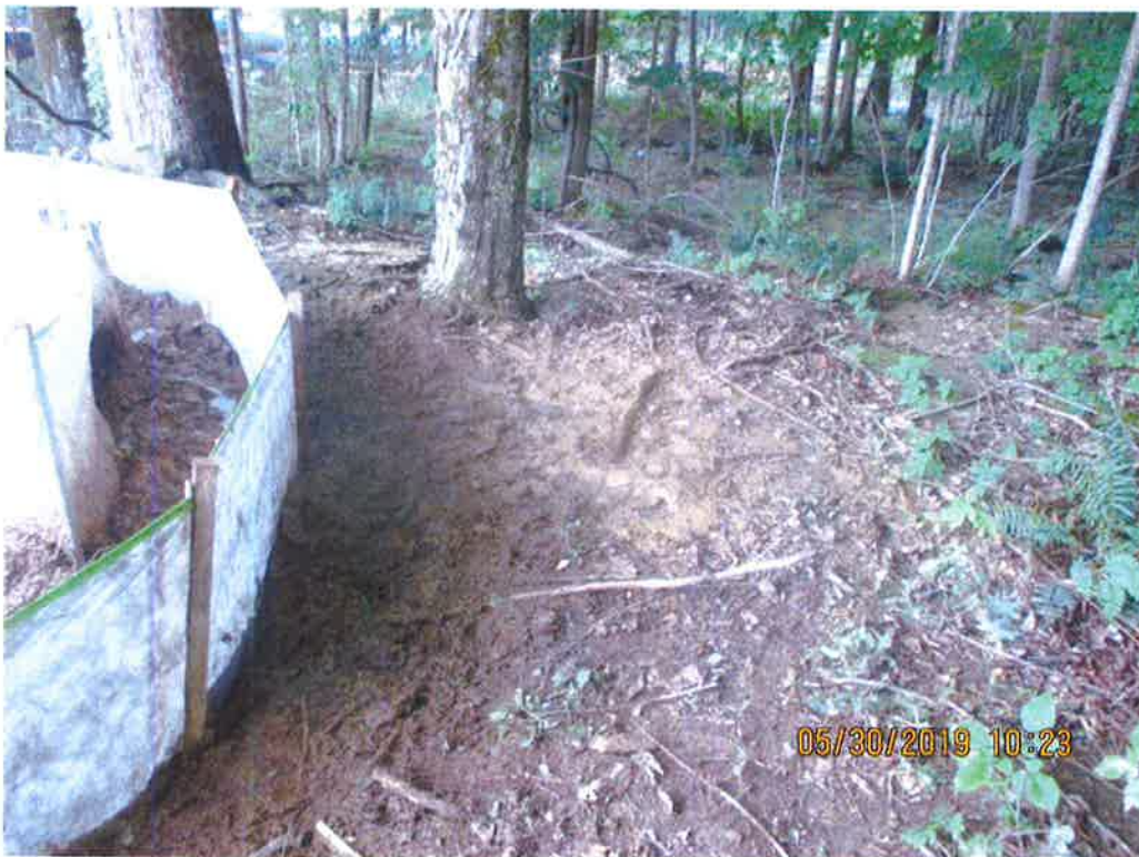
Facing downslope towards Stream S-N10. Scouring of vegetation and sediment deposits were observed below these controls.
