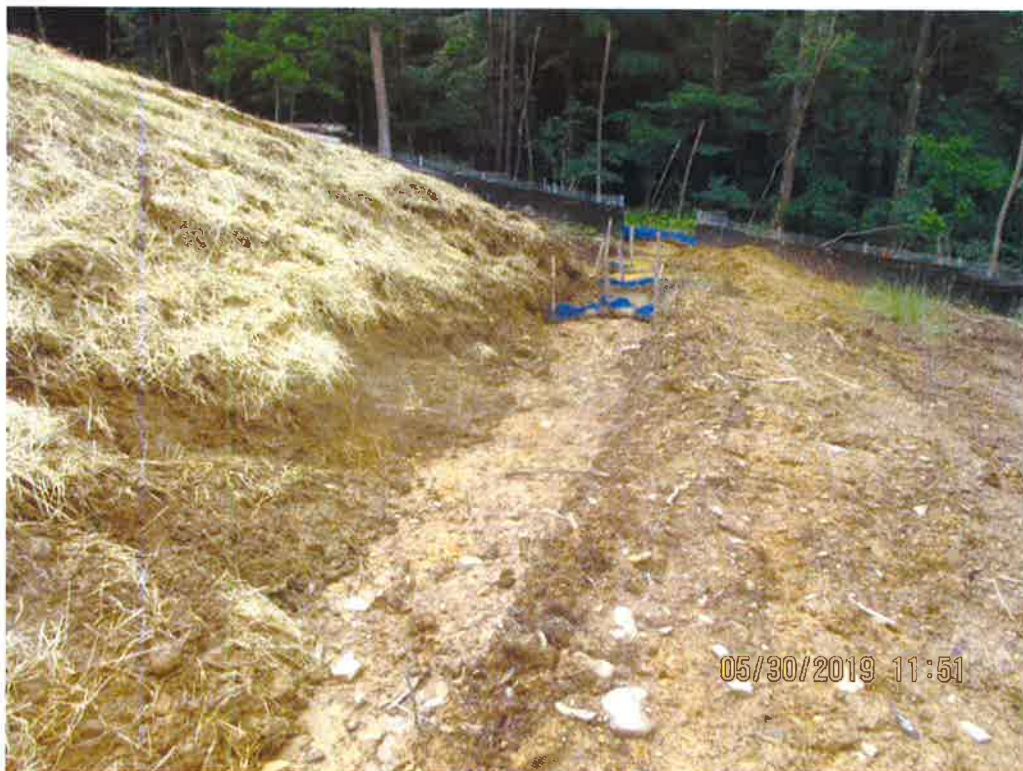
Waterbar with CFS checks installed and scouring topsoil pile below Deepwell road crossing at Station No. 6508+30.
