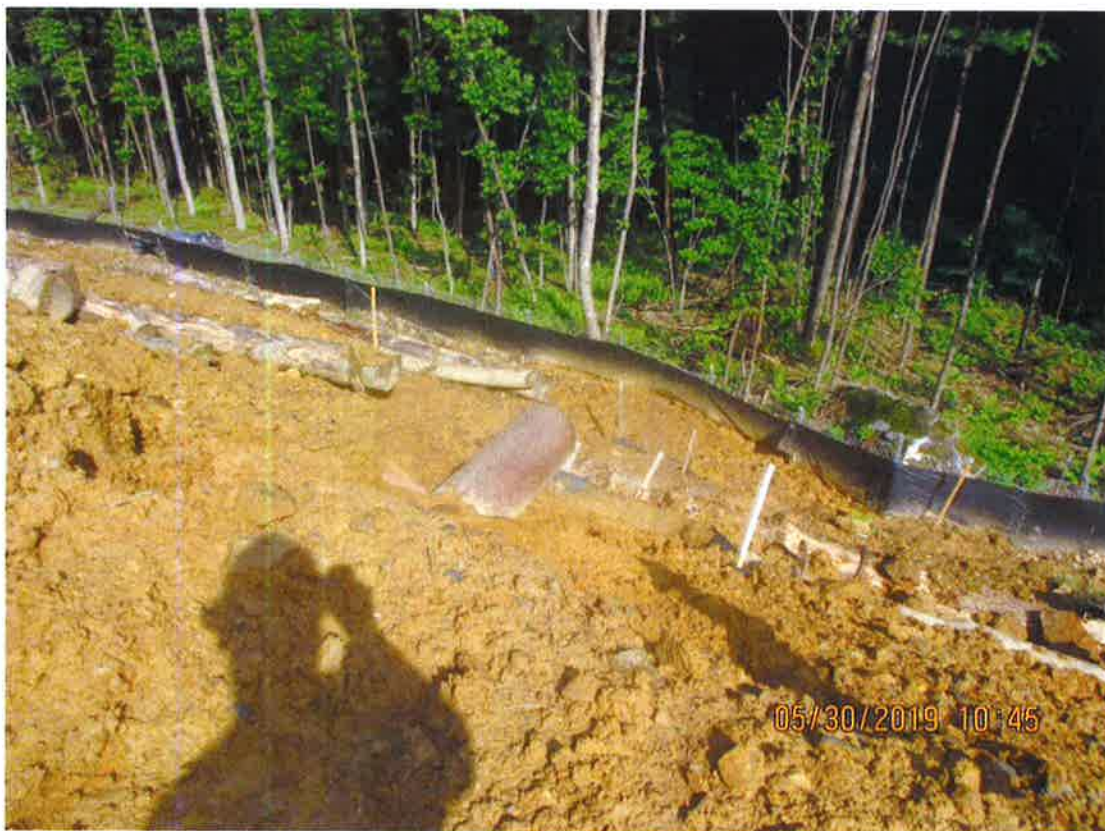
Pipe outlet below seep. Diversion not stabilized and No rip rap apron installed as required per SWPPP near station No. 6485+10. The inlet had been cut due to trench being dug.
