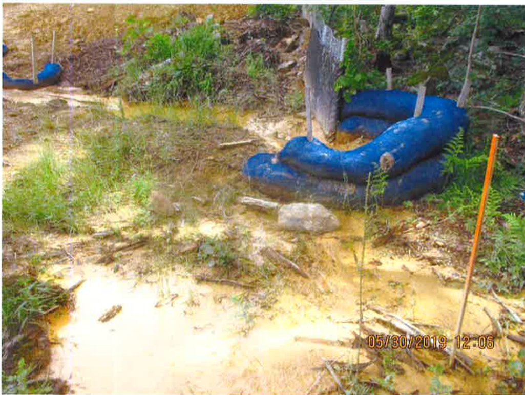
Waterbar outlet at station No. 6510+40 facing upslope. Sediment deposits were observed past LOD and conveying towards Wetland W-N18.
