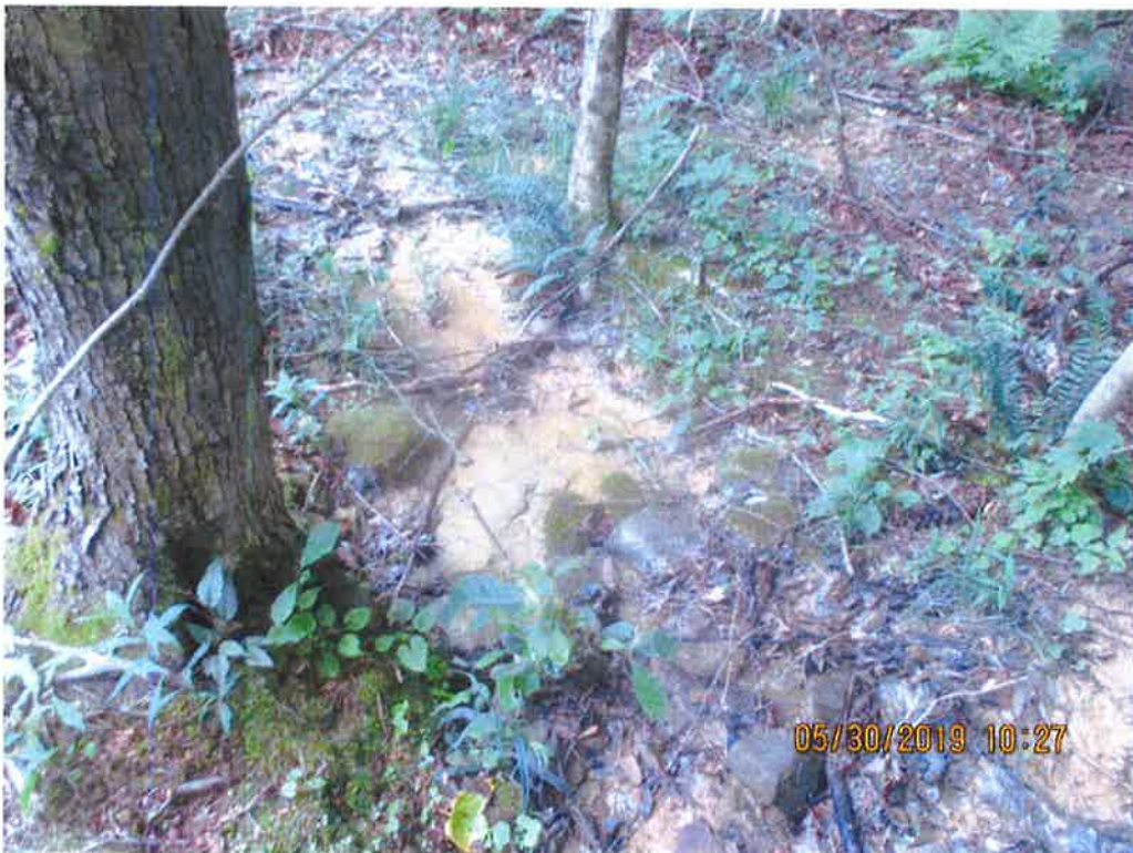
Sediment deposits past the LOD and controls at station No. 6474+16.
