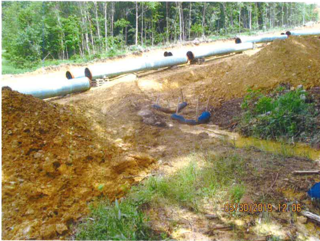
Waterbar at station No. 6510+40 facing upslope.
