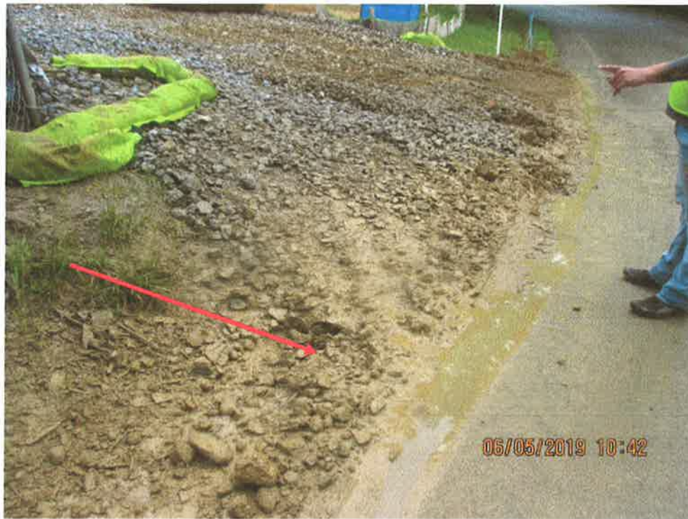
Construction entrance at the Route 82 crossing at station No. 5539+00. Arrow depicts culvert inlet.
