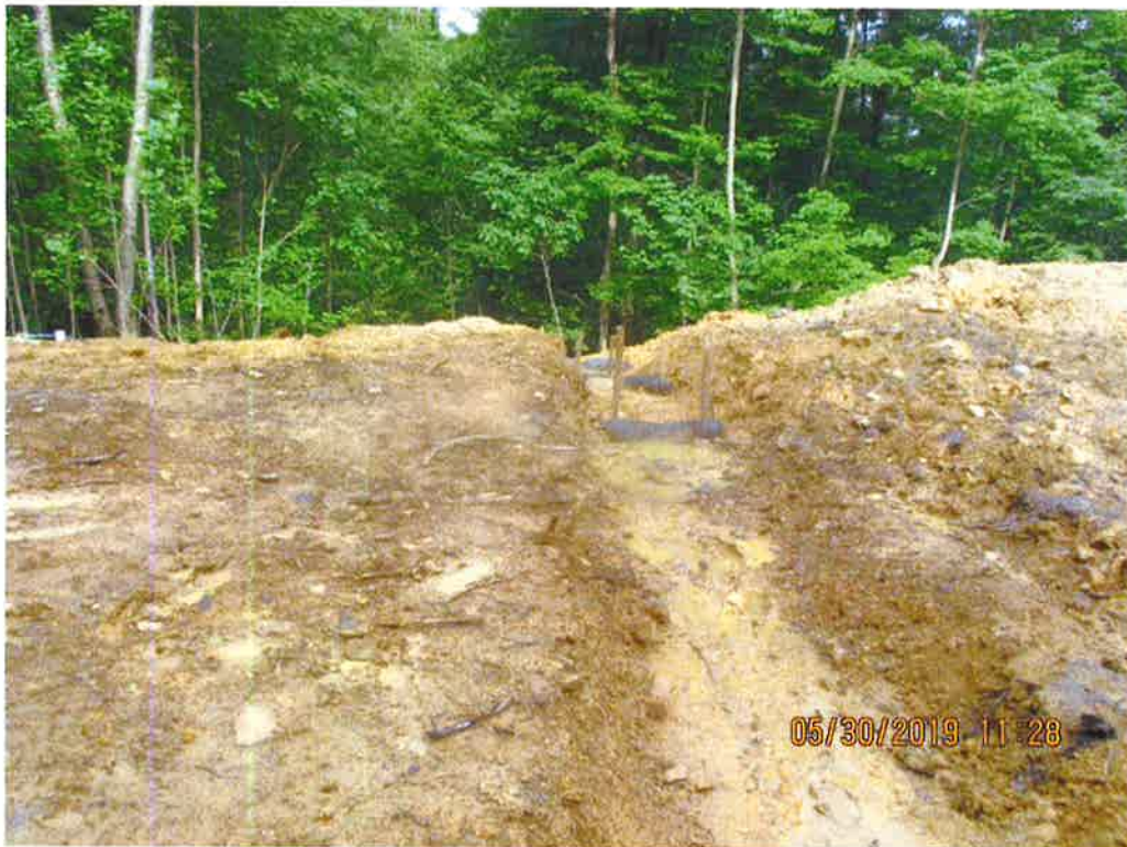
Seep running onto ROW via Waterbar above Stream S-N13. Diversion not stabilized near station No. 6940+00.
