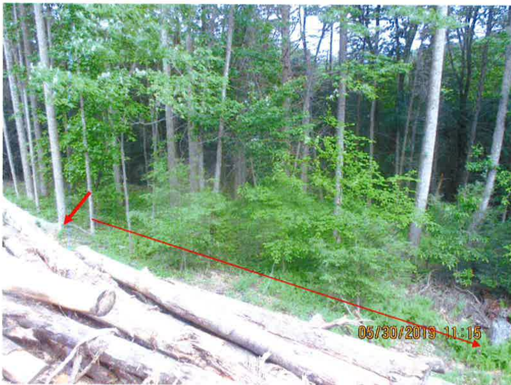
No perimeter control installed per SWPPP on downslope side of fill slope at station No. 6495+00.
