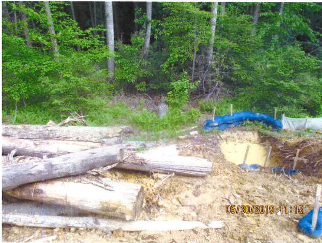
Same area near station No. 6495+00. Perimeter controls not extended per SWPPP into outlet controls.
