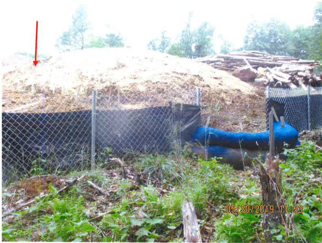
Facing upslope at Waterbar and topsoil pile at station No. 6508+30. Arrow depicts topsoil pile that is slipping into Waterbar.
