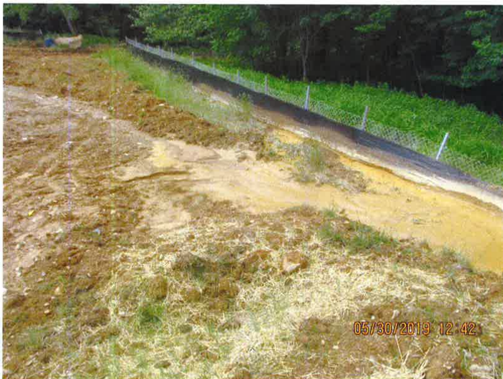
Erosion and sediment/SLW overwhelming perimeter controls at ATWS-22-7A at station No. 6514+60. Sediment deposits observed past controls and LOD.
