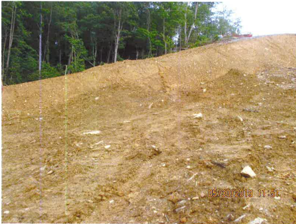
Facing upslope at Deepwell road construction entrance near station No. 6504+20. Erosion present on fill slope and ROW leading to Waterbar.
