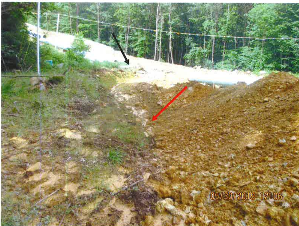
Sediment deposits and SLW traveling downslope at station No. 6510+40. Seep was present in cut next to topsoil pile. Channel wasn't stabilized and conveys to a sump with a slope drain that crosses ROW. Arrow depicts seep. Black arrow shows sump with slope drain inlet.
