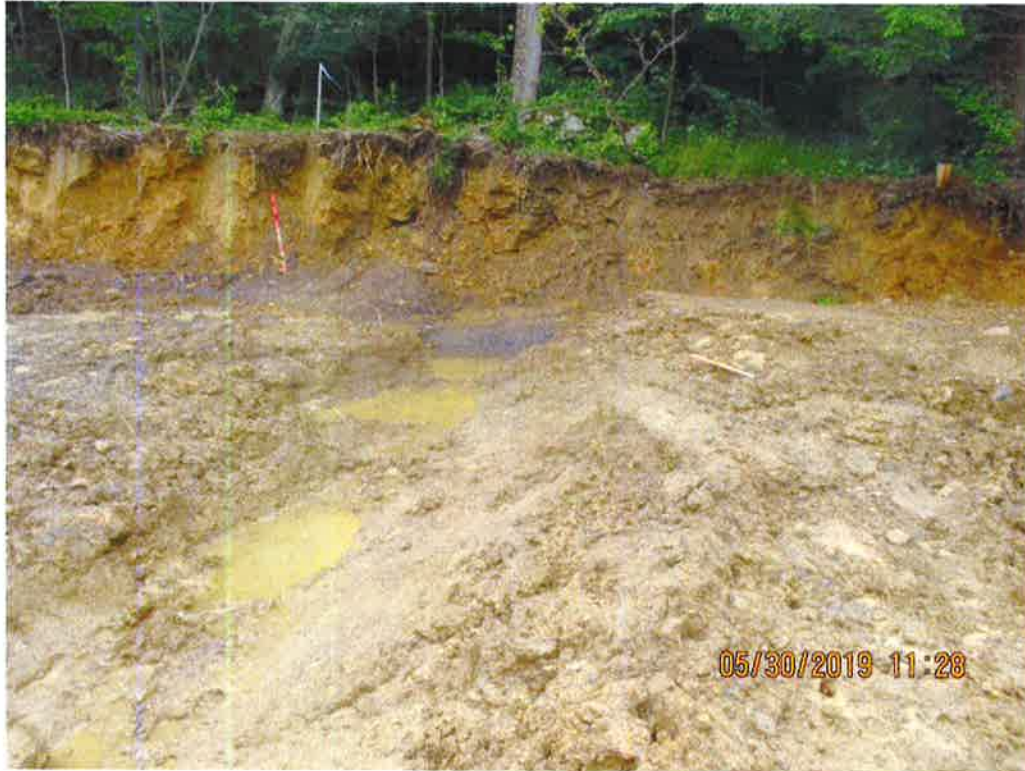
Seep running onto ROW above Stream S-N13. Diversion not stabilized near station No. 6940+00.
