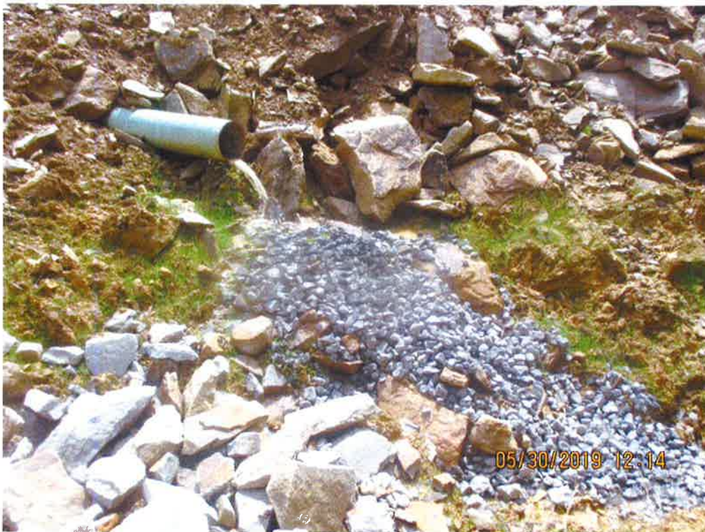
Seep slope drain outlet. Rock apron present.
