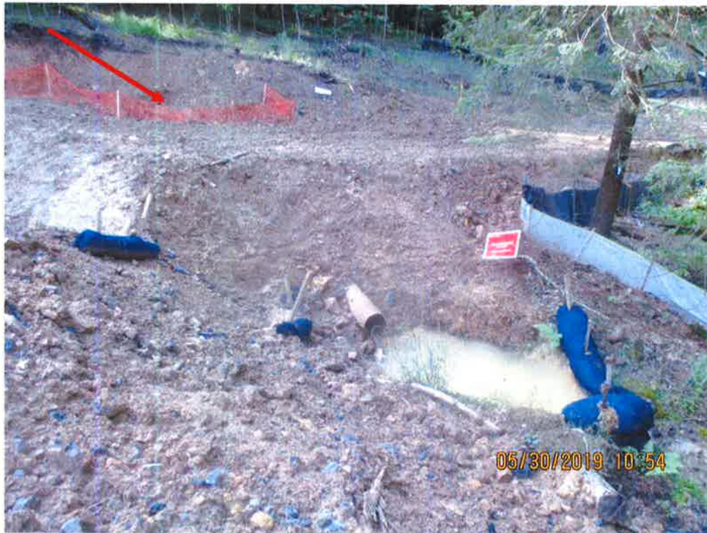
Sep drain outlet above Stream S-EE1. Clean water diversion not stabilized above or below inlet/outlet. Clean water was being conveyed approximately 15 foot across disturbed soil to a sump where the inlet was located. The topsoil pile around the inlet was eroding into the sump. Arrow depicts where inlet was located.
