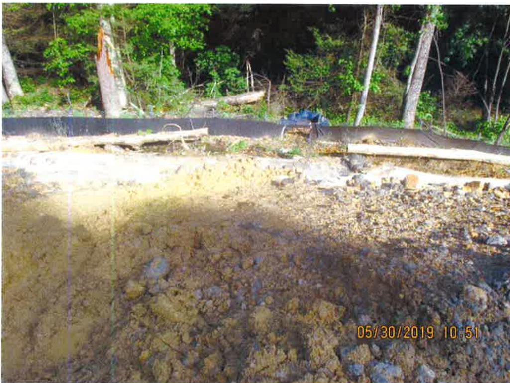
Waterbar outlet terminating onto slope at station No. 6485+10. Erosion present on slope above perimeter controls.
