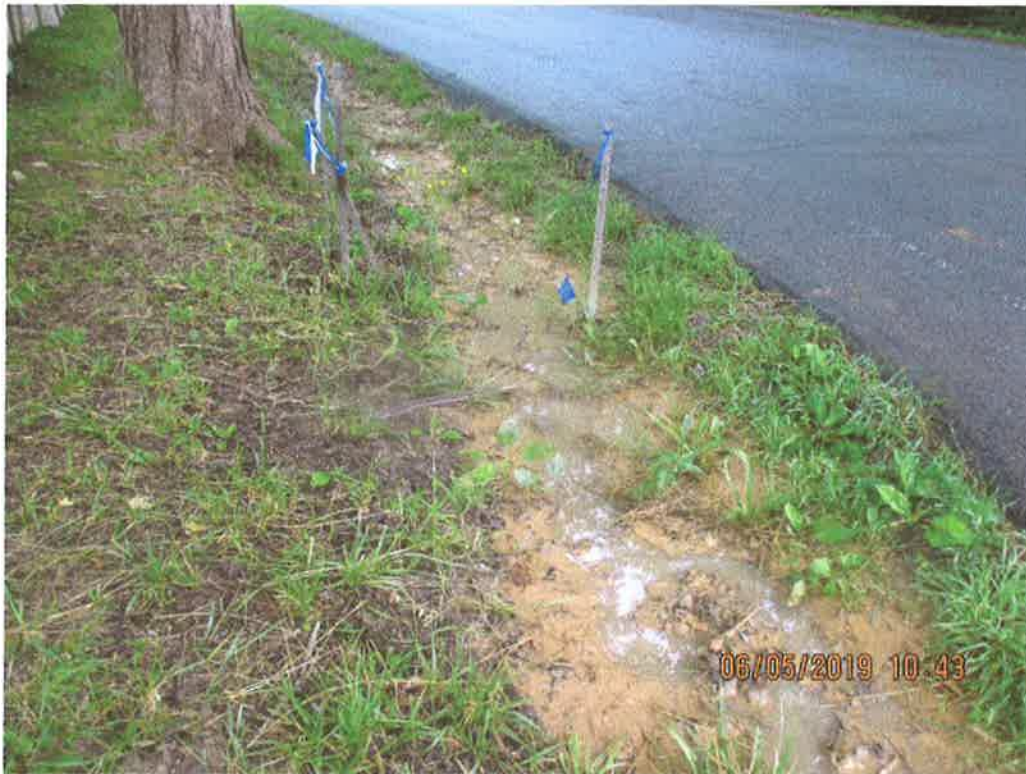
Sediment deposits and sediment laden water being conveyed past the LOD along Route 82.
