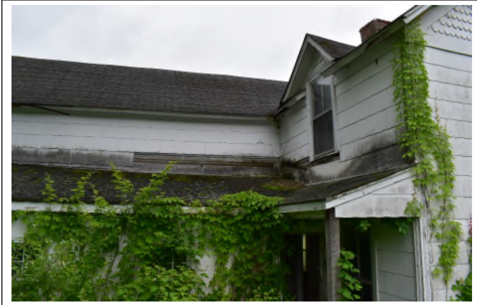
Photograph 5: Carter Residence – rear elevation (water-damaged walls and window sills, overgrowth, caving roof), View S
