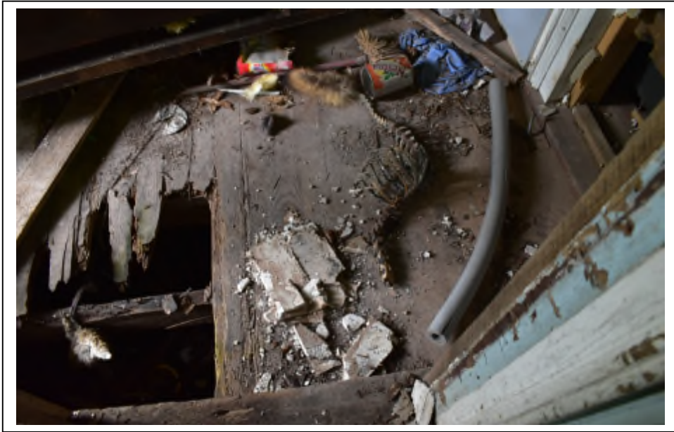
Photograph 7: Carter Residence – rear addition interior (missing floor boards, water-damaged, walls and flooring)
