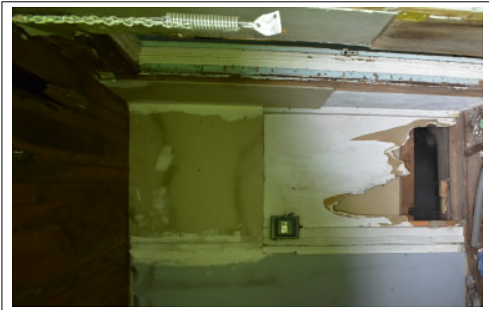
Photograph 9: Carter Residence -kitchen interior (water-damaged and missing ceiling, wall repairs that demonstrate previous damage and reconfigured rooms)
