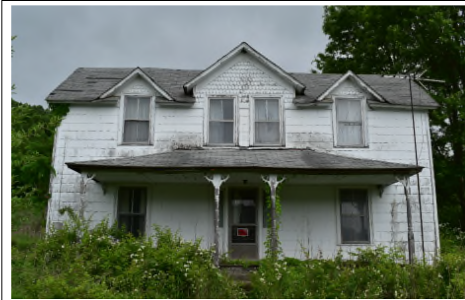
Photograph 3: Carter Residence – façade [overgrowth, roof damage, and water damage to exterior walls (most noticeably at porch roof)], View N
