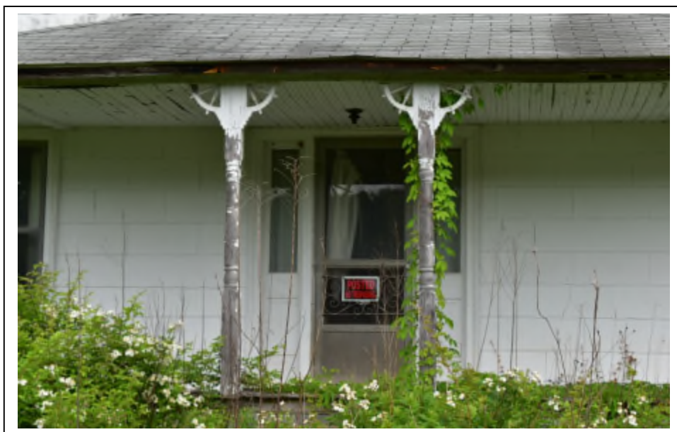
Photograph 2: Carter Residence - front porch (ceiling bowing and water damaged), View N
