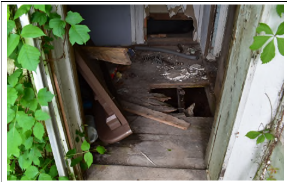
Photograph 6: Carter Residence – rear addition (missing floor boards, water-damaged floor and walls, overgrowth)
