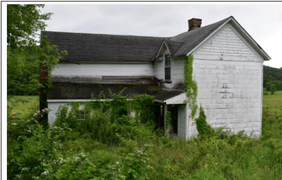
Photograph 4: Carter Residence – rear elevation (overgrowth, water damage to exterior walls, rear addition roof caving), View S
