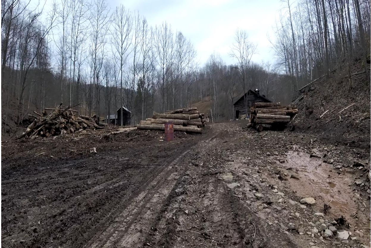
Photograph 1. Log landing area (proposed MVP-ATWS-1553) currently in use within the Cunningham Farmstead (Losch Farmstead BX-0351) for timbering operations unrelated to MVP undertaking. View Northeast.
