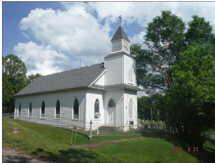
Photo 2-1. St. Bernard's Church and Cemetery (NR 85001583), Camden, Lewis County, Facing SW
